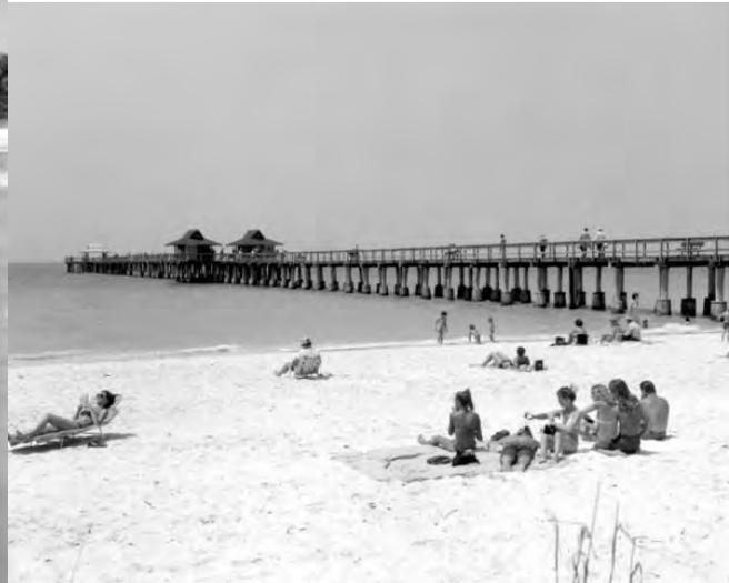
Figure 2, 3: Post-Hurricane Donna Design. Note the original concrete and wood trestle bents, which have since been replaced by all-concrete bents.
