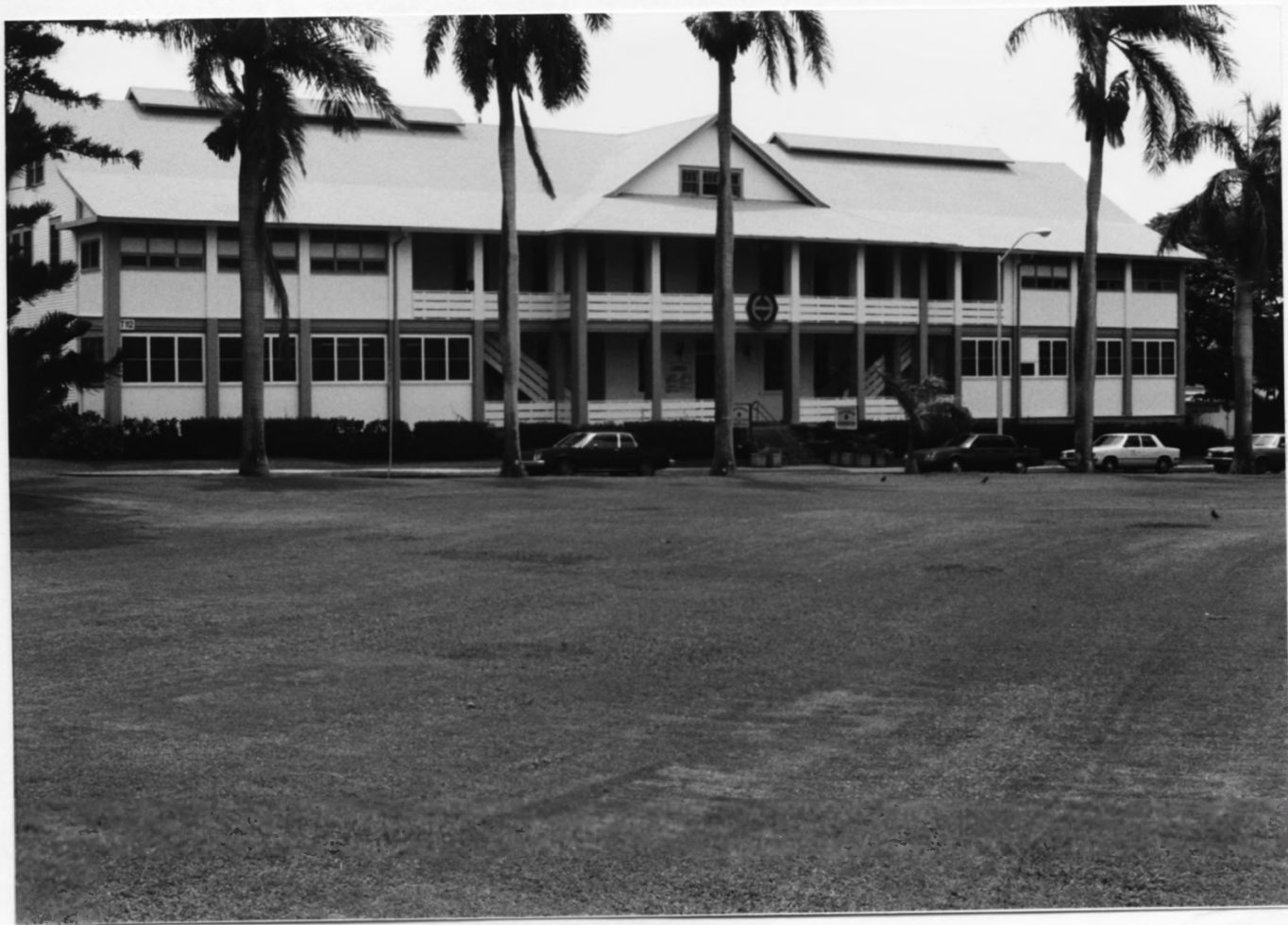
Typical 1907 barracks at Palm Circle, Fort Shafter, Hawaii. The building now contains administrative offices. The exterior corridors have been partly enclosed.
