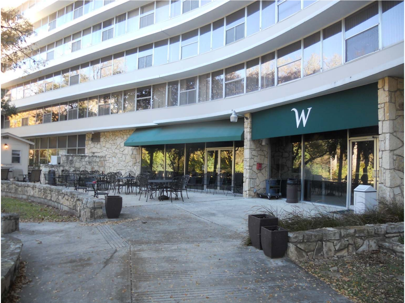
Photo 13 Patio access from first floor, facing north
