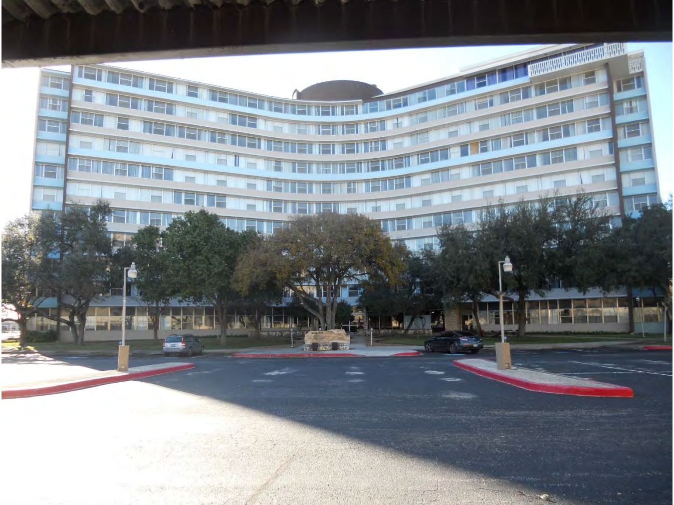
Photo 3 North elevation looking south
