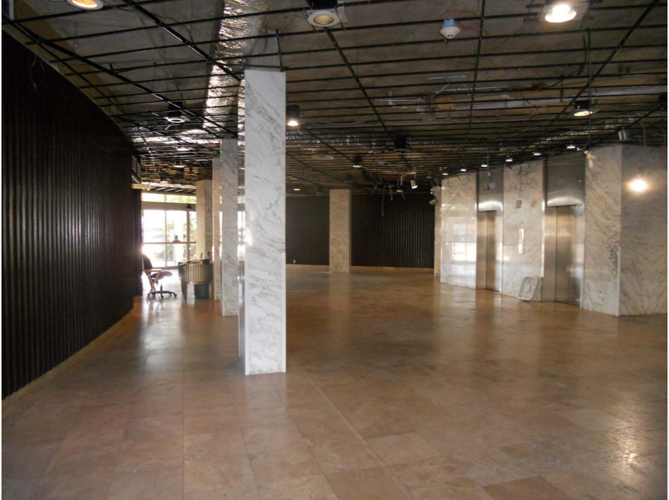
Photo 10 Lobby, facing southeast
