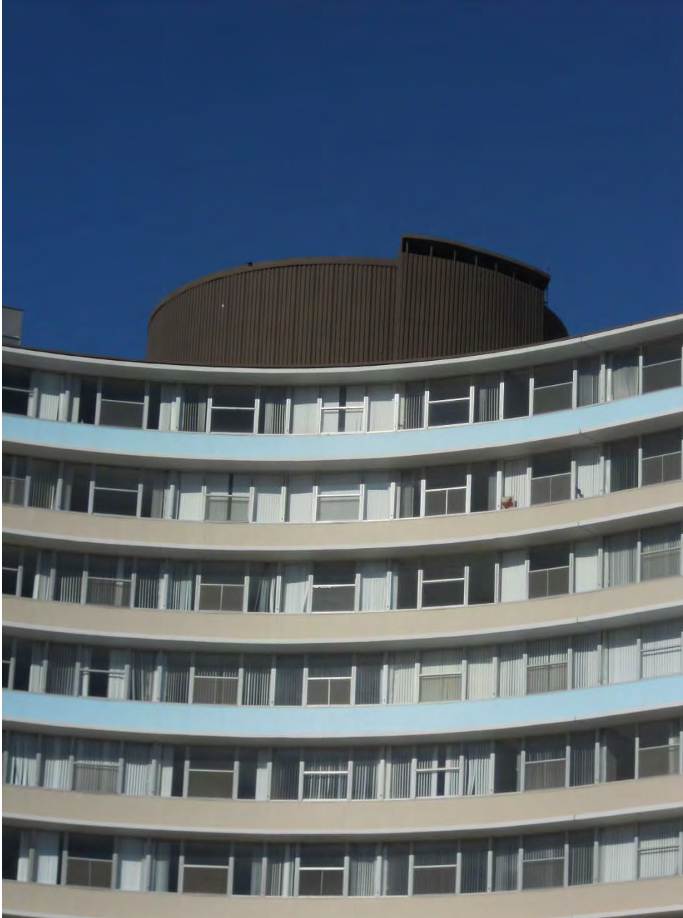
Photo 7 North Elevation detail, facing south
