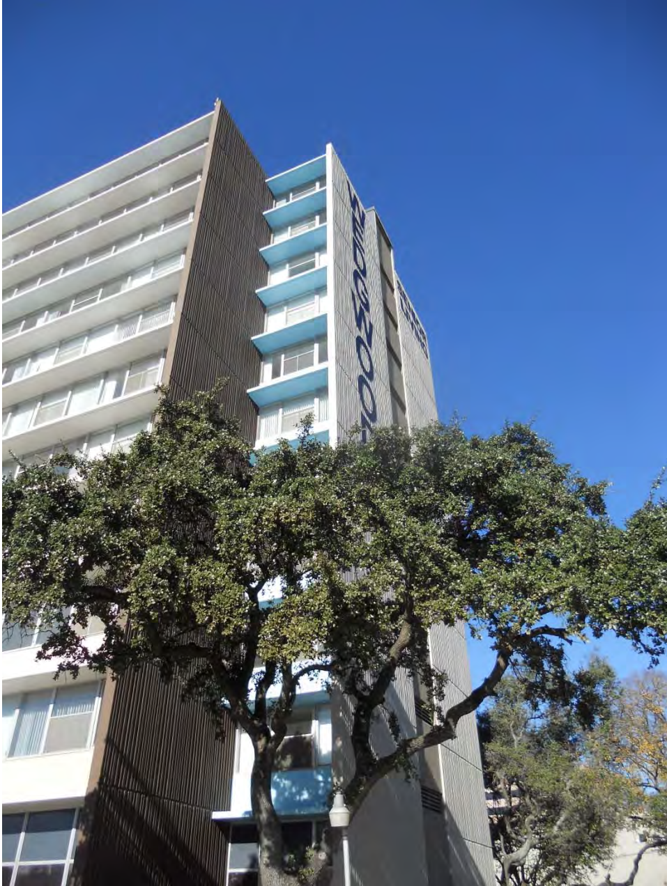
Photo 8 East wing fire stair setback, facing north
