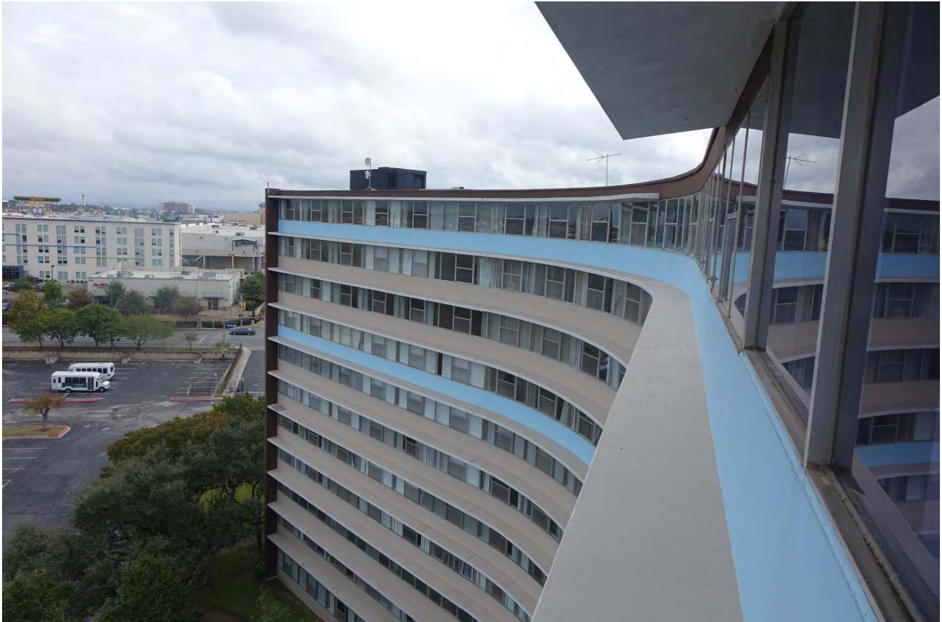
Photo 17 View from west end of the 11 th floor, looking east Photographed by Gregory Smith, October 2015
