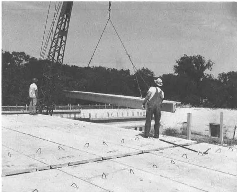
Figure 49. New concrete roof for 1907 packing cellar in 1958 (Siems collection).
