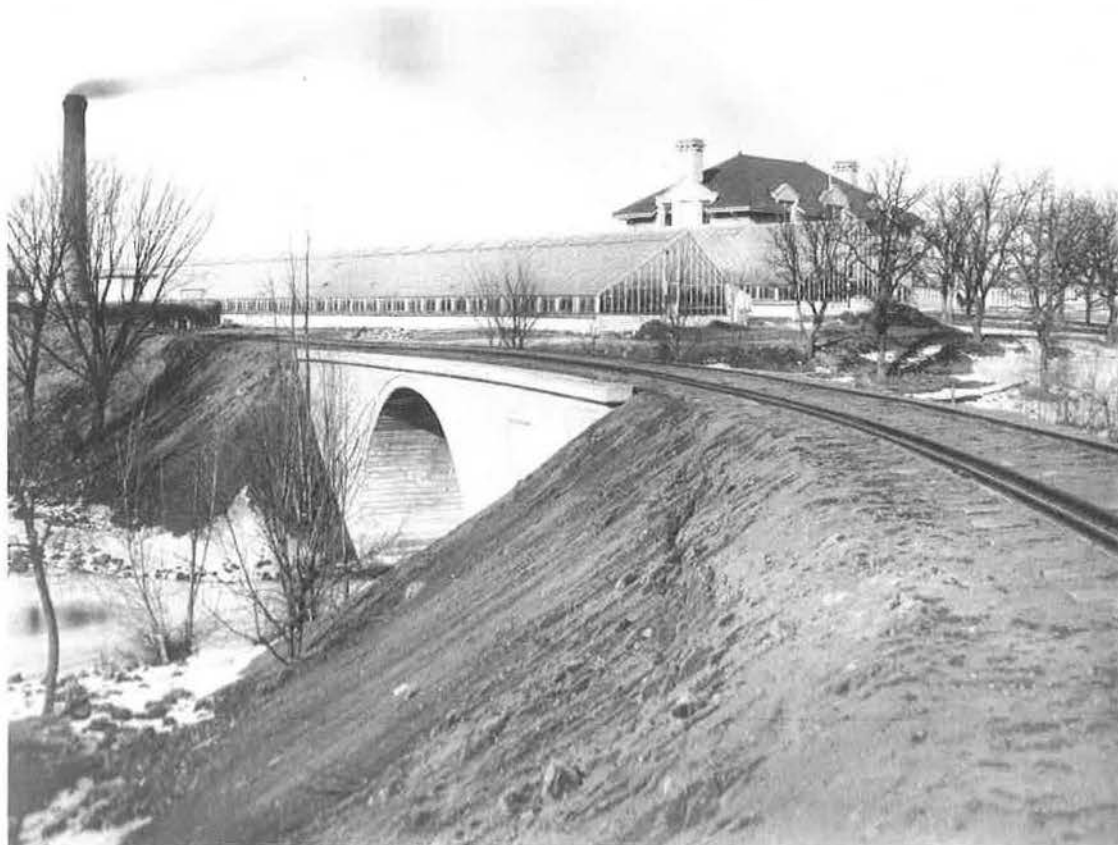
Figure 24. View looking west over south railroad bridge toward office, no date (Floyd County Historical Society).
