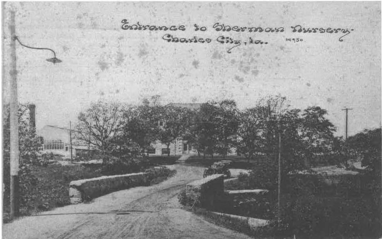
Figure 21. View looking west over stone entry bridge to office, 1913 postmark (Floyd County Historical Society).
