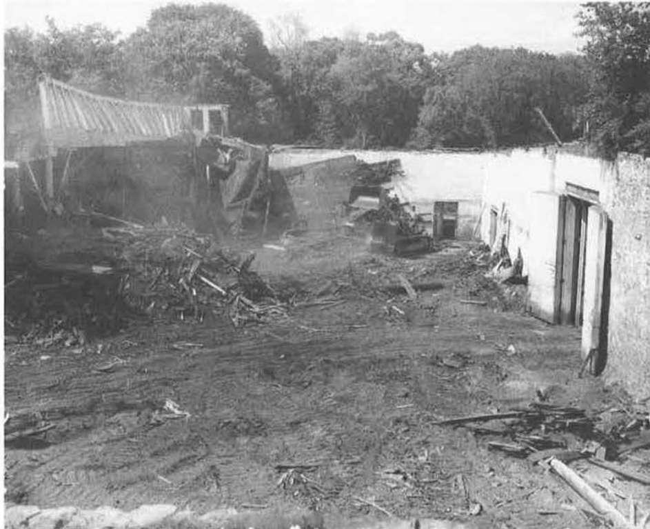
Figure 48. Demolition of roof of 1907 packing cellar in 1958 (Siems collection).
