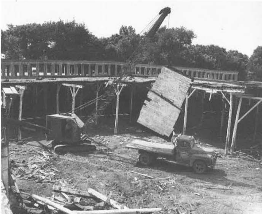
Figure 47. Demolition of roof of 1907 packing cellar in 1958 (Siems collection).
