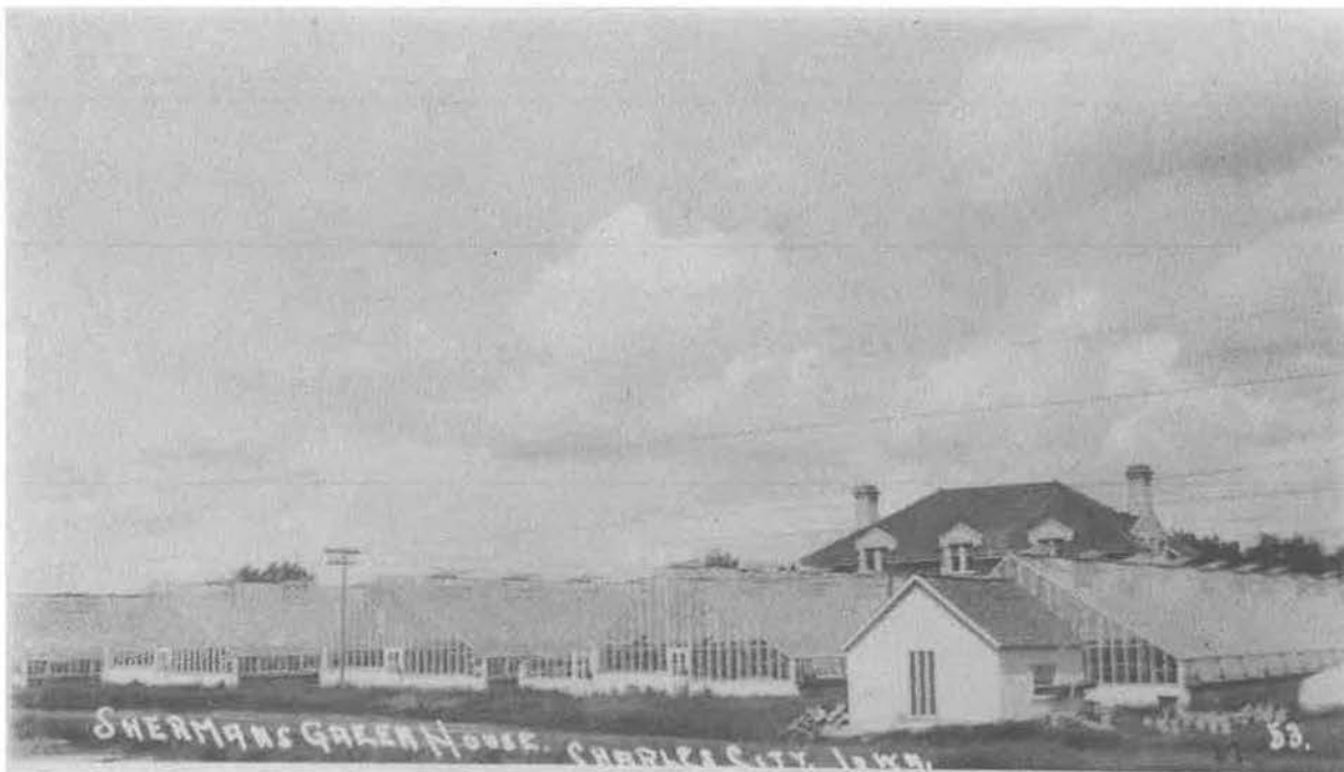
Figure 29. View looking at greenhouses prior to 1914 construction (Floyd County Historical Society).
