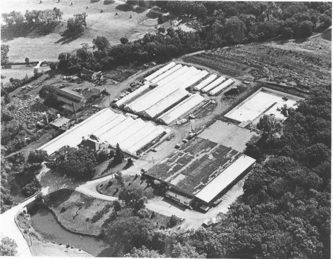
Figure 52. Buildings associated with Sherman Nursery Company in 1976 with new packing/storage building under construction, looking southwest (Siems collection).
