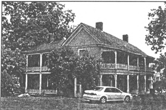
6. Hall House Hotel (site #33), 142 Jackson St., camera facing NW 7. Photo #15
