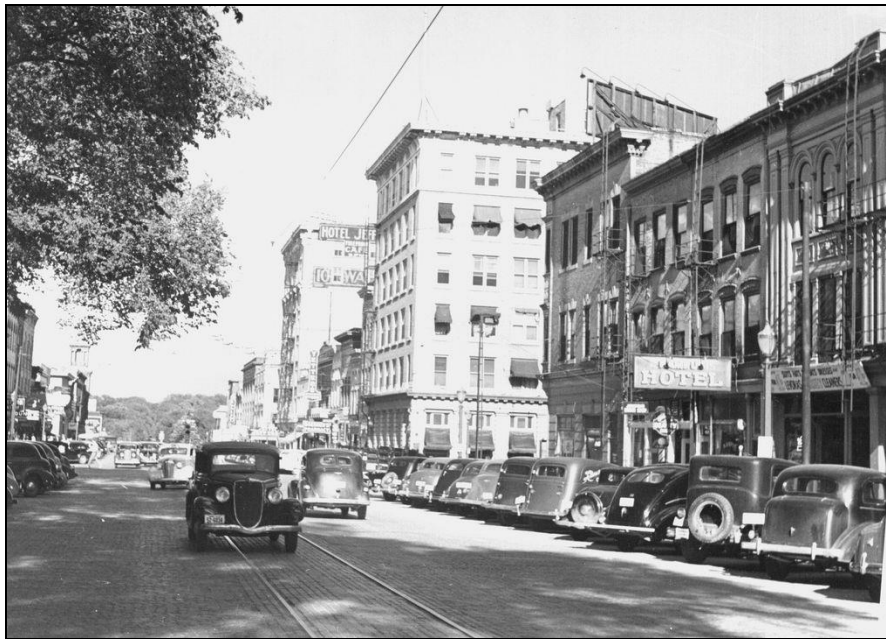
Figure 61: View looking southeast along Washington Street, from west of Clinton Street, ca. 1945 (Kent Photo Collection, University of Iowa)
