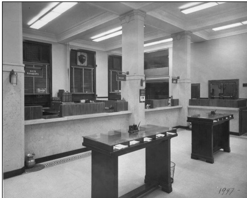
Figure 13: Remodeled lobby view, north area, looking northeast (note mezzanine over vault) (Courtesy Neumann Monson Architects)
