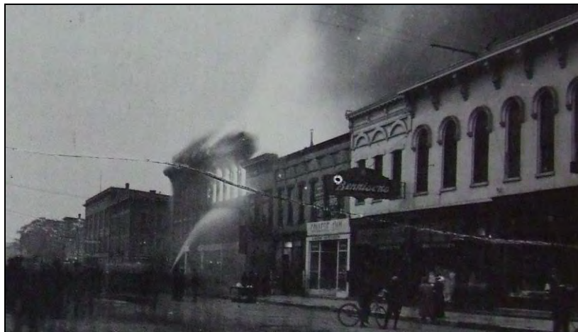
Figure 46: The October 1912 fire, view southeast (Mansheim, p. 154)
