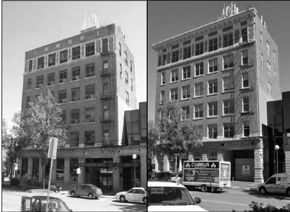
Figures 27-28: West facade, looking northeast, 2014 (left), 2016 (right) (photos courtesy of Neumann Monson Architects, Iowa City)
