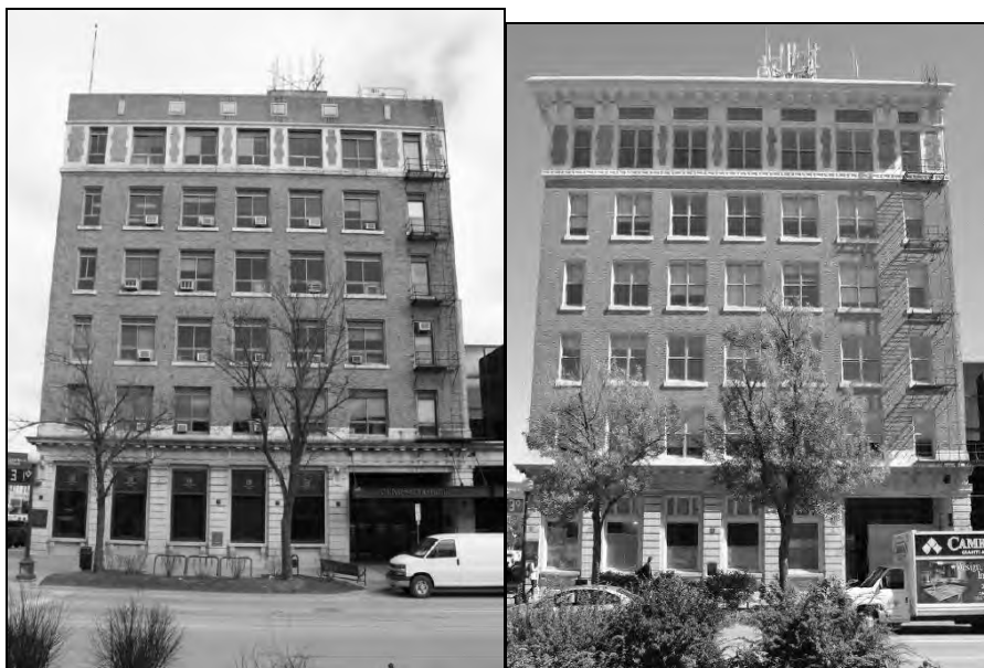
Figures 25-26: West facade, looking east, 2014 (left), 2016 (right) (photos courtesy of Neumann Monson Architects, Iowa City)
