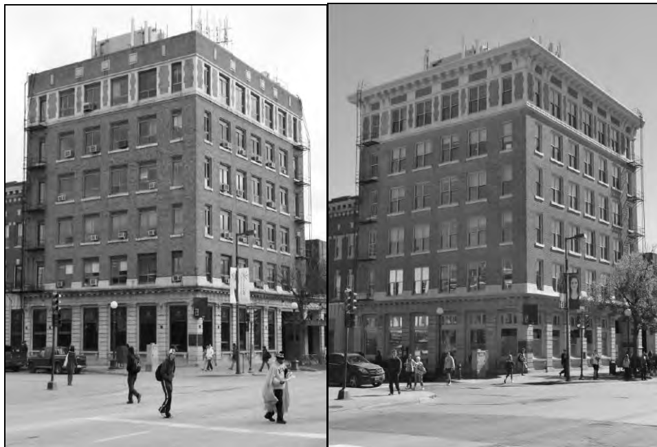
Figures 23-24: North and west facades, looking southeast, 2014 (left), 2016 (right) (photos courtesy of Neumann Monson Architects, Iowa City)
