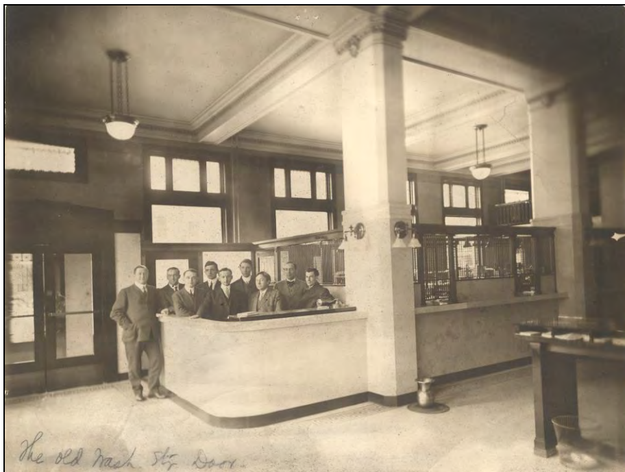
Figure 11: Lobby showing the Washington Street corner entrance at the far left and teller counters, ca.1912, looking northeast (Courtesy Neumann Monson Architects)
