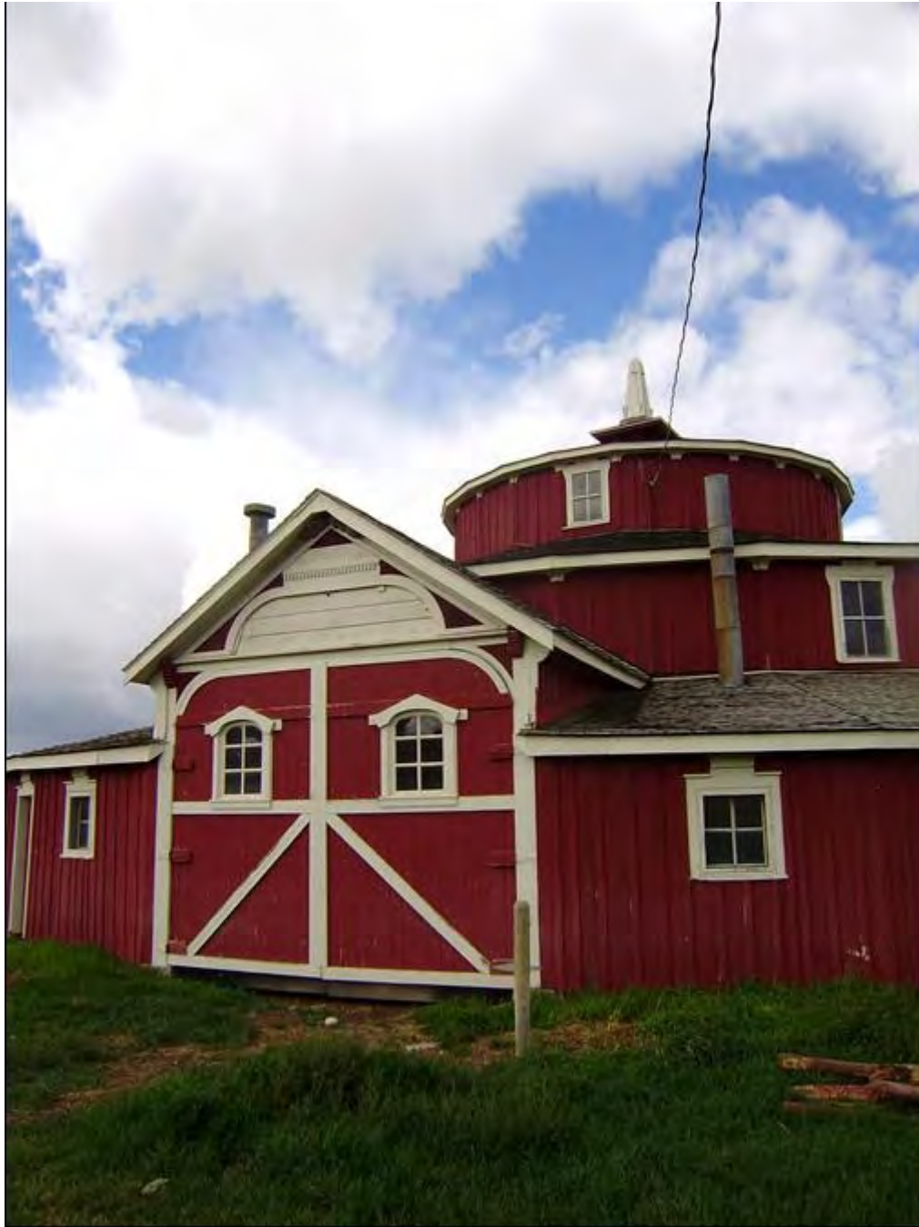
Photo 0008. East facade. View to the west-southwest.
