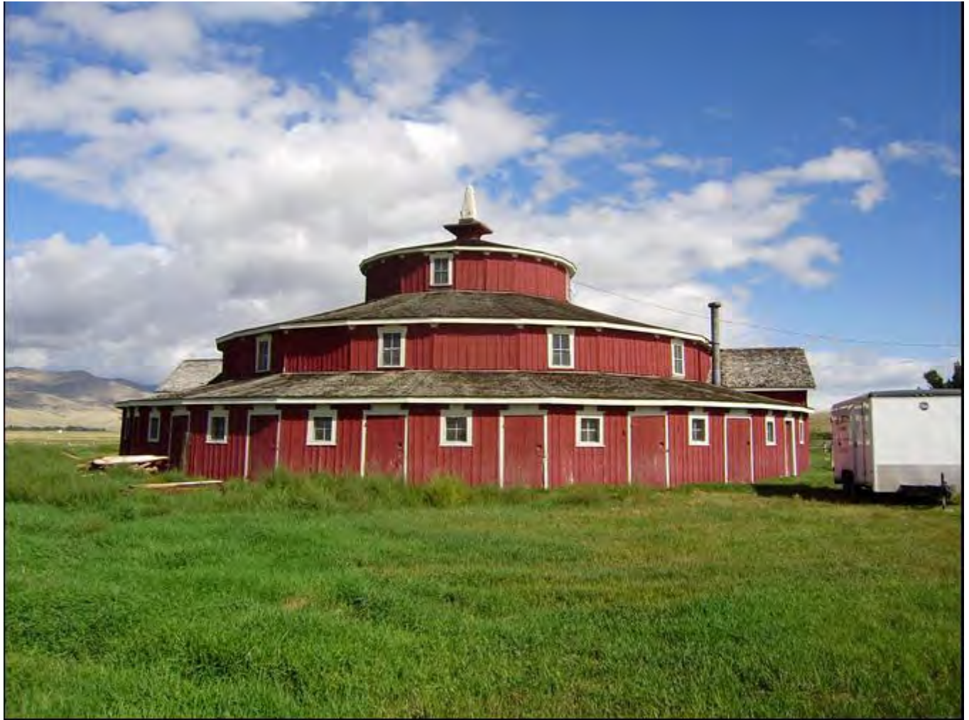
Photo 0007. South elevation of barn. View to the north.
