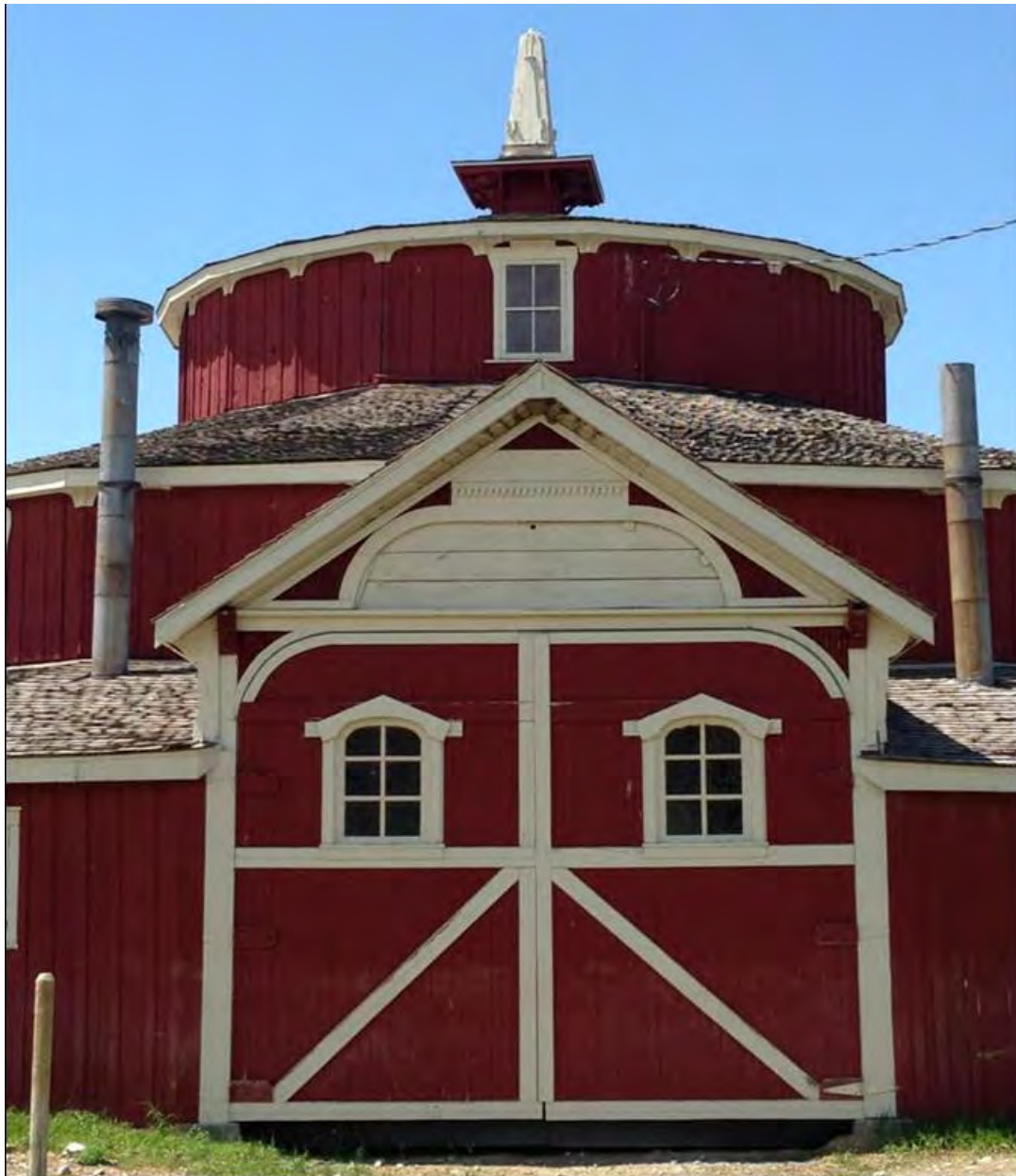
Photo 0009. Detail of primary entry of barn. View to the west.
