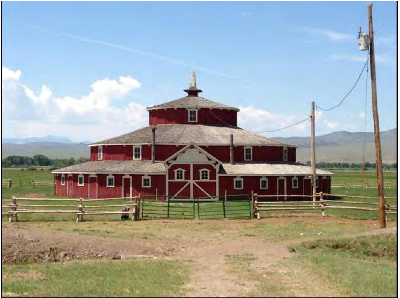
Photo 0001. Façade of Doncaster Round Barn. View to the west.
