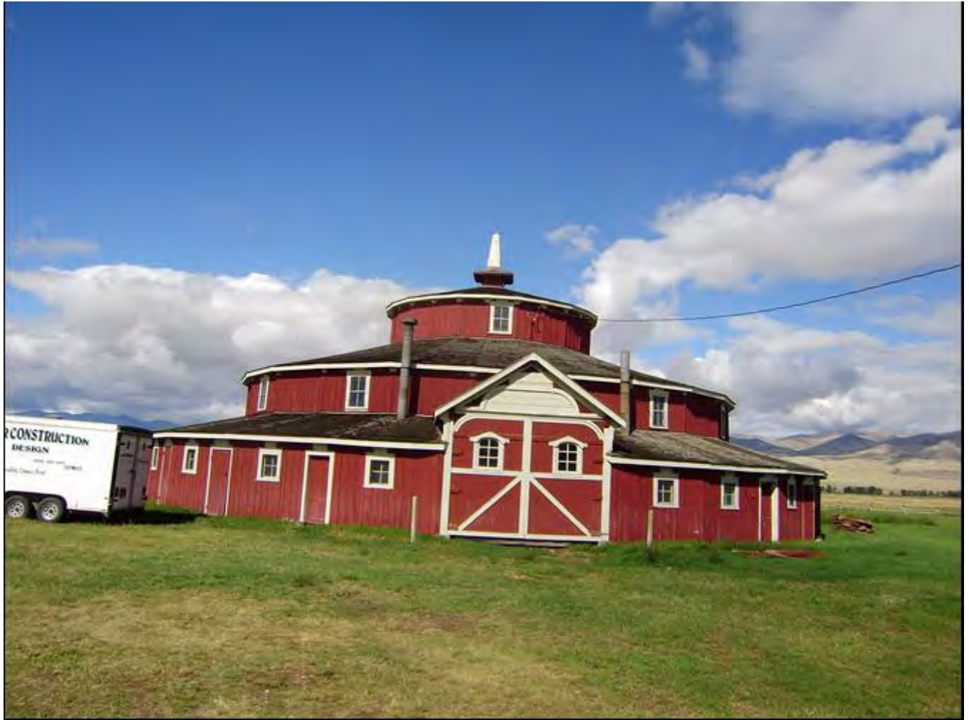
Photo 0002. Façade of barn. View to the west.
