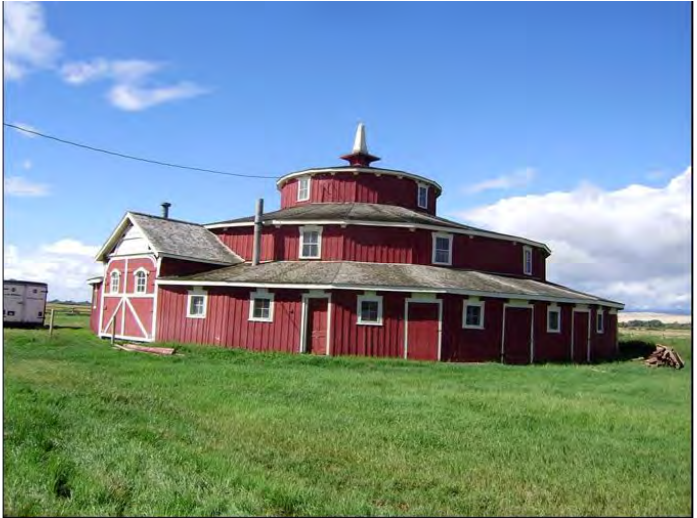
Photo 0003. Façade and north elevation of barn. View to the south.
