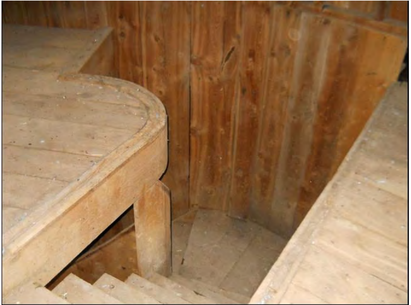
Photo 0017. Detail showing staircase to second floor.
