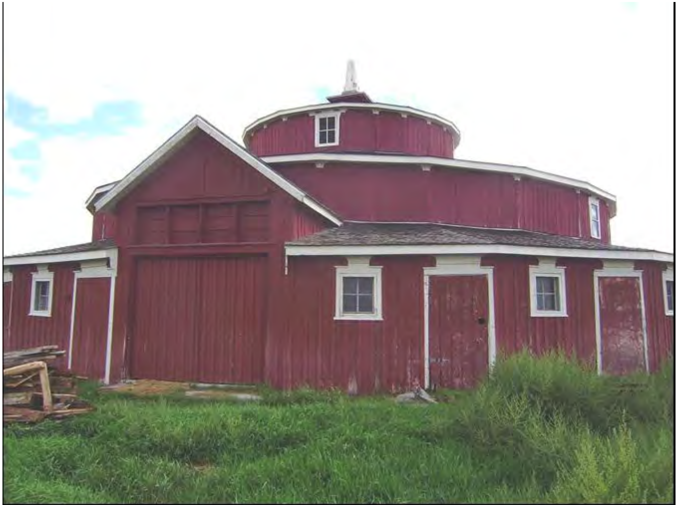
Photo 0005. West façade and west entry of barn. View to the east.
