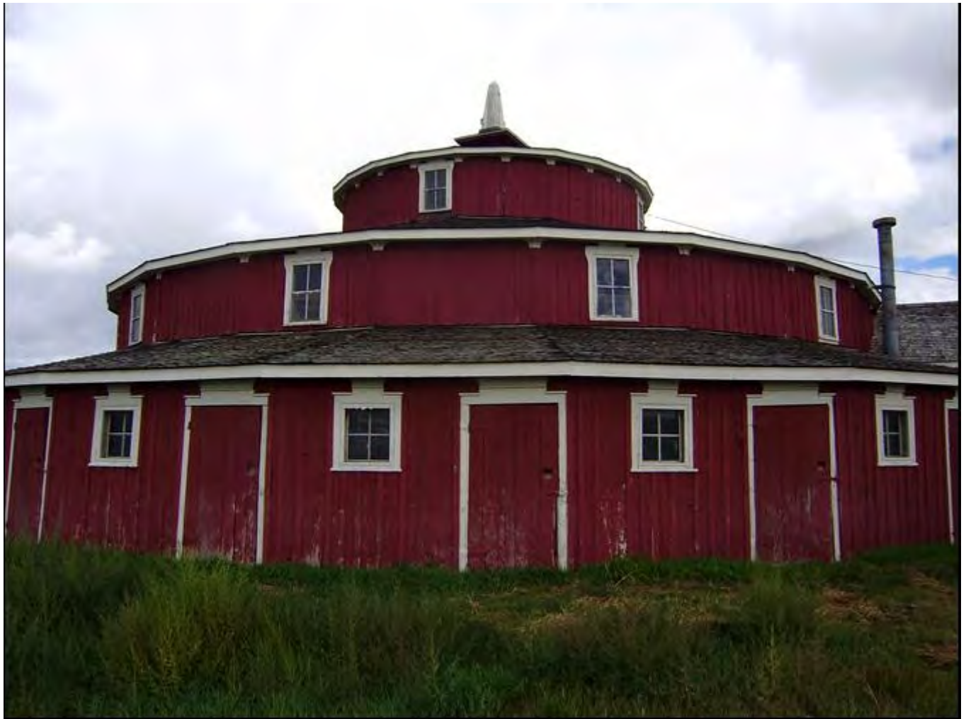
Photo 0010. Detail of south elevation of barn. View to the north.
