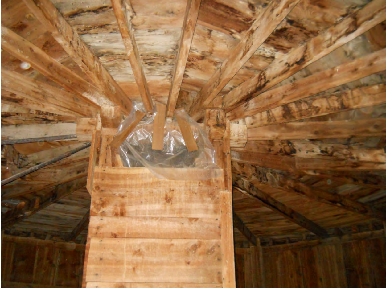
Photo 0015. Interior detail of ceiling joists.
