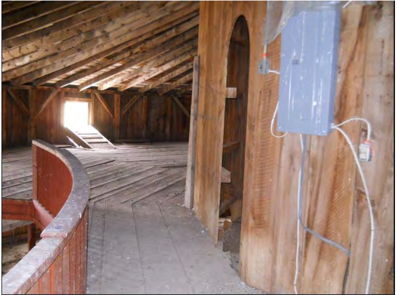
Photo 0016. Second floor showing grain distribution system at window.
