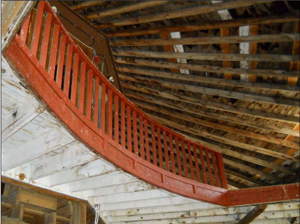
Photo 0014. Interior detail of second floor balcony railing and ceiling joists.
