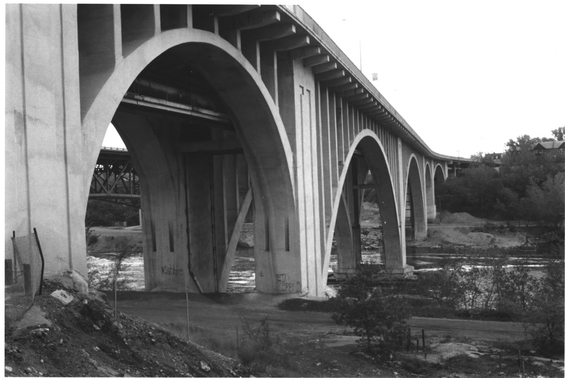
CEDAR AVENUE BRIDGE, NO. 2796 HENNIPEN CO., MN PHOTO I.D. 09971 #20A
