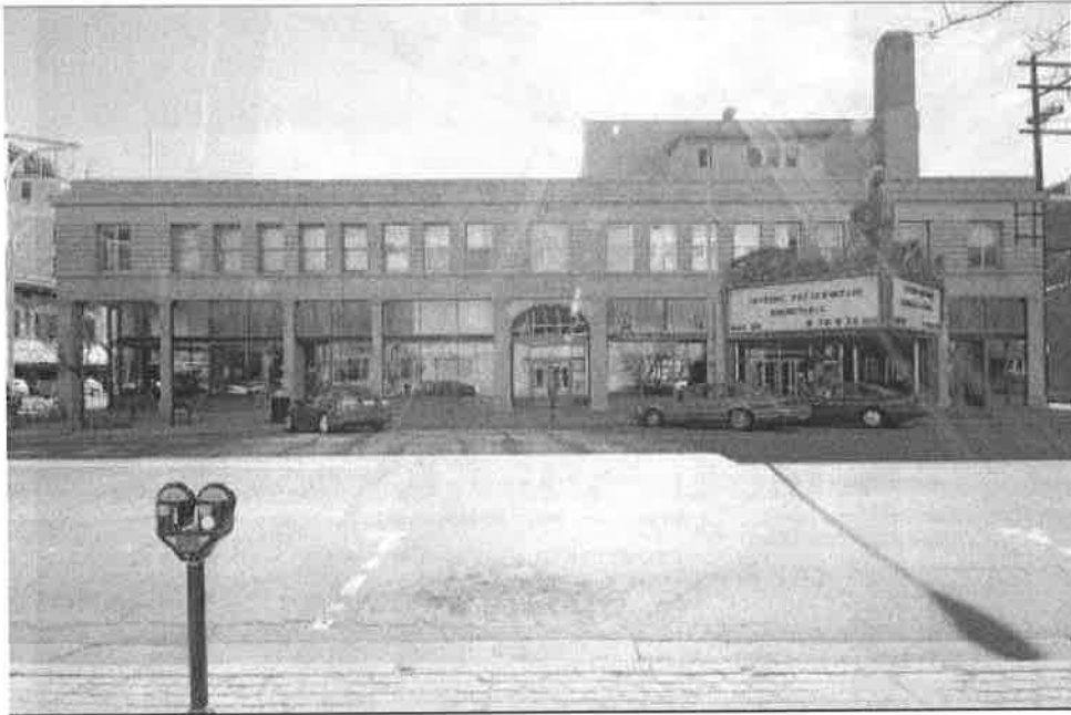
Photo #0004 (MT_YellowstoneCounty_BabcockTheatreBld_0004) View of north elevation, view to the S
