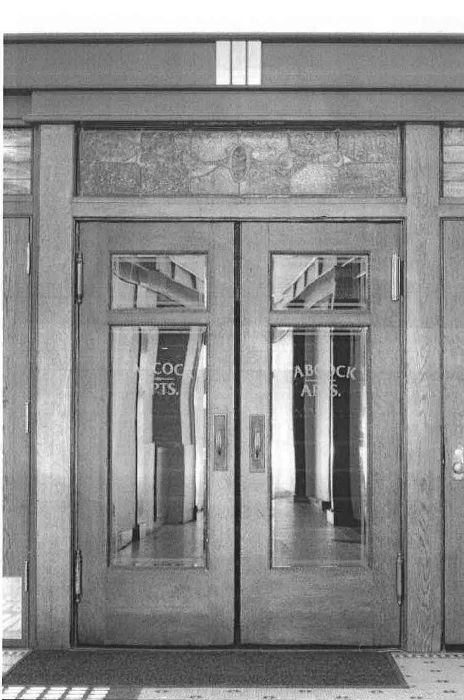
Close up of original doors to apartments
