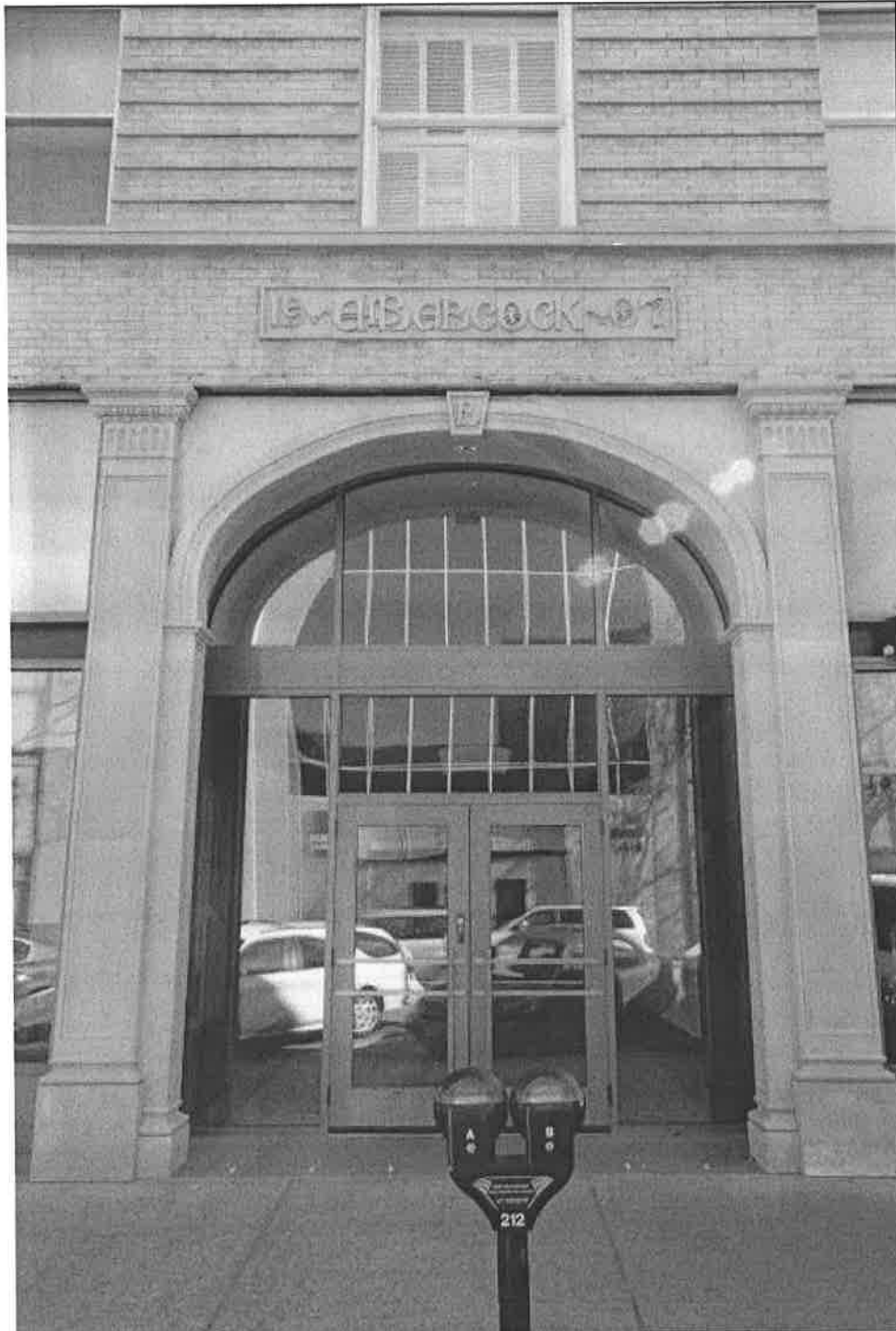
Photo #0024 (MT_YellowstoneCounty_BabcockTheatreBld_0024) North side entry to arcade, view to the S
