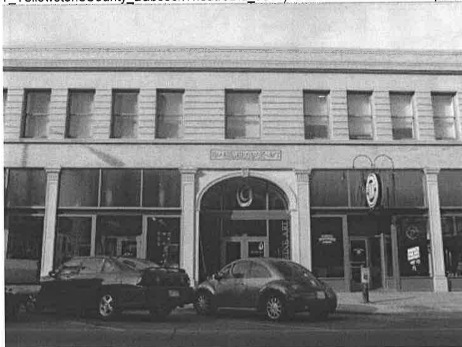
Photo #0014 (MT_YellowstoneCounty_BabcockTheatreBld_0014). East elevation middle portion, view to the W
