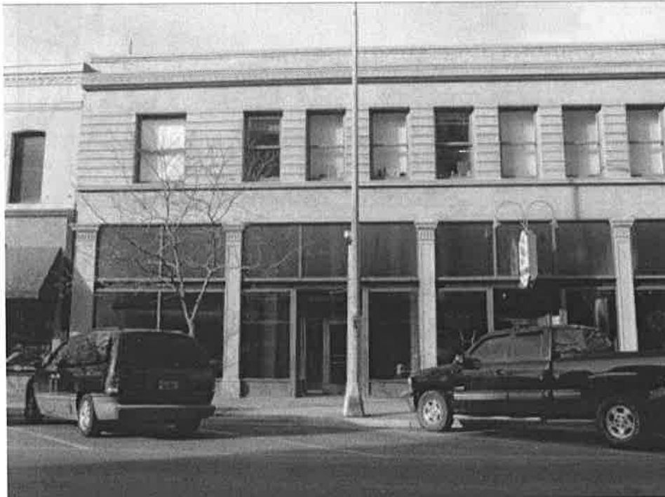
Photo #0013 (MT_YellowstoneCounty_BabcockTheatreBld_0013). East elevation southern portion, view to the W
