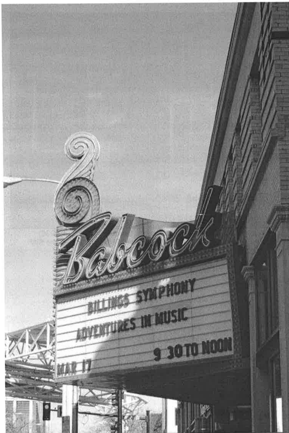
Photo #0029 (MT_YellowstoneCounty_BabcockTheatreBld_0029) Theatre marquee, view to the E
