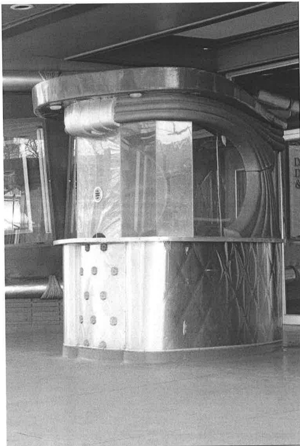
Photo #0031 (MT_YellowstoneCounty_BabcockTheatreBld_0031) Ticket booth, view to the SE
