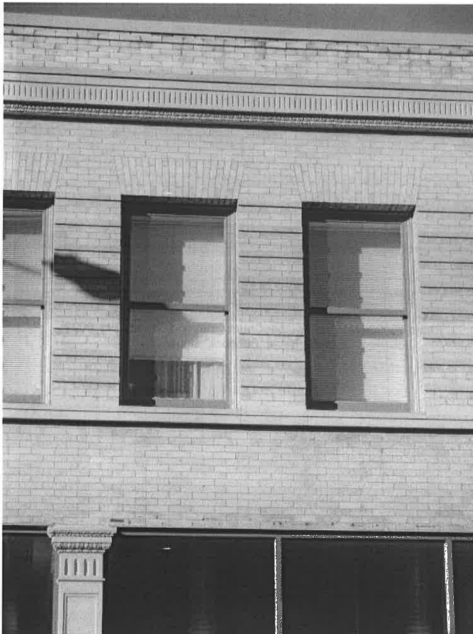
Photo #0023 (MT_YellowstoneCounty_BabcockTheatreBld_0023) 2 nd floor wall detail, view to the W
