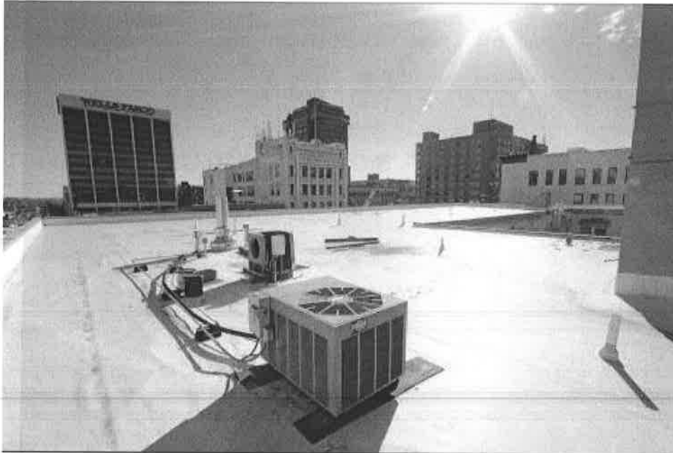
Photo #0007 (MT_YellowstoneCounty_BabcockTheatreBld_0007) Roof above apartments looking southeast
