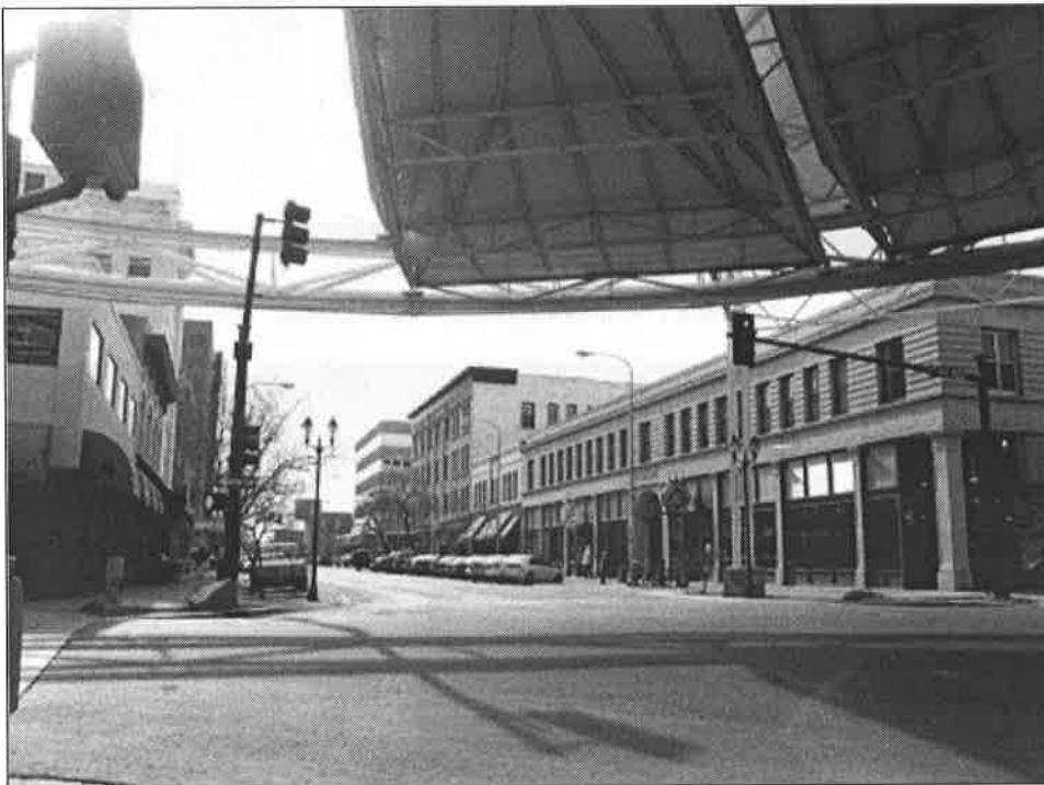
Photo #0001 (MT_YellowstoneCounty_BabcockTheatreBld_0001). View of neighborhood at east elevation, view to the SW
