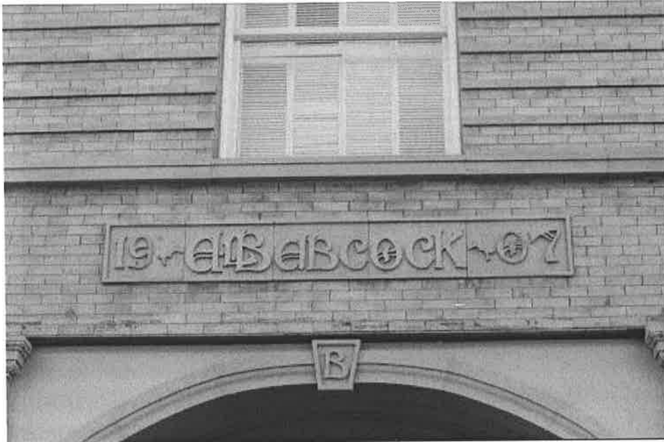
Photo #0022 (MT_YellowstoneCounty_BabcockTheatreBld_0022) Exterior detail "Babcock" signage
