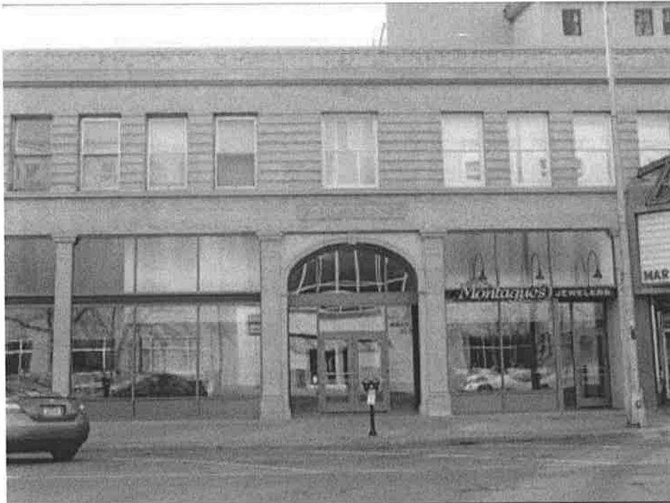
Photo #0017 (MT_YellowstoneCounty_BabcockTheatreBld_0017). North elevation middle portion, view to the S
