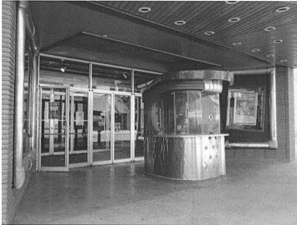
Photo #0030 (MT_YellowstoneCounty_BabcockTheatreBld_0030) Theatre entry under marquee on north side of building, view to the SW
