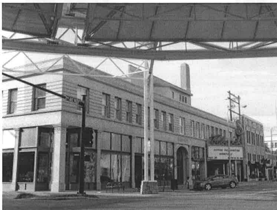
Photo #0003 (MT_YellowstoneCounty_BabcockTheatreBld_0003). View of North Elevation from corner, view to the SW
