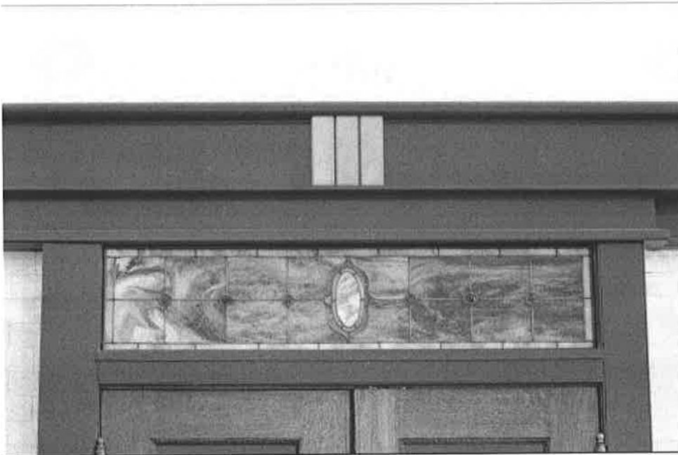
Close up of original stained glass at apartment door area
