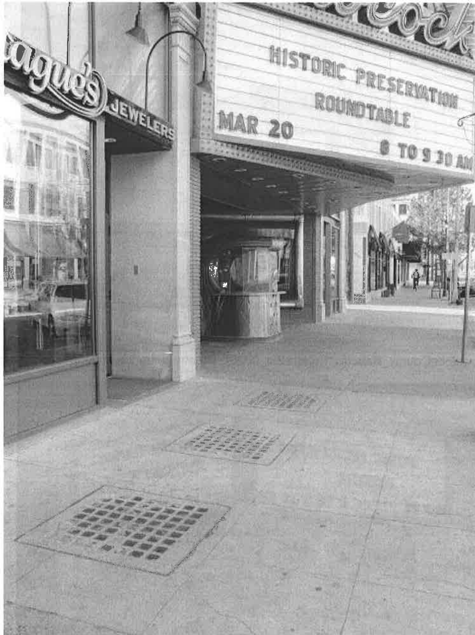
Photo #0028 (MT_YellowstoneCounty_BabcockTheatreBld_0028) Exterior detail prism glass in north sidewalk, view to the W
