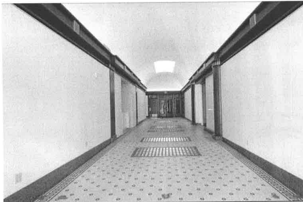
Interior of north entry – arcade looking south
