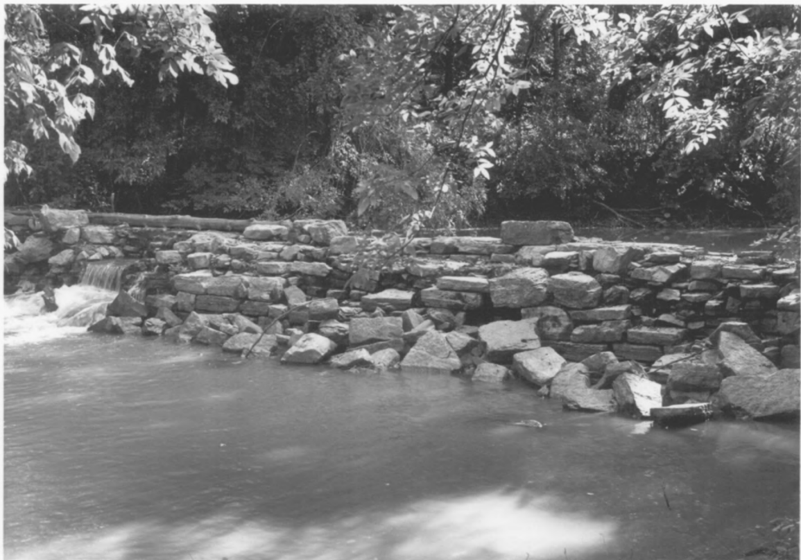
Shaddon Mill Site, Blount Co., TN, Photo 2 of 2
