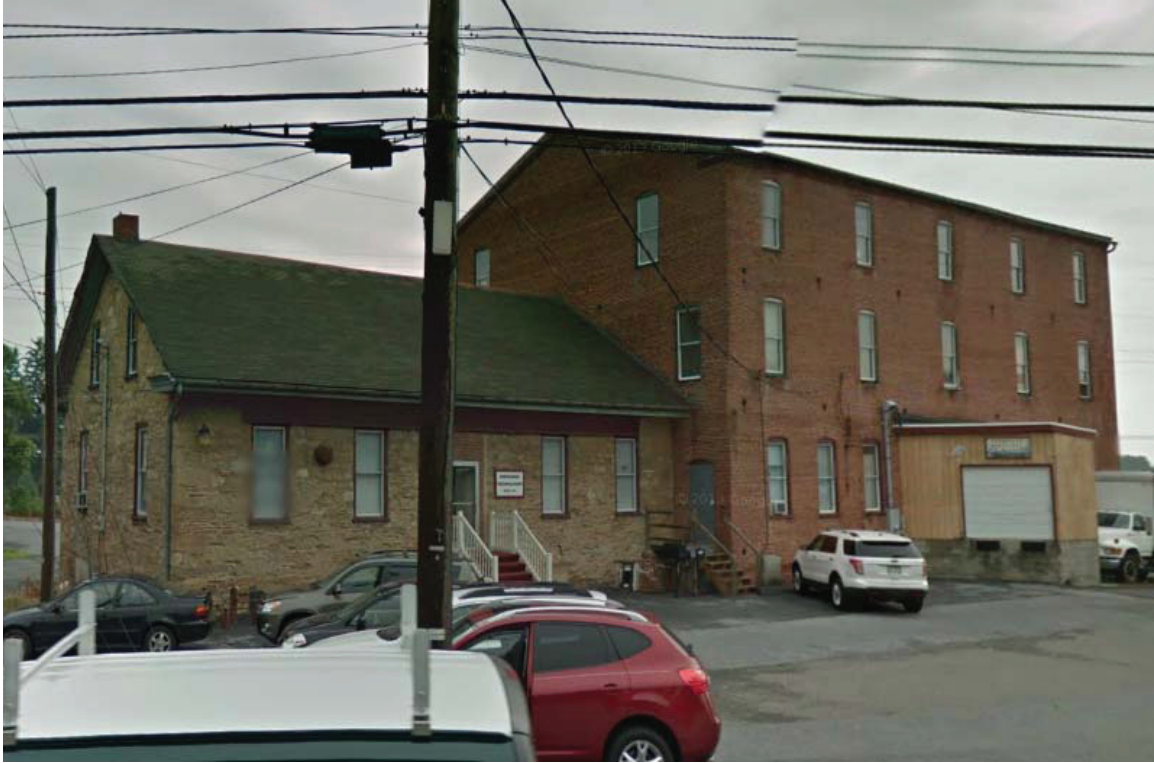
Phares Nissley & Company Tobacco Warehouse (ca. 1910), Main Street, Salunga. Note the replacement windows and altered entrances (Source: Google Earth, July 2013).
