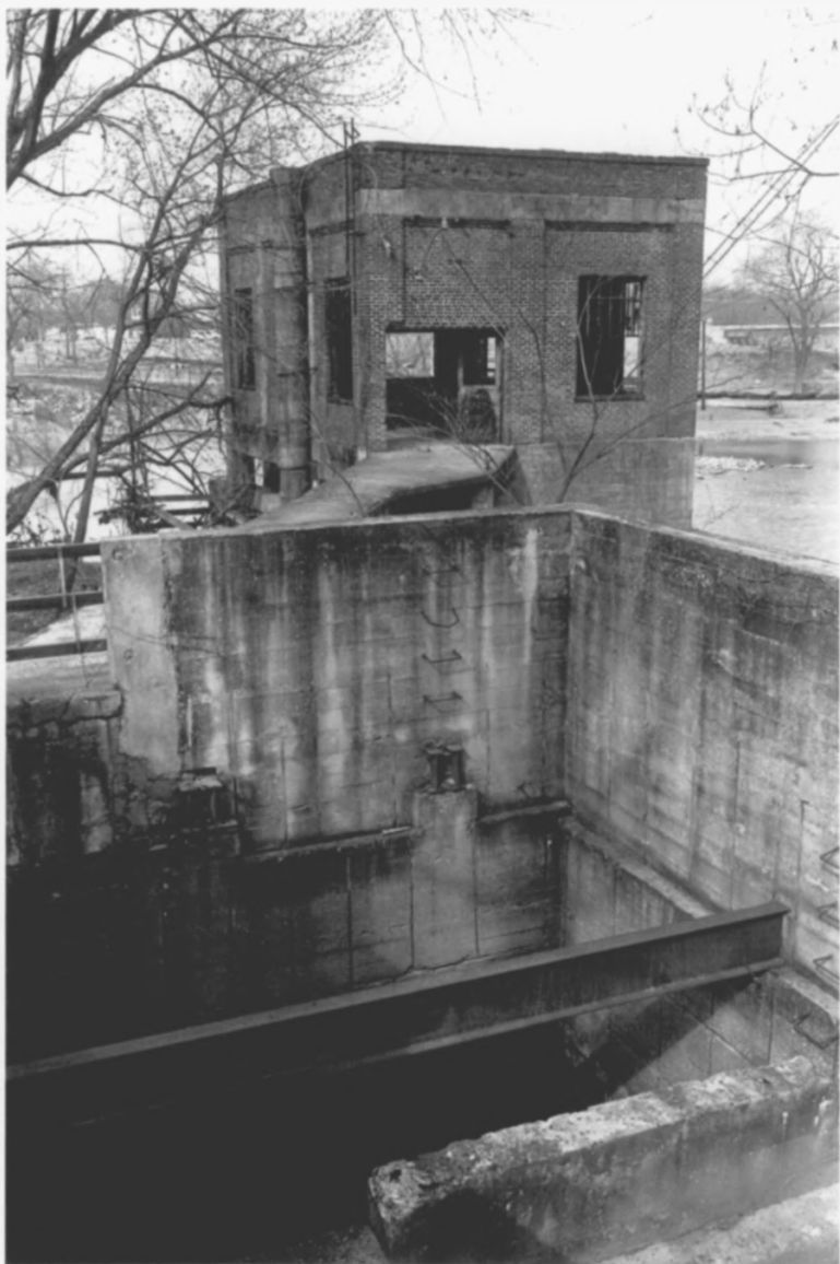
Shelbyville Hydroelectric Station Shelbyville, Bedford County, TN
