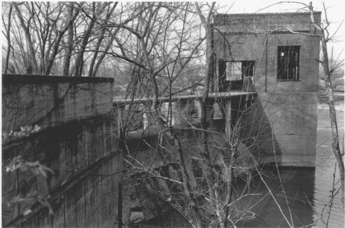
Shelbyville Hydroelectric Station Shelbyville, Bedford County, TN
