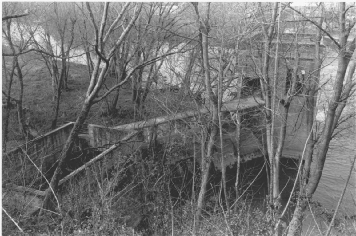
Shelbyville Hydroelectric Station Shelbyville, Bedford County, TN
