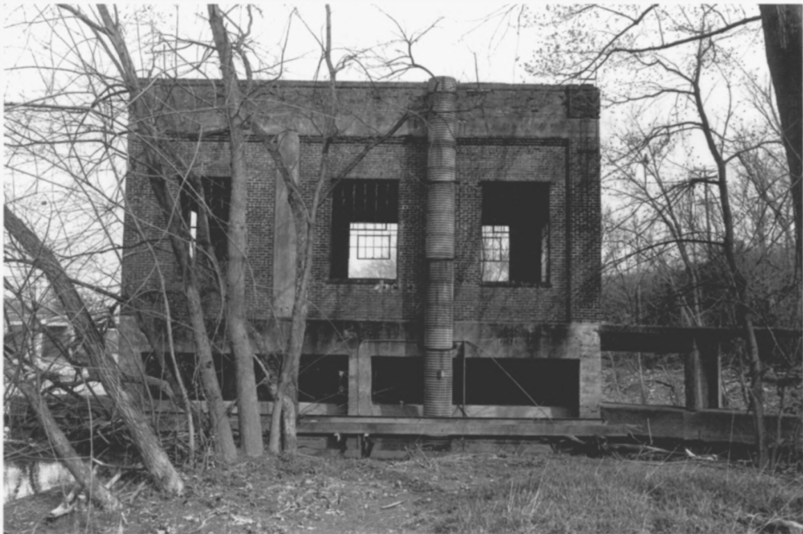
Shelbyville Hydroelectric Station Shelbyville, Bedford County, TN
