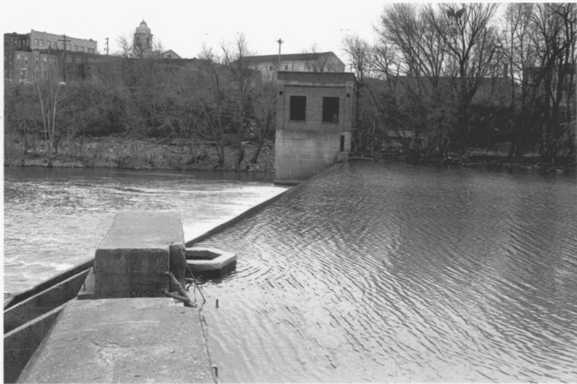
Shelbyville Hydroelectric Station Shelbyville, Bedford County, TN
