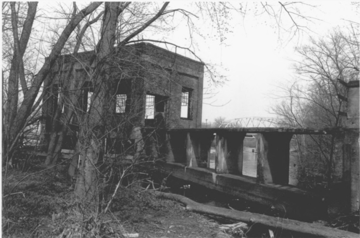
Shelbyville Hydroelectric Station Shelbyville, Bedford County, TN
