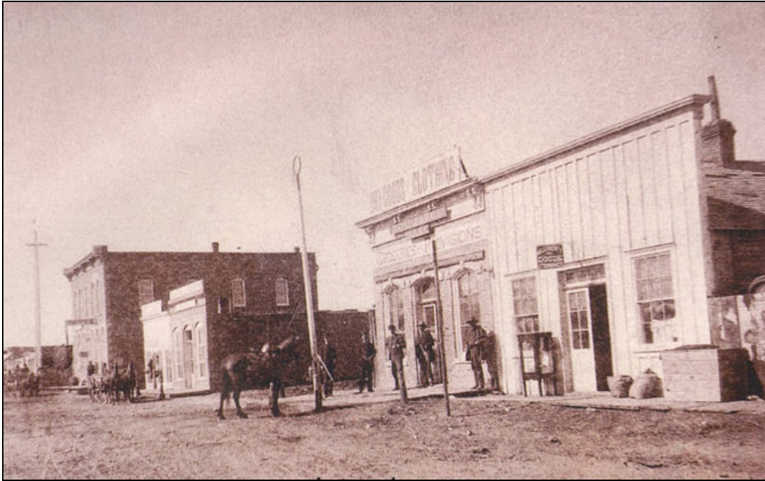
Figure 4. This pre-1882 view southwest shows the west side of the 300 block (odd numbers) of 4 th Street. The two-story Dunn Block (5SH.1901) looms in the distance to the left with a one-story building and the north part of 313-15 4 th Street (5SH.1902) to its right. The brick-faced adobe building with segmental arches at center housed the Gotthelf and Mayer mercantile (number 307). A false front adobe building is present at the right. The two buildings to the right now comprise 307 4 th Street (5SH.1904) under a common false front façade. Courtesy Saguache Chamber of Commerce, photograph, pre-1882, Saguache, Colorado.
