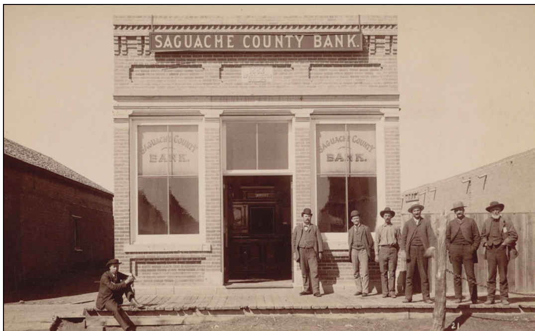
Figure 7. By 1882, the Saguache County Bank had outgrown its space in the Gotthelf and Mayer building (right) and this building at 311 4 th Street (5SH.1900) was erected to house its operations. The building plaque below the signband reads "1882 J.F. Farrington builder." The walls of 313-15 (5SH.1902) and 307 4 th Street (5SH.1904) are shown to the left and right, respectively. Courtesy Amon Carter Museum, photographic collection, image number P1976.11.226, ca. 1880s, Fort Worth, Texas.
