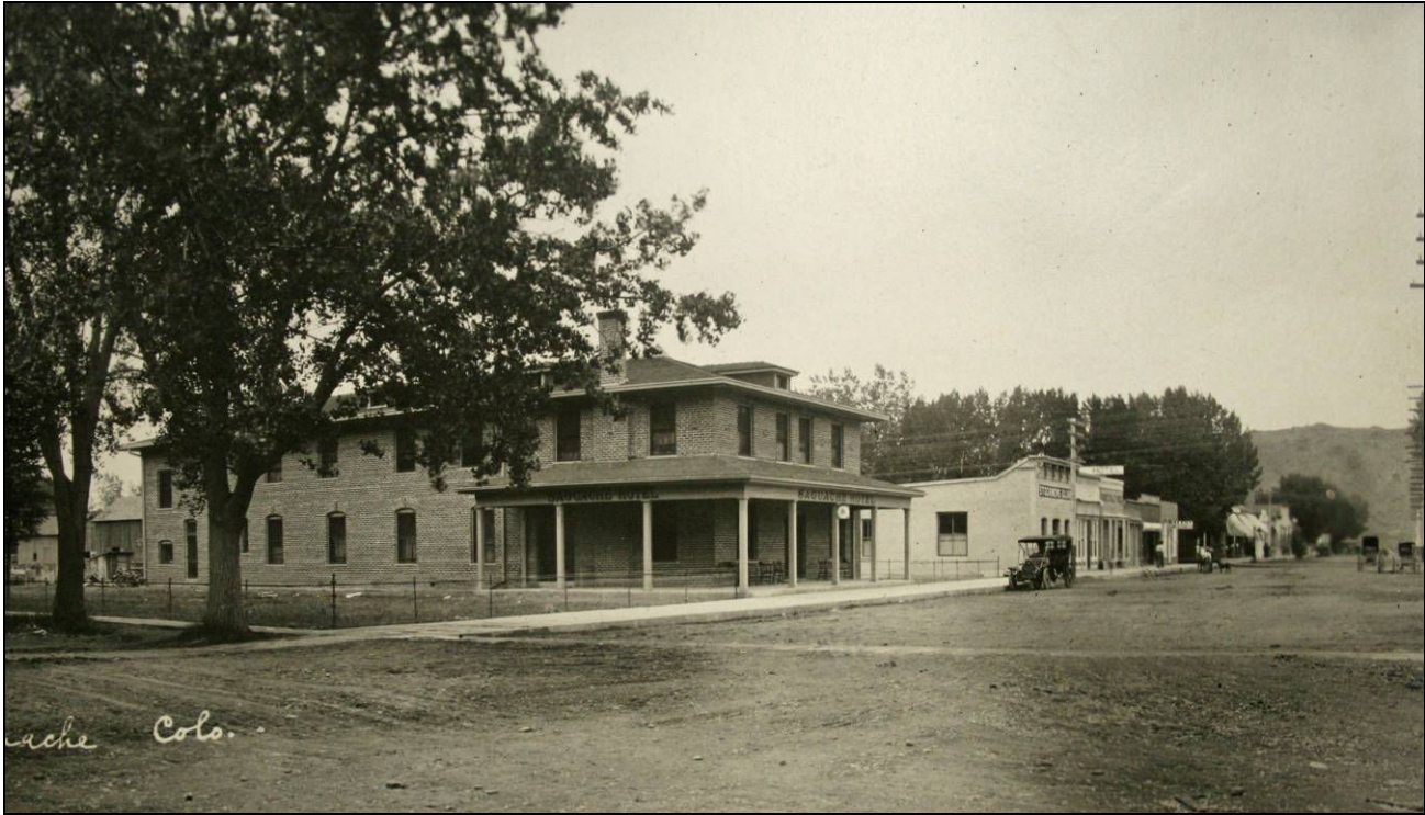
Figure 14. The new Saguache Hotel (left) dominates this ca. 1912 view of the west side of the 400 block of 4 th Street. Cottonwoods and a segment of the street ditch on the north side of Christy Avenue are at the extreme left. Courtesy Saguache County Museum, photograph collection, ca. 1912, Saguache, Colorado.
