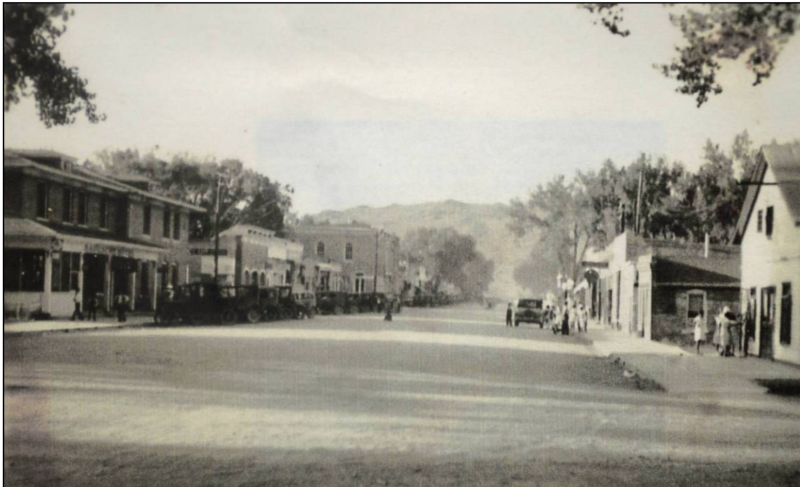
Figure 20. This ca. early 1920s view north up 4 th Street from Christy Avenue shows the 1910 Saguache Hotel (5SH.384) at the left with its ca. 1920 north wing. The building at the right housed the Rialto Theater; it burned in 1926. To its north is 416-18 4 th Street (5SH.4591), which then had a brick false front. Courtesy Saguache County Museum, photograph collection, early 1920s, Saguache, Colorado.
