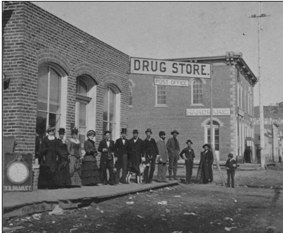
Figure 6. The Pioneer Drug Store (401 4 th Street, 5SH.4586), which also housed the Post Office and jeweler W.R. Bradley, is in the foreground with the Dunn Block (5SH.1901) beyond in this early 1880s view to the north-northwest. Courtesy Amon Carter Museum, photographic collection, image number P1976.24.386, ca. 1882-84, Fort Worth, Texas.
