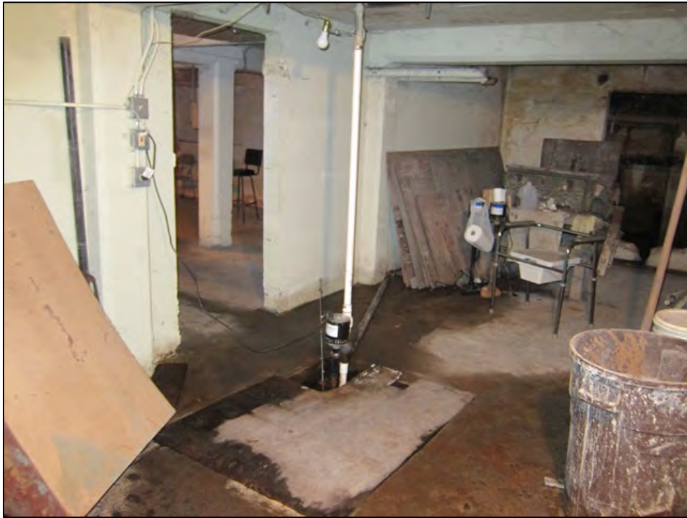
Photo 9 of 16: Interior of basement room east of central stair, looking northwest
