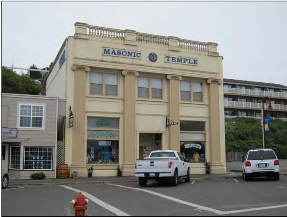
Photo 1 of 16: Northern elevation of building, looking south
