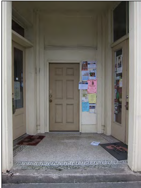
Photo 6 of 16: Front entry on northern elevation, looking south
