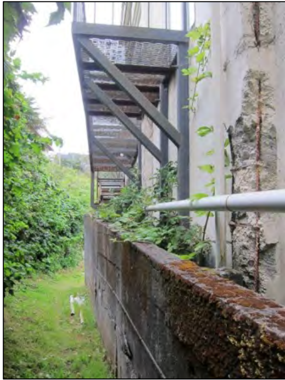
Photo 5 of 16: Southern elevation detail of retaining wall, looking west
