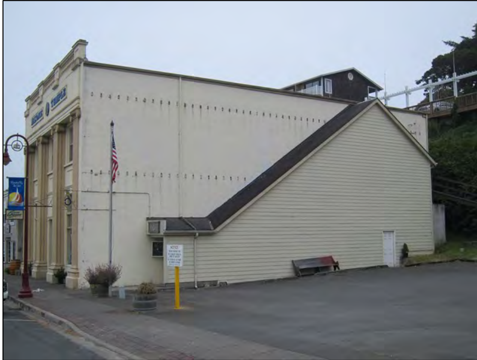
Photo 3 of 16: Western elevation of building, looking east
