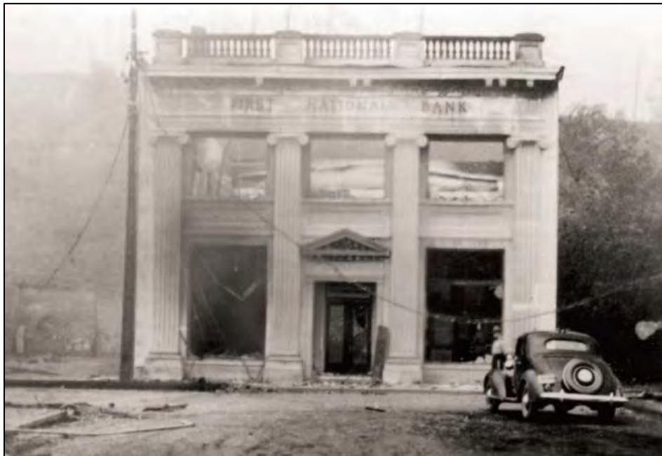
Figure 9: Historic Photo from 1936 fire, North Elevation. Courtesy of Bandon Historical Society and Museum.
