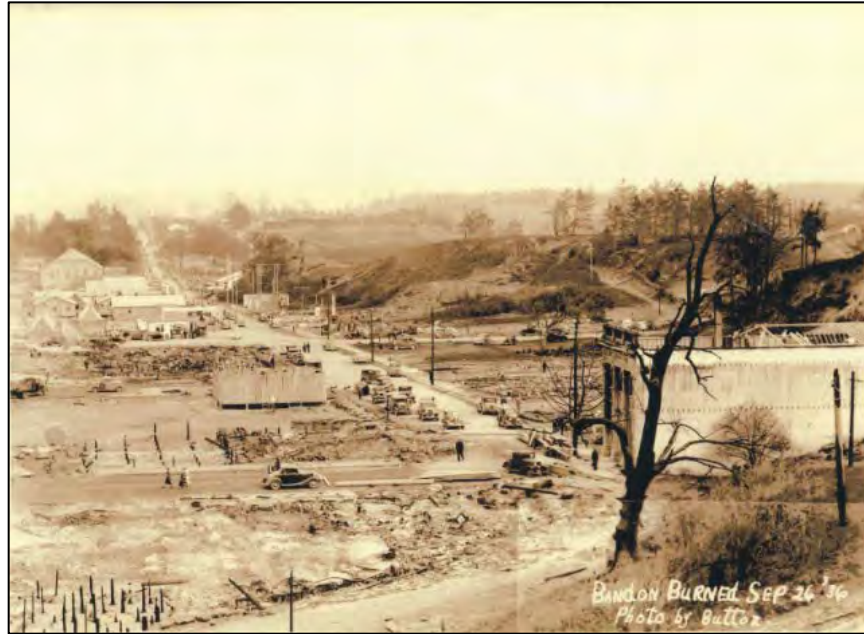
Figure 10: Historic Photo from 1936 fire, site photo. Courtesy of Bandon Historical Society and Museum. Note the roof being rebuilt.
