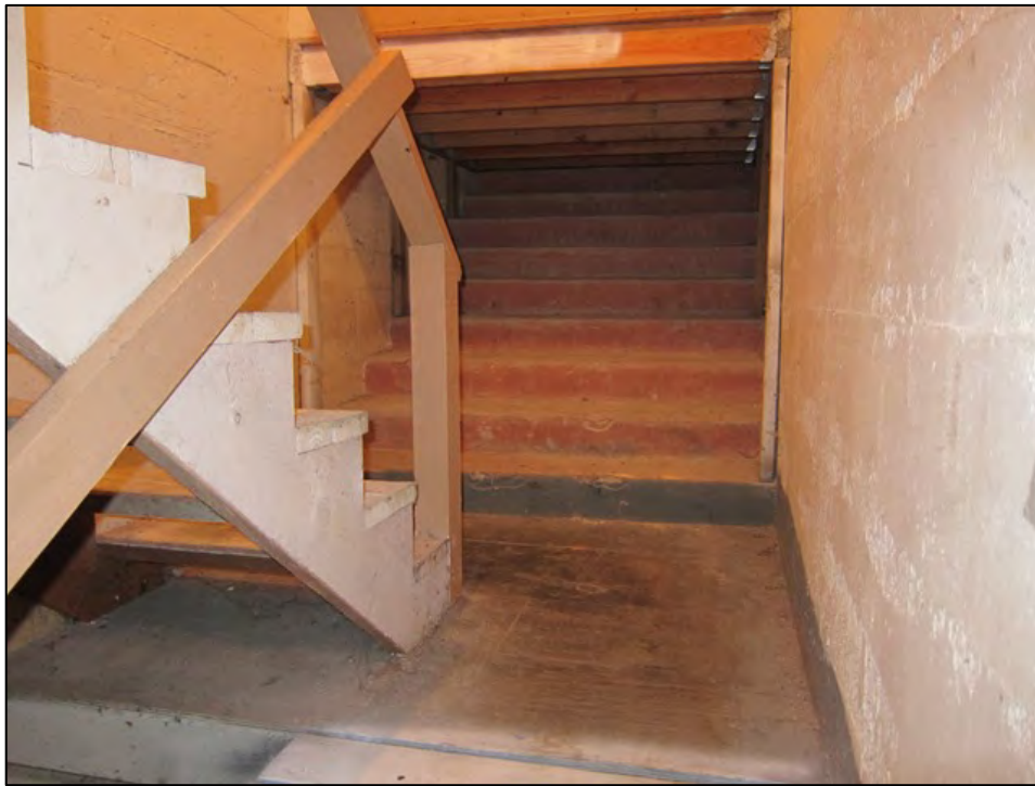
Photo 8 of 16: Interior detail of central stairway from basement, looking south
