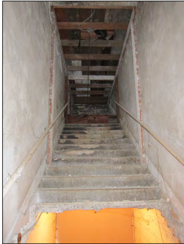
Photo 7 of 16: Interior detail of central stairway remnants, looking south
