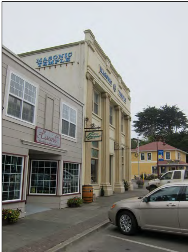
Photo 2 of 16: Northern and eastern elevation of building, looking southwest
