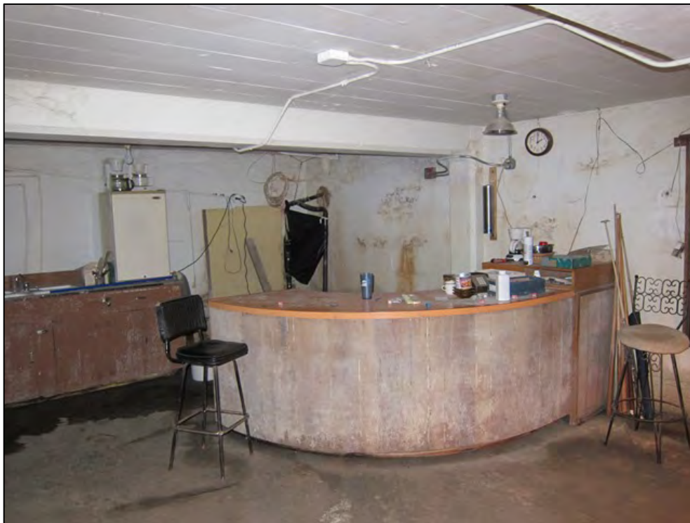
Photo 10 of 16: Interior of basement room west of central stair, looking southwest
