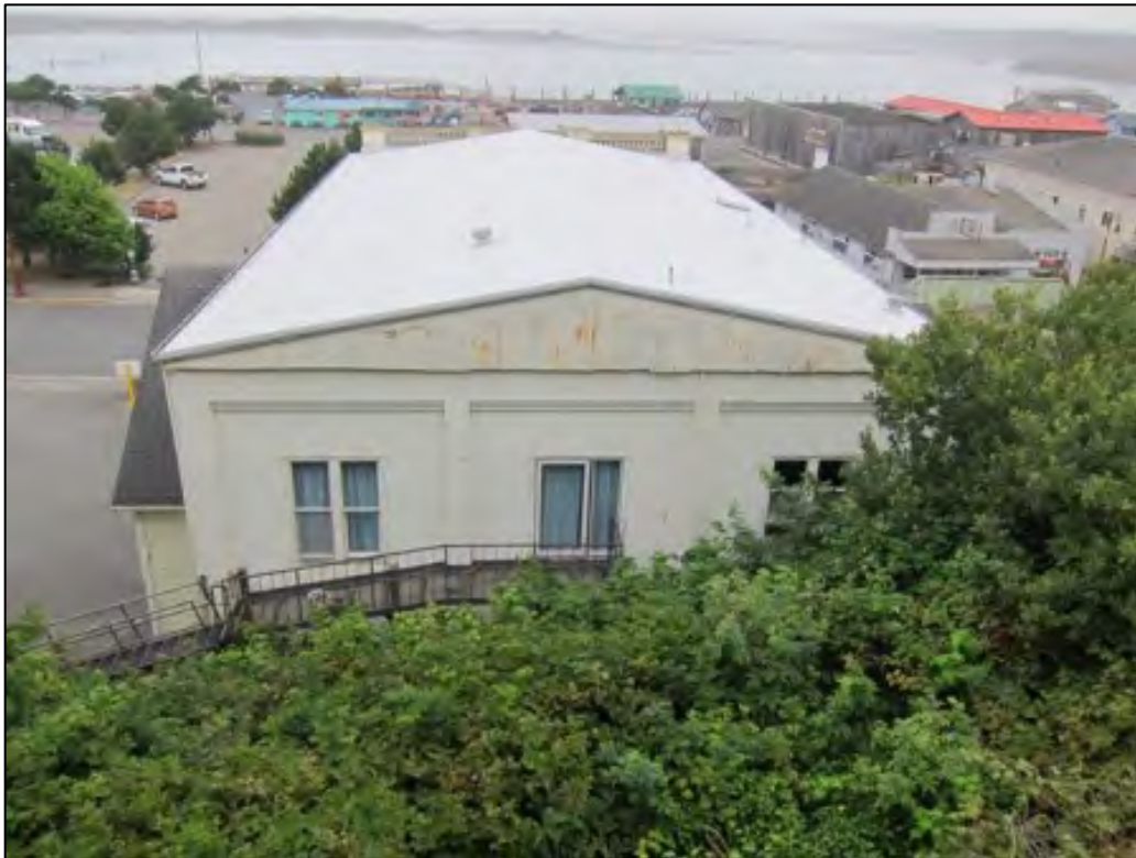
Photo 4 of 16: Southern elevation of building and roof, looking north
