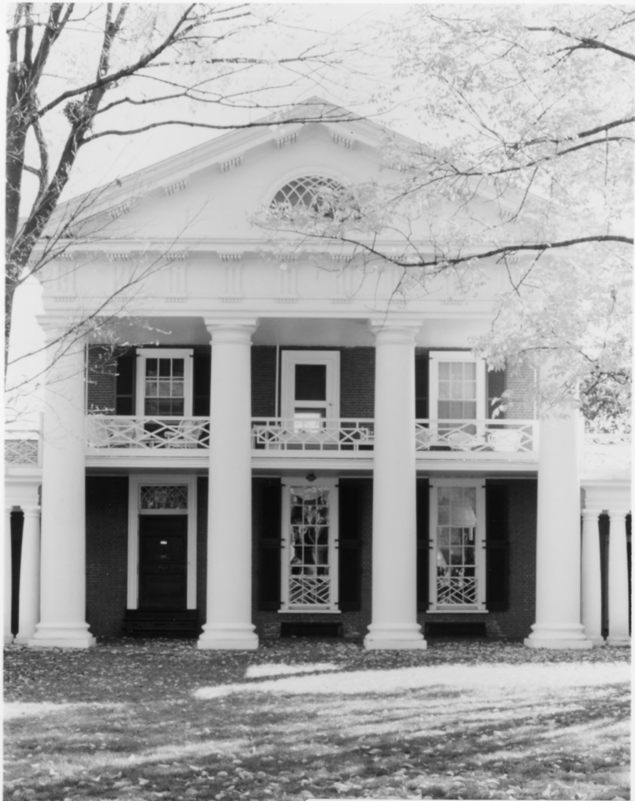
17. Pavilion IV, facade
