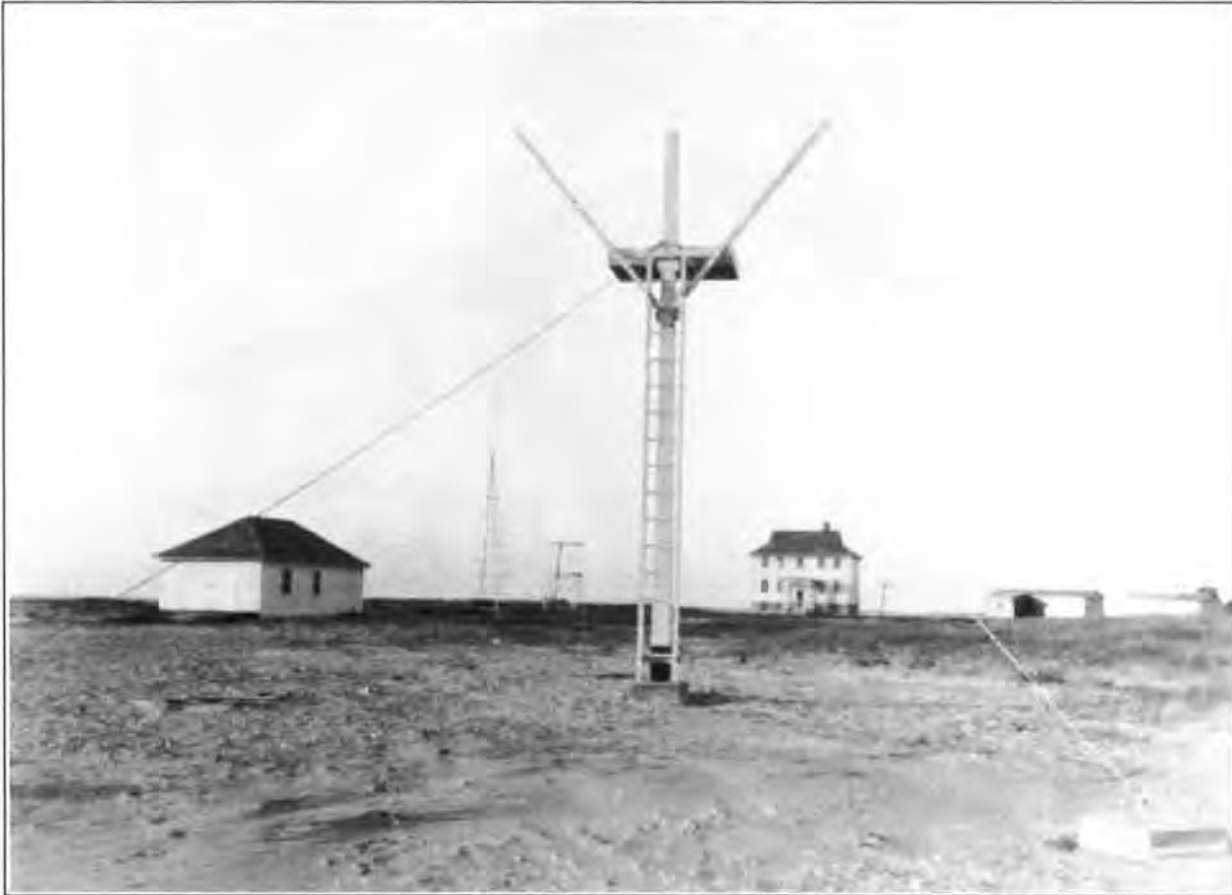
Figure 10. Historical photograph showing USCG Garage/Boathouse, circa 1925. View looking north/northwest (reproduced in Phillips 2007:42).
