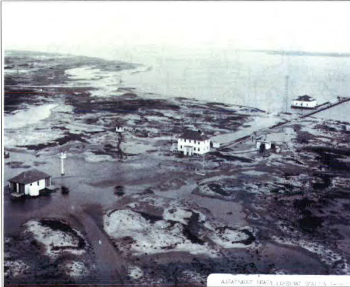
Figure 8. Aerial view of Assateague Beach Coast Guard Station, March 8, 1962 (reproduced in Phillips 2007:25).
