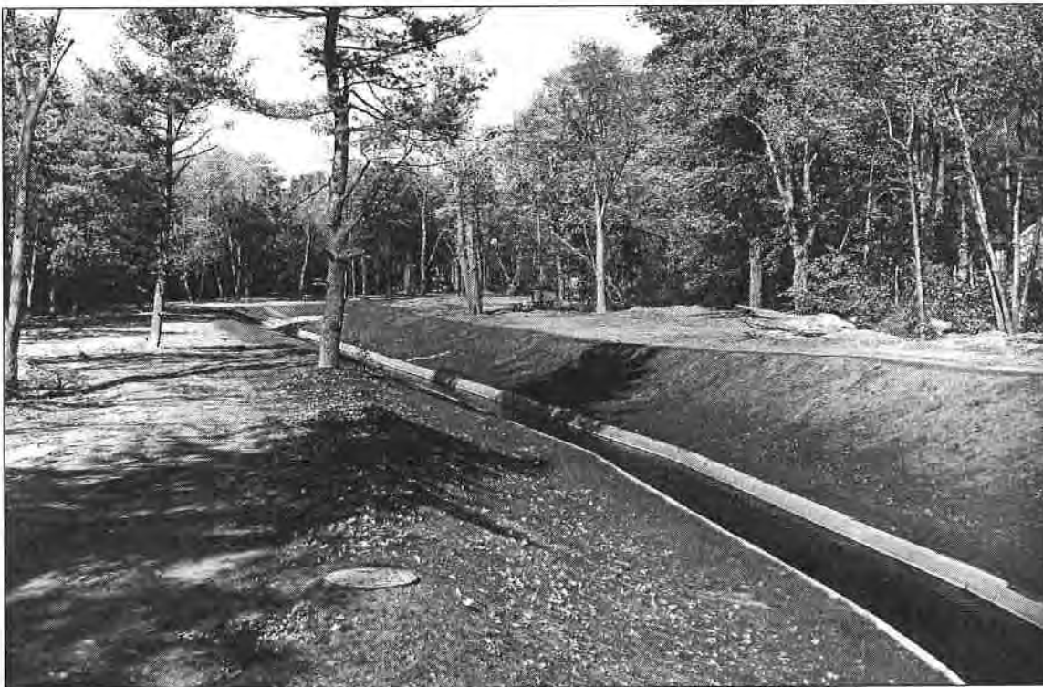
View of Fuller Brook near Denton Road after concrete curbing was installed, circa 1958. (Wellesley Natural Resources Commission files)
