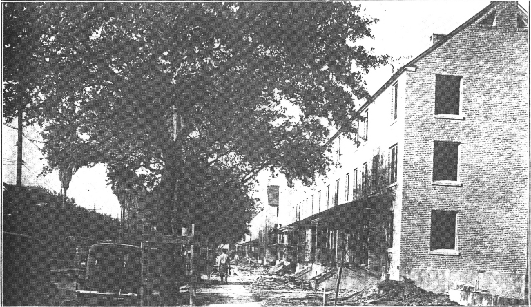
NEARLY COMPLETED SECTION OF MAGNOLIA PROJECT LOOKING OUT LOUISIANA AVENUE.
