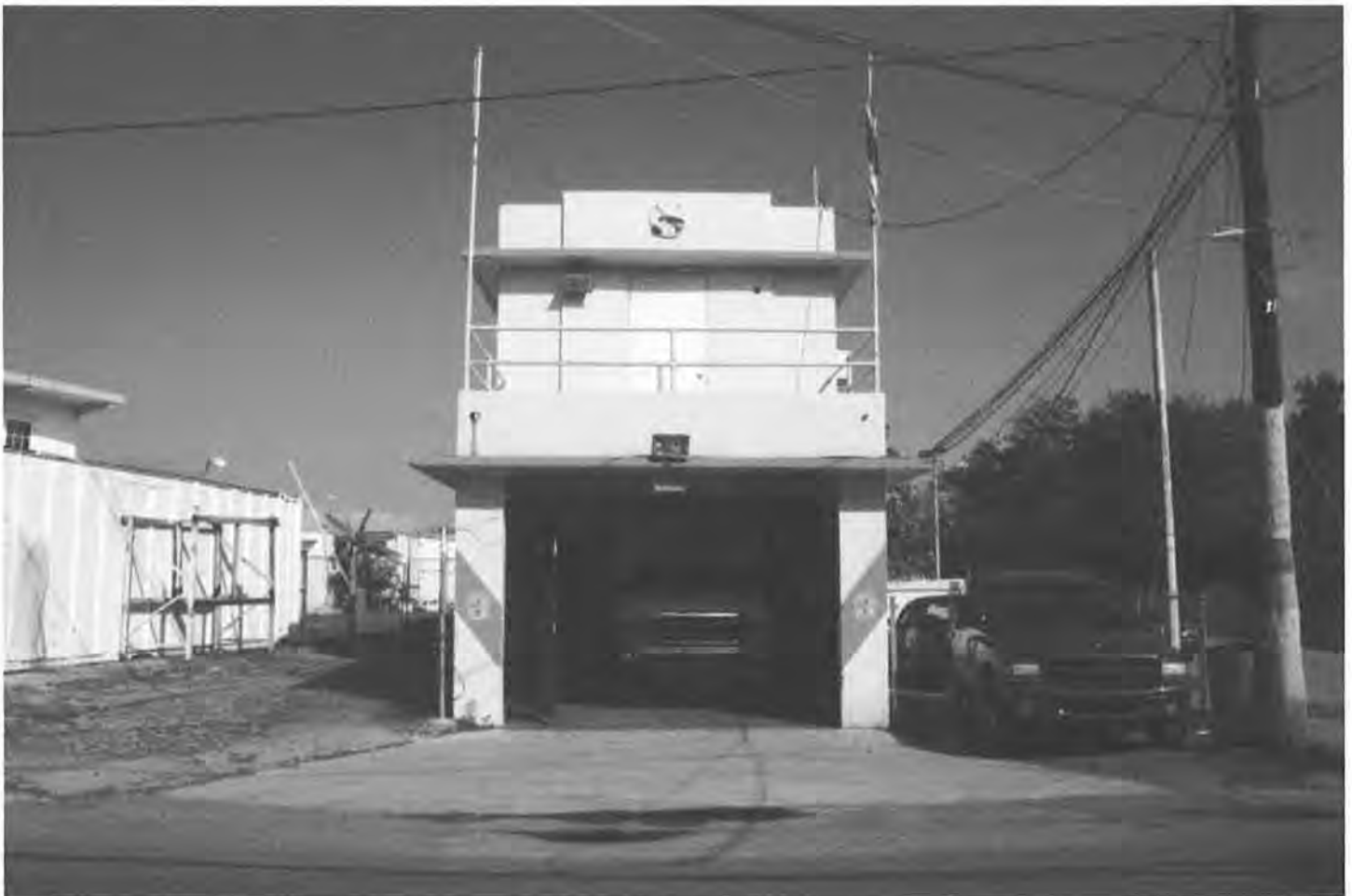
FIG. 2: Ceiba Fire Station west elevations, looking east. The main (west) façade is symmetrical in composition. The garage opening at ground floor level framed what constituted the station's foremost feature: the fire truck parked inside, facing towards the street. The straight arch entry with fillet corners is one of the few of the elements that recall the Art Deco idiom in somewhat subdued manner. Half way up the wall segments, diagonal inward painted stripes incorporate the CEM logos at center. A concrete eave projects from the lower portion of the flat arch and wraps around onto the side facades. At the second floor, the façade recedes, but also steps down in vaguely reminiscent Art Deco fashion on the uppermost profile. Today the property serves home for the State Medical Emergencies Services "Cuerpo de Emergencias Medicas Estatal (CEM)". Photo: Guillermo Marrero, February 15, 2012. Source: Jorge Rigau Arquitectos, San Juan Puerto Rico.
