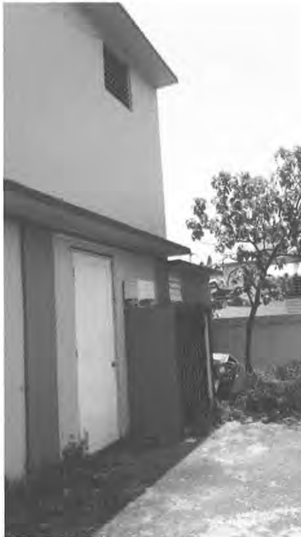
FIG. 5: Ceiba Fire Station south elevation detail looking northeast. North and south elevation share similar architectural elements, including the two wrap around concrete eaves and fenestrations. On the south façade one of the original window openings has been enlarged to accommodate an aluminum door in the 1980's. Other elements in this elevation include the meter to measure electricity, overflow pipes at roof level, some loose cables, a security lighting fixture and gas tank storage closet. Photo: Guillermo Marrero, February 15, 2012. Source: Jorge Rigau Arquitectos, San Juan Puerto Rico.
