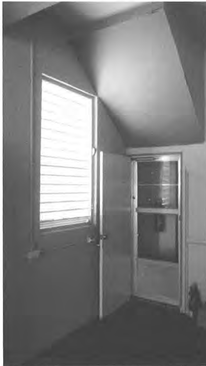
FIG. 6: Ceiba Fire Station interior view, looking east. A one level annex was added that is accessed through the storage space adjacent to the the stairs. The added volumes, clearly a plug-in solution to provide additional space, provide now for a mixed use office/resting/dispatch area including a small bathroom. Photo: Guillermo Marrero, June 10, 2012. Source: Jorge Rigau Arquitectos, San Juan Puerto Rico.
