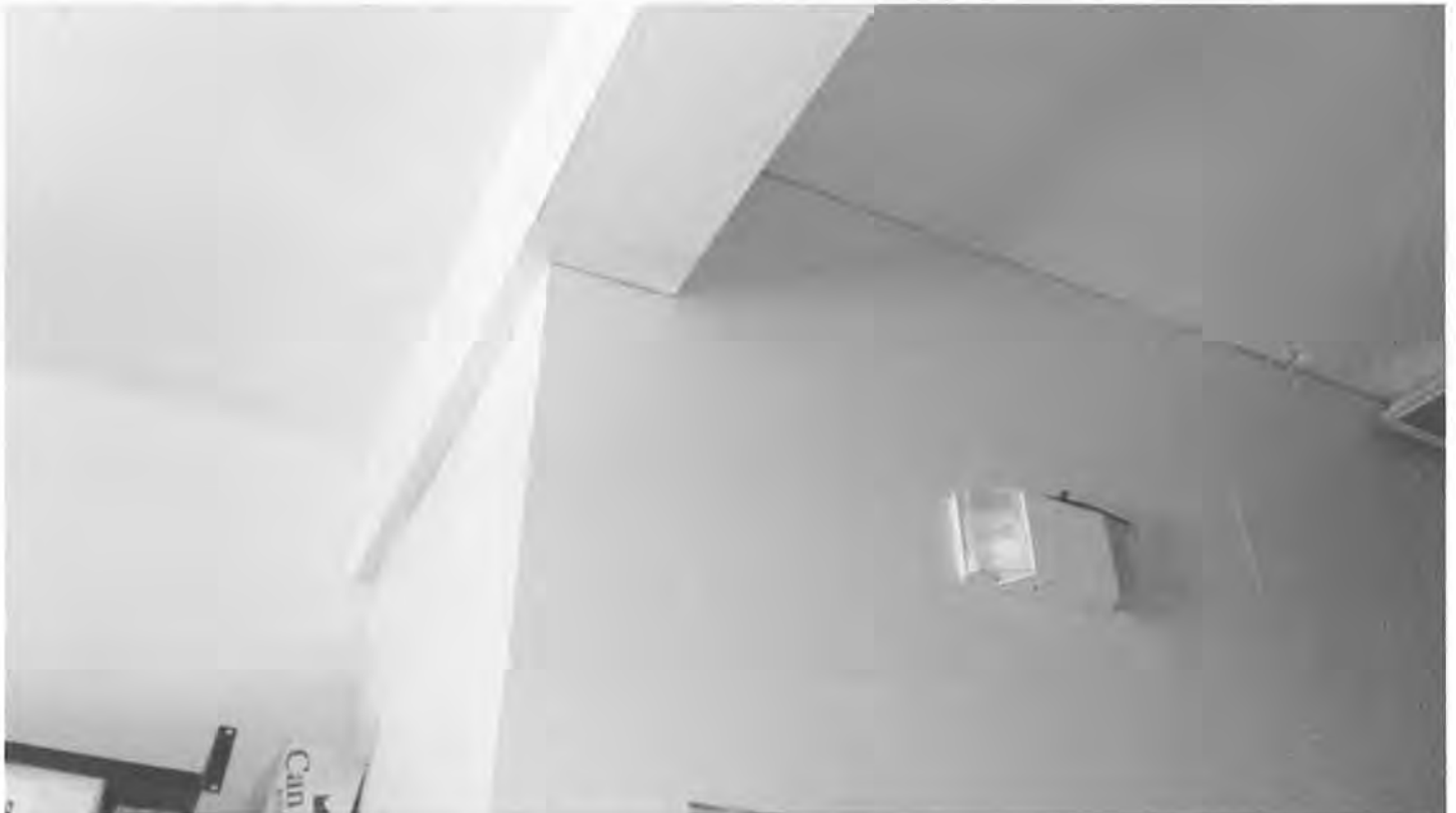
FIG. 8: Ceiba Fire Station interior detail view. On the second floor the hand rail height parapet of the stairs was closed off and another door was added in front of the restroom. A new window was added to the back façade to provide natural light to enter the enclosed stairwell. The original second floor bathroom was enlarged to accommodate a new shower area. Photo: Guillermo Marrero, February 15, 2012. Source: Jorge Rigau Arquitectos, San Juan Puerto Rico.
