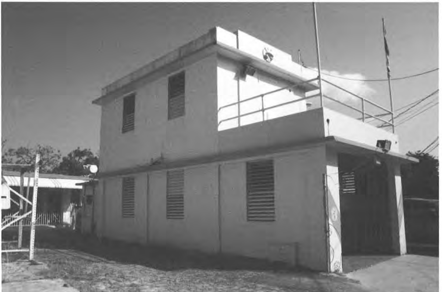
FIG. 4: Ceiba Fire Station north and west elevations, looking southeast. The fire station's emblematic presence is further established by its object-like nature. From the northwest, the building appears clearly as a freestanding volume within the surrounding urban milieu. Photo: Guillermo Marrero, February 15, 2012. Source: Jorge Rigau Arquitectos, San Juan Puerto Rico.
