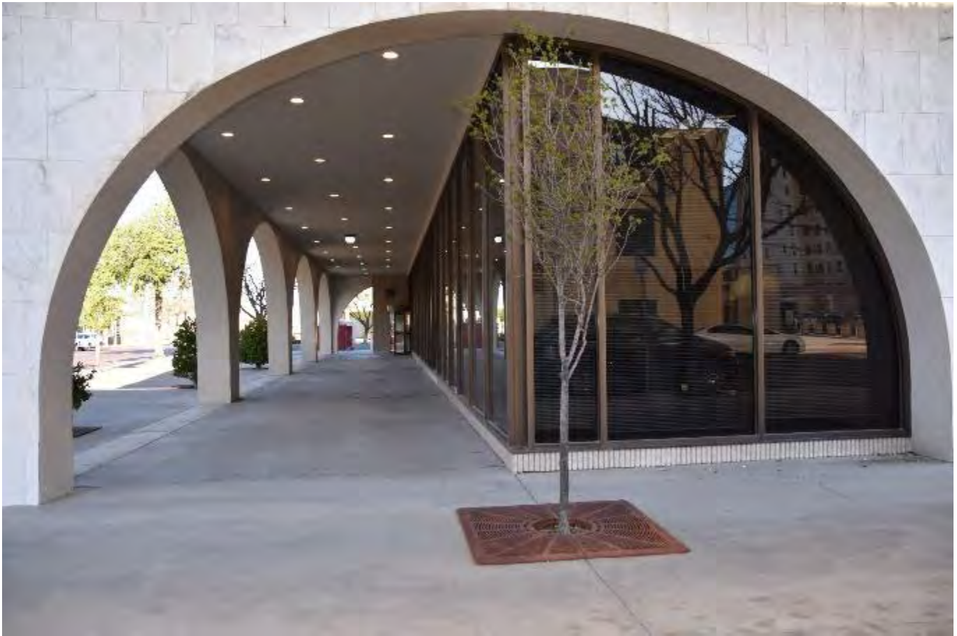
Photo 7 Ground floor arcade Camera facing west
