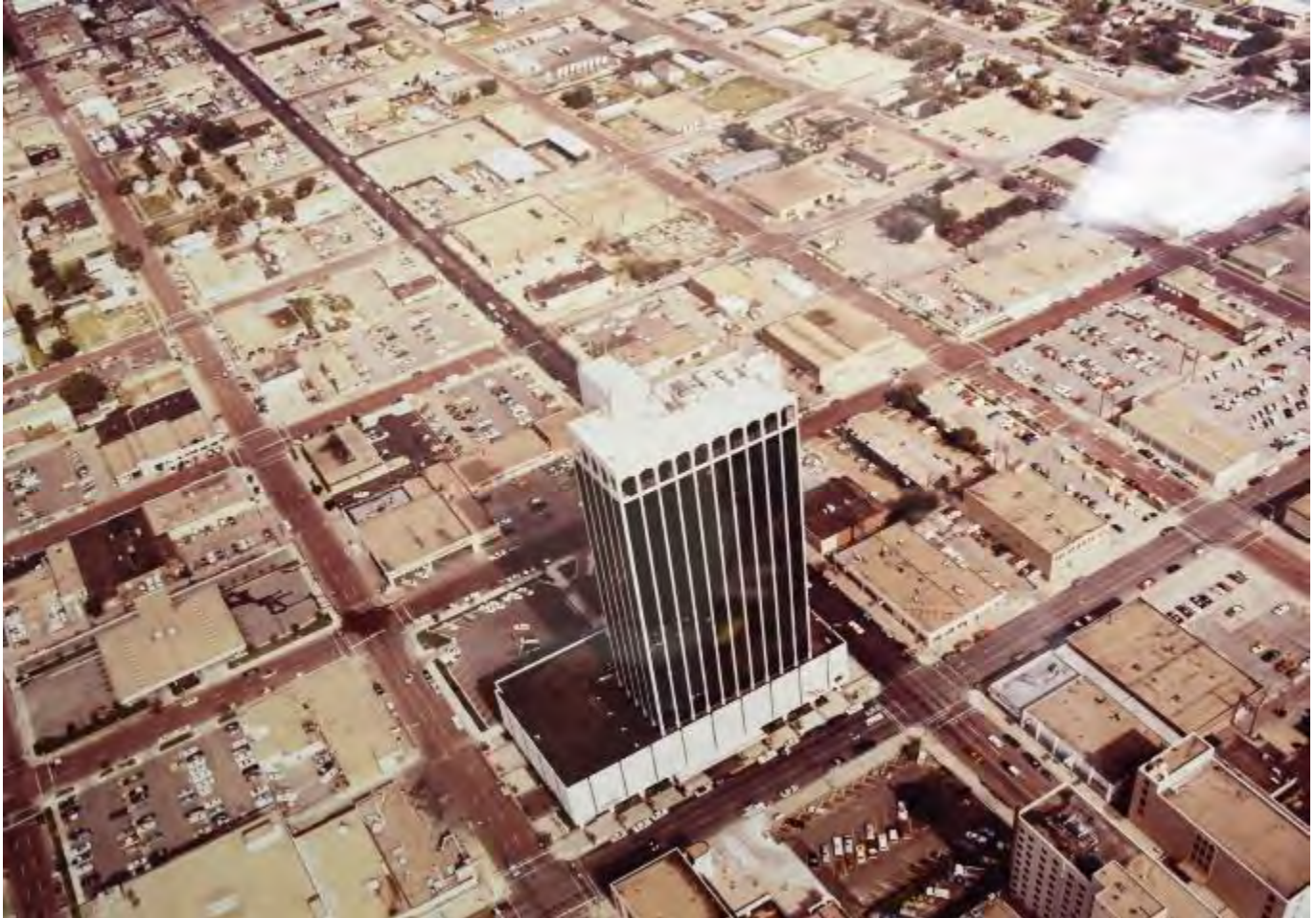
Figure 4: American National Bank Building and SPS Tower Aerial, facing west c. 1970 Source: Building Owner
