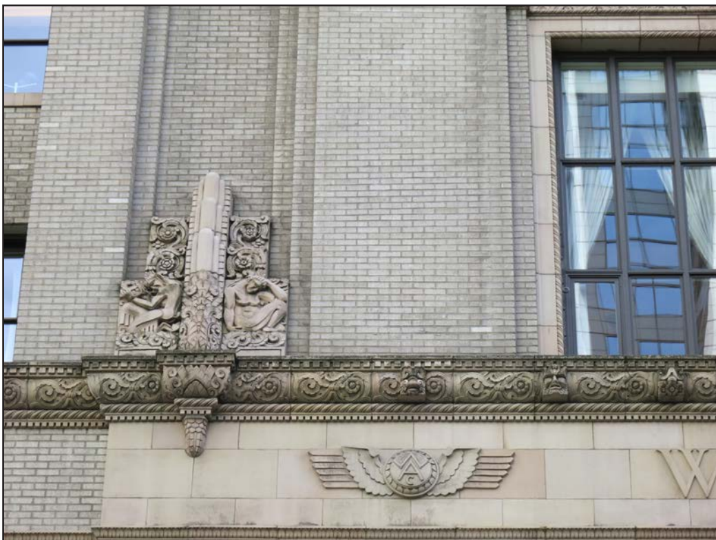
0020. North facade decorative elements and details; looking south.
