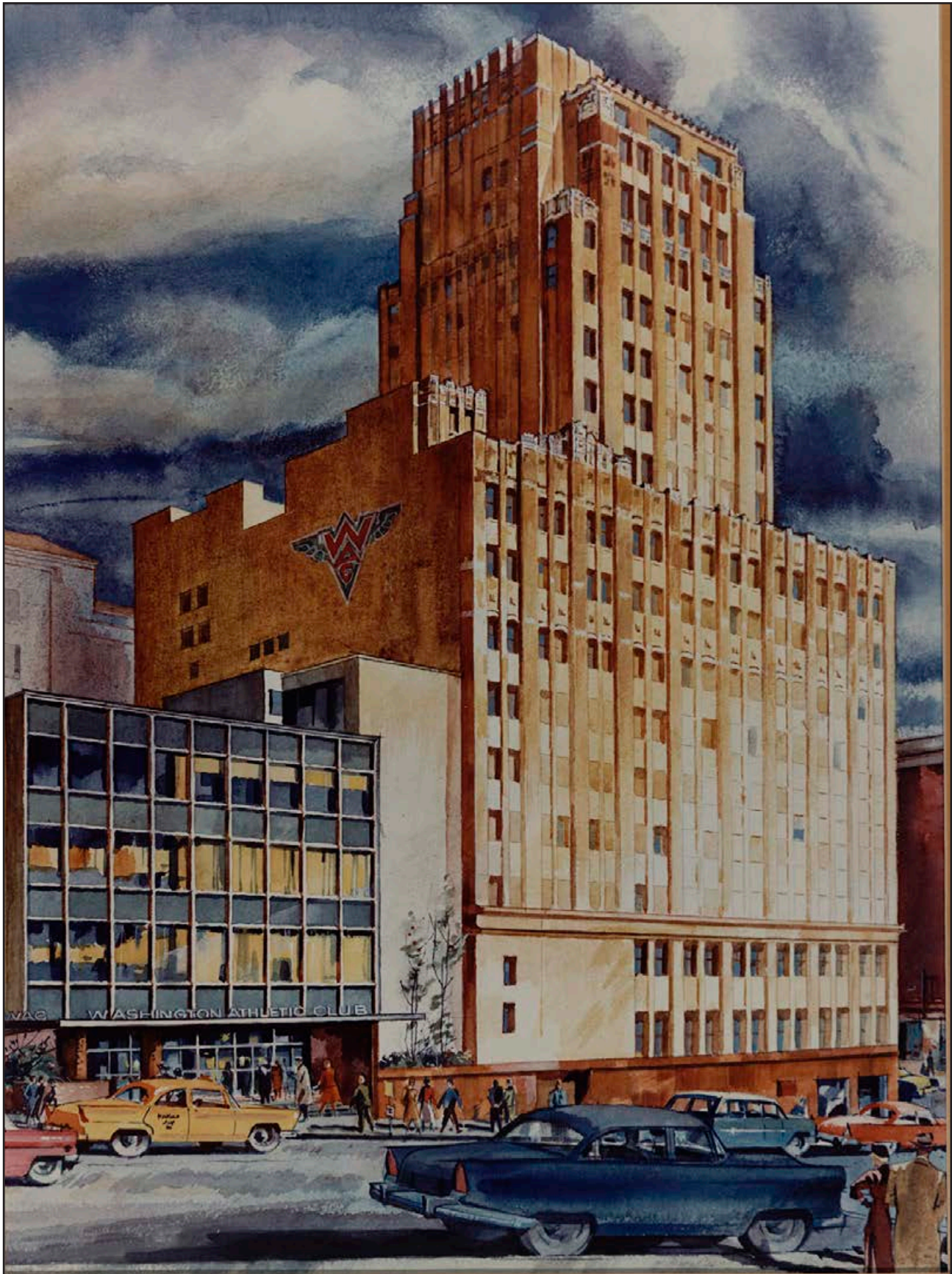
Ca. 1954 artist rendering of the Washington Athletic Club building with four-story, modern addition to the south. Source: Washington Athletic Club
