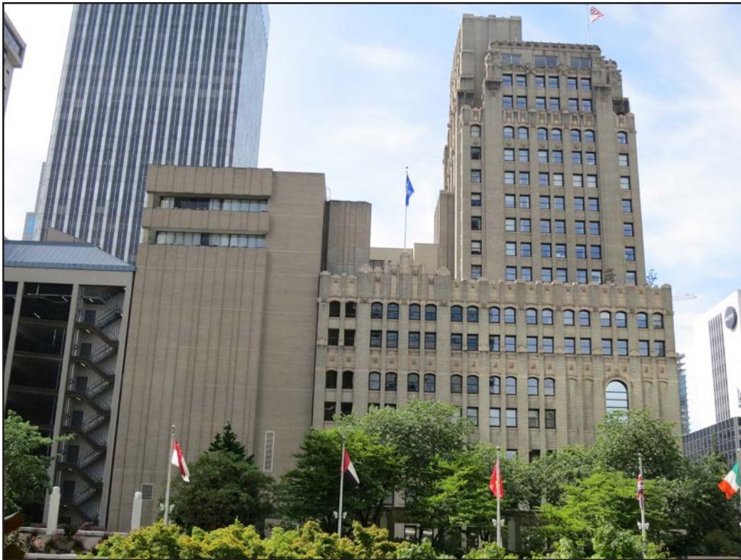
0007. East facade, looking west. Original 1930 building on right; 1970 addition on left.
