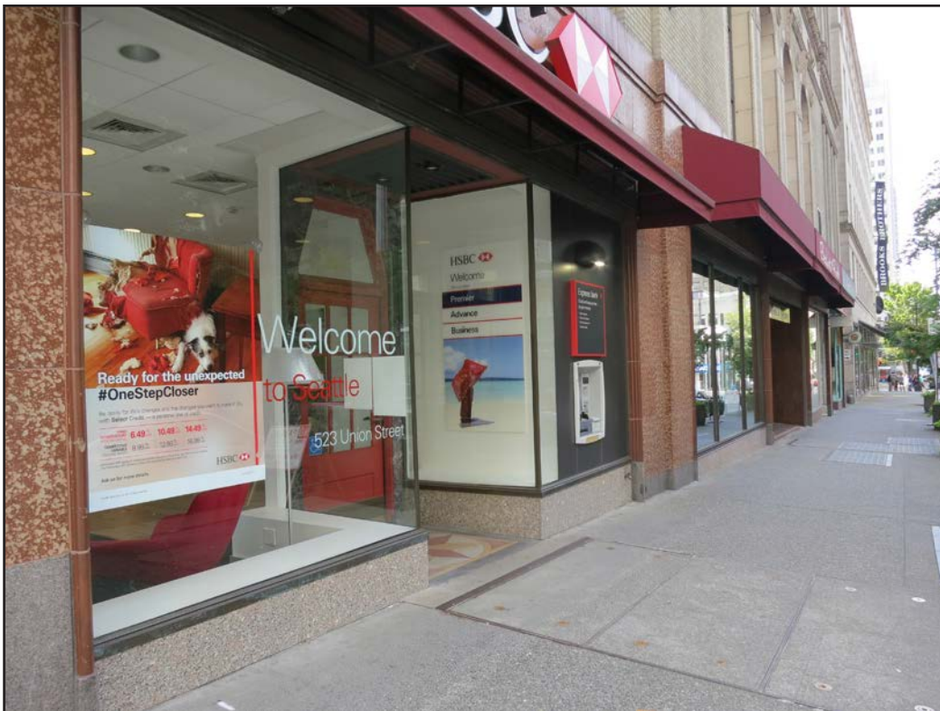
0015. North facade and retail storefronts, looking west.
