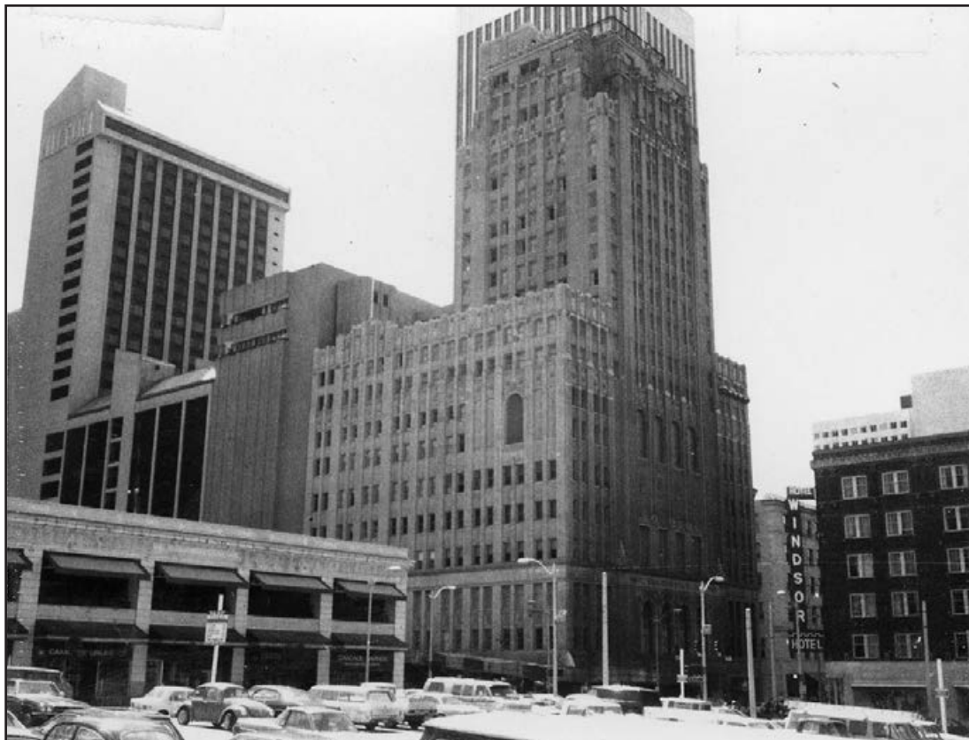
King County Tax Assessor photographs for Washington Athletic Club. Top left: 1970, addition under construction; top right and bottom: 1990. Source: Washington State Archives, Puget Sound Region Branch
