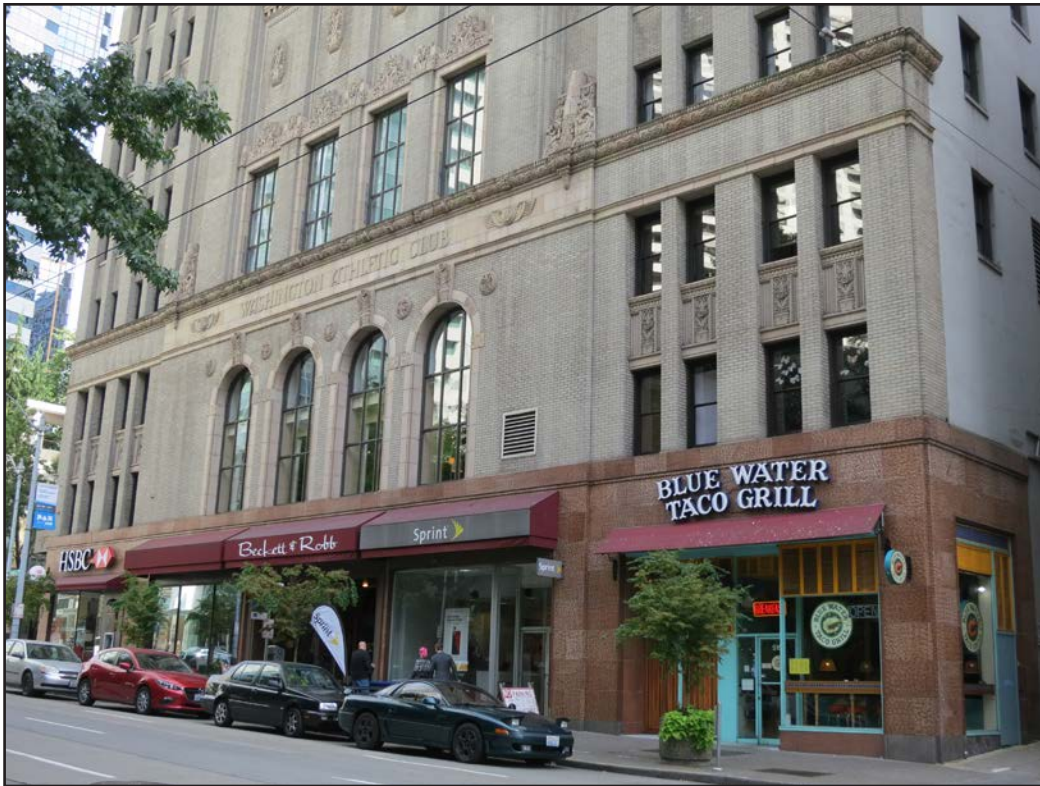
0013. North facade and retail storefronts, looking southeast.
