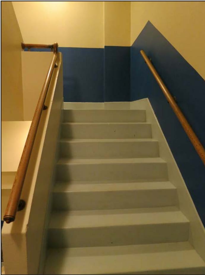
0051. Interior, stairs (typical) on hotel floors (10-20).
