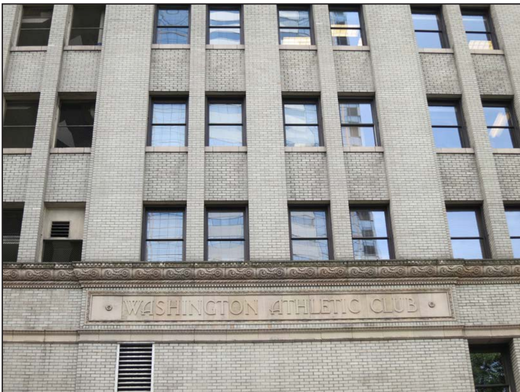
0018. East facade windows, decorative elements, building name; looking west.
