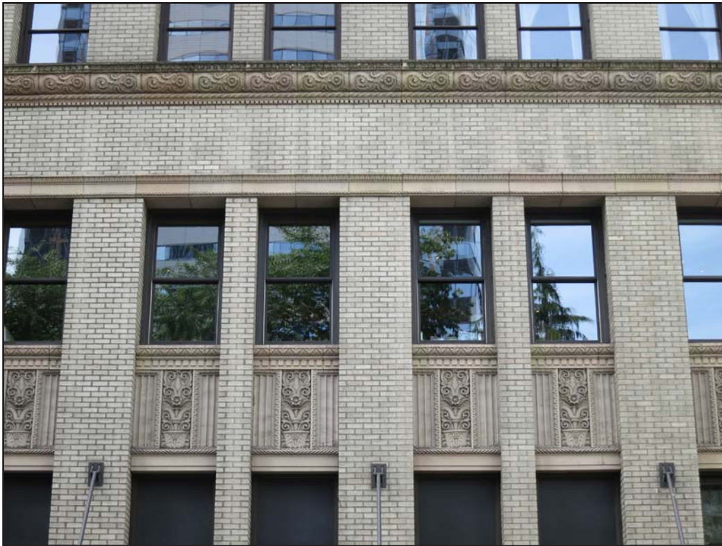
0019. East facade windows and decorative elements; looking west.
