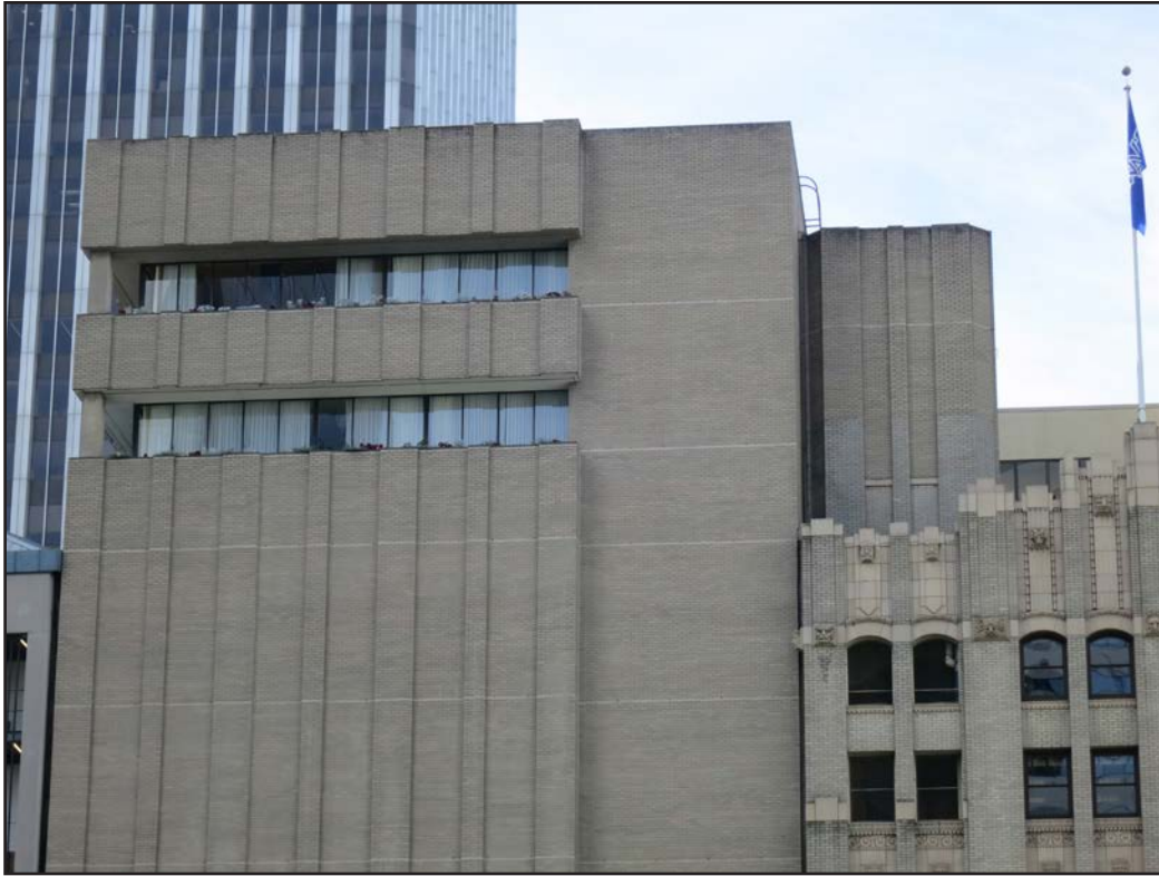
0021. East facade of 1970 addition and partial east facade of original 1930 building, looking west.
