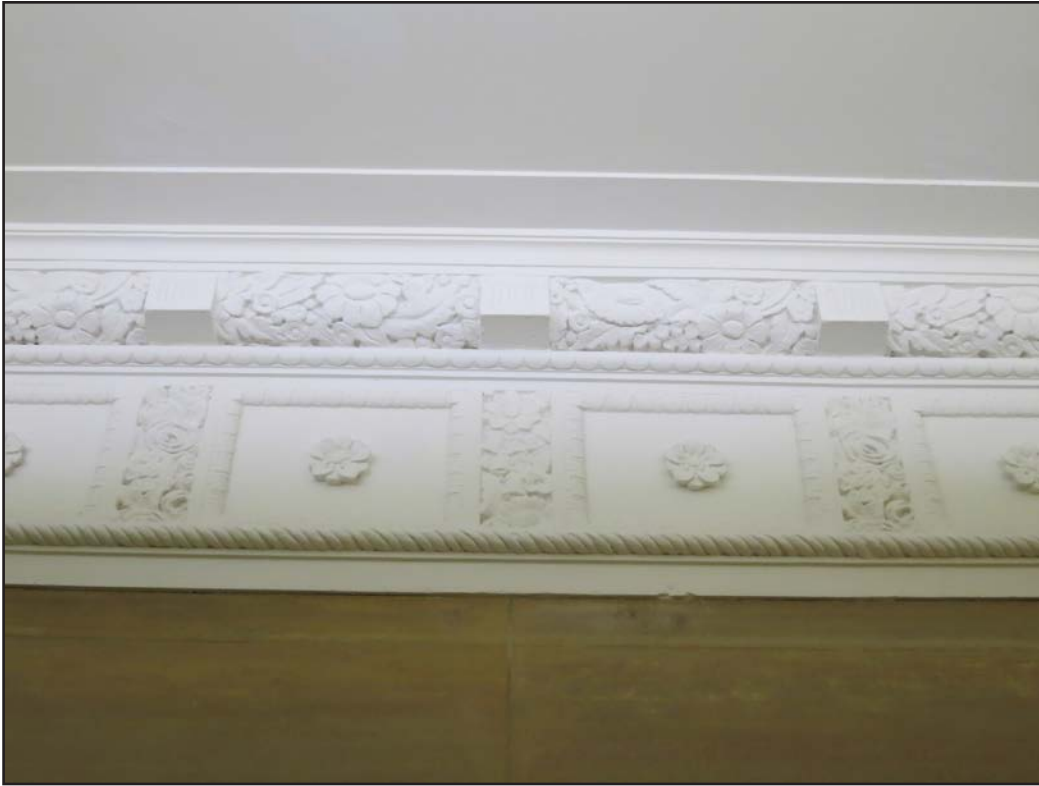
0027. Interior, first floor lobby - original decorative molding above elevators.
