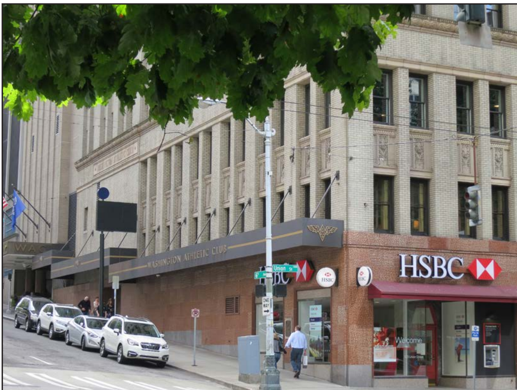
0012. East facade and partial north facade, looking southwest.
