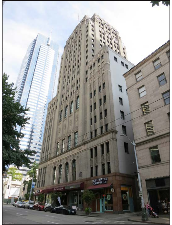
0004. North facade and partial west facade, looking southeast.
