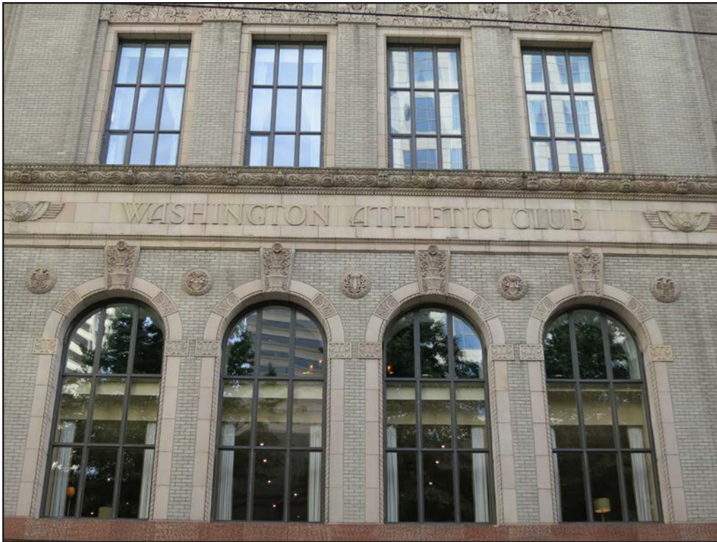
0017. North facade windows, decorative elements, building name; looking south.
