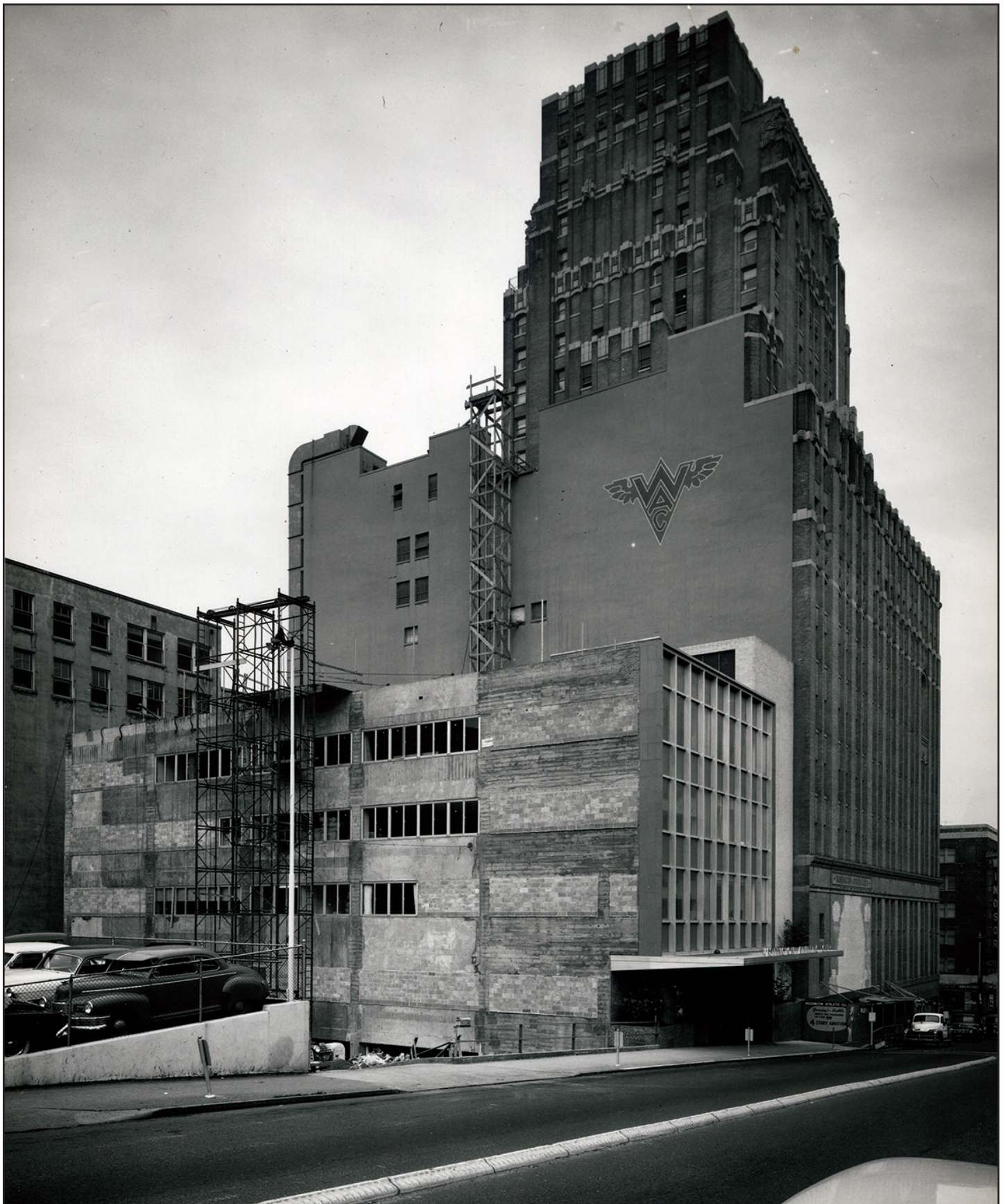
1955. Four-story addition under construction. Source: WAC
