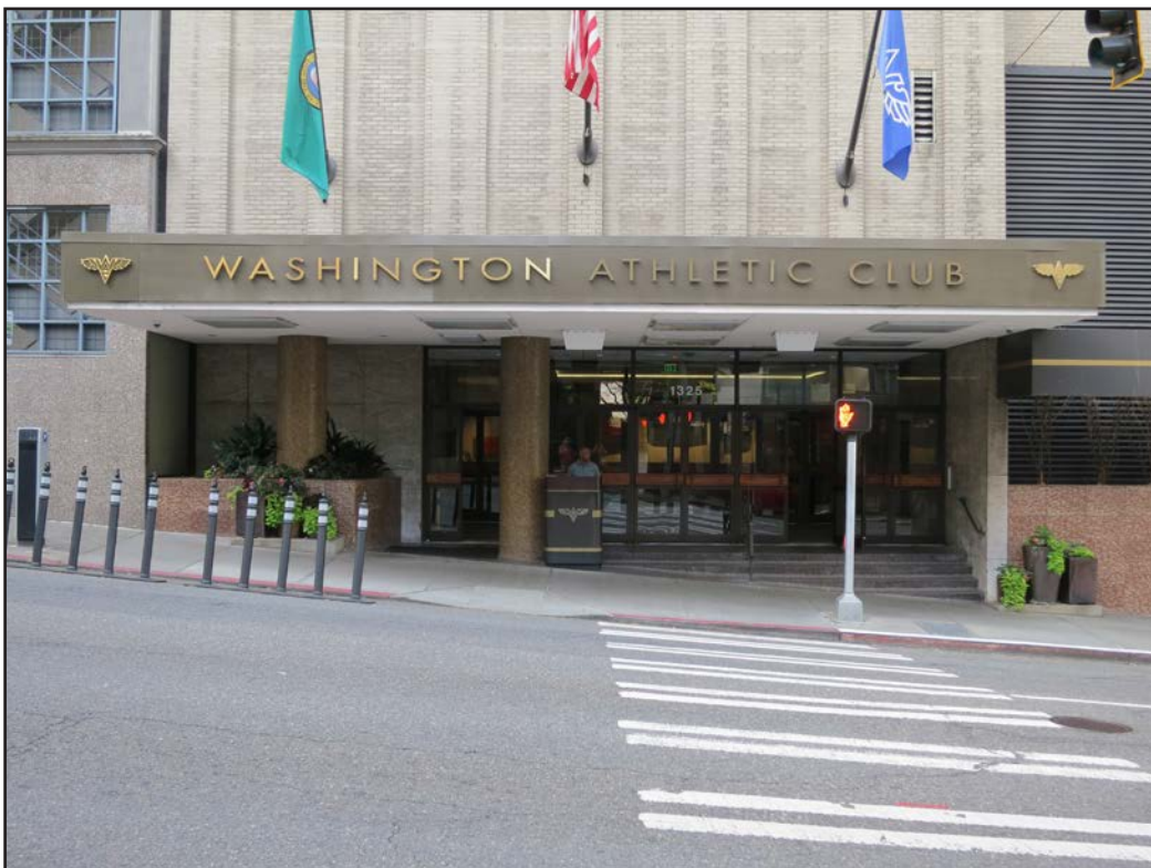
0010. East facade of 1955/1970 addition, looking west. Main entrance to the WAC.
