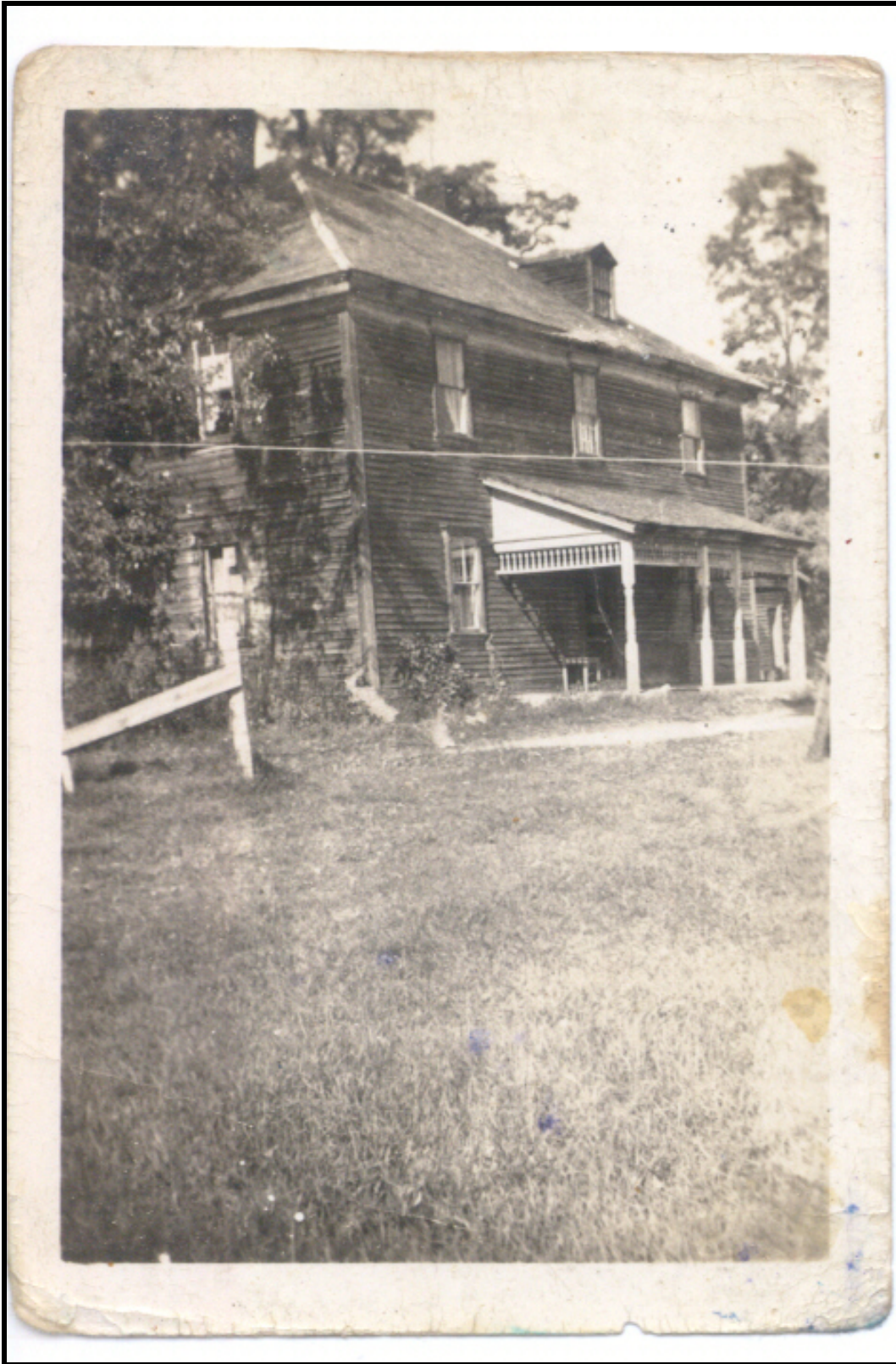
ABOVE, Martin-Fitch house, 1943, view showing south and east (rear) elevations
