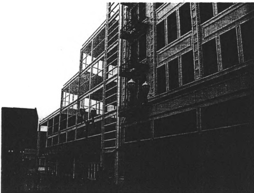
Figure i. Twohy Building, San José, CA
