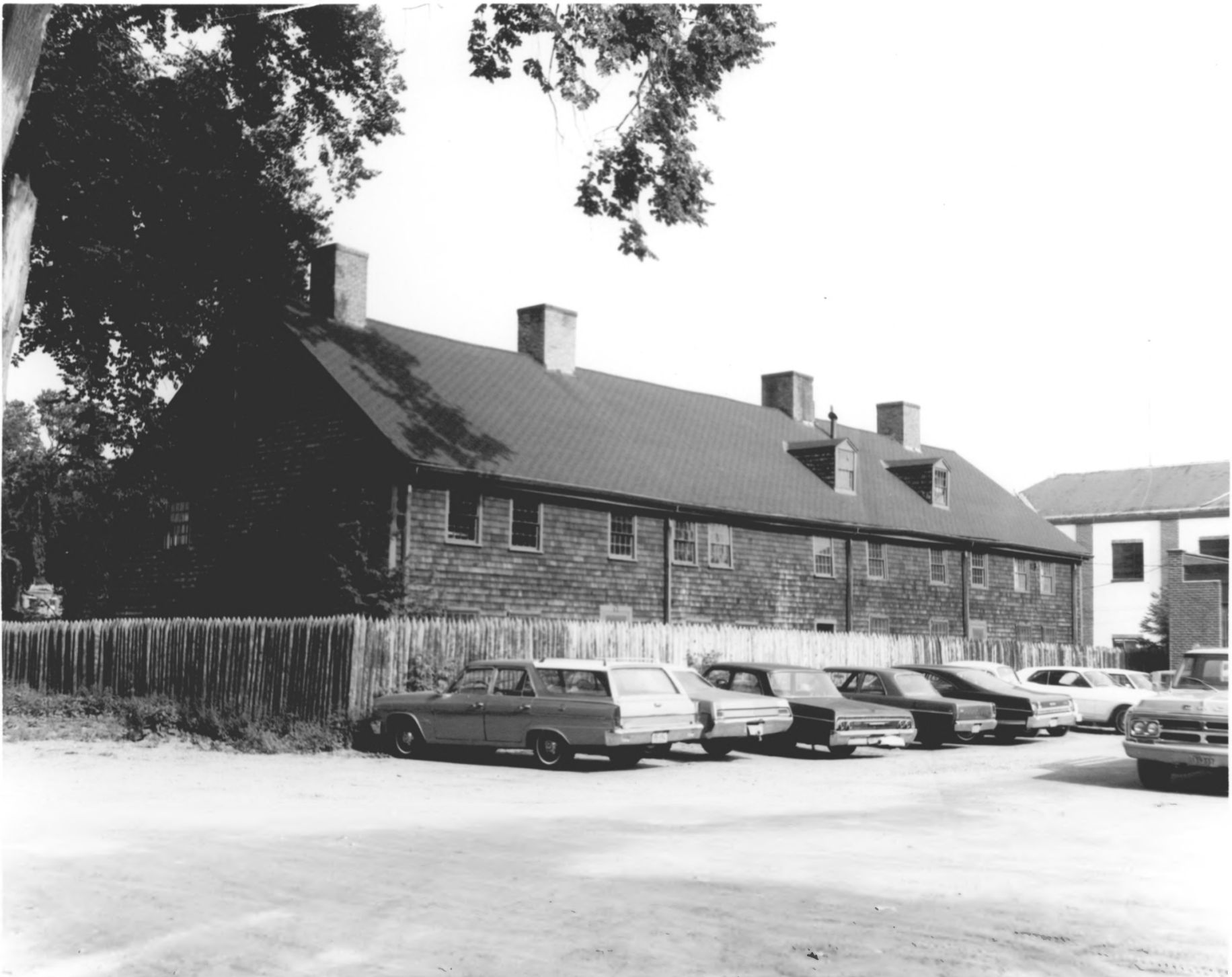
Fort Western, Augusta, Maine Rear elevation.
