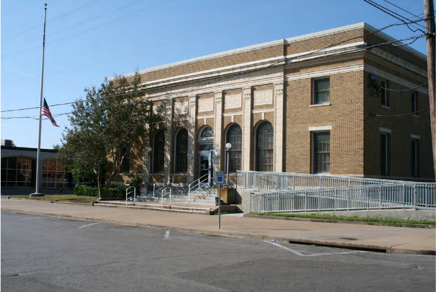
Photo 1: Resource #84, Ennis Post Office, 205 N. McKinney St. Camera facing SW.
