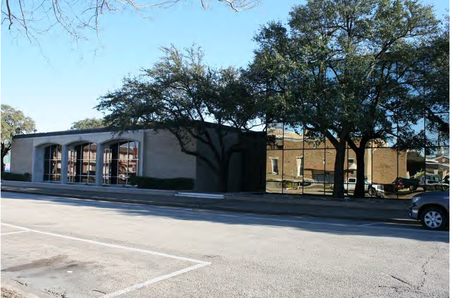
Photo 3: Resource #86, Citizens National Bank Building (Bank of America), 301 W. Knox St (left) and addition (right). Camera facing SE.
