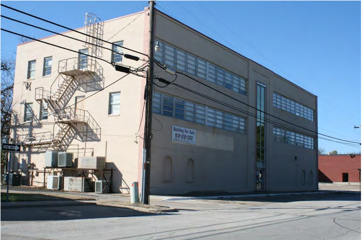
Photo 6: Resource #88, Texas Fire Insurance Company/Ennis Business Forms Building, 107 N. Sherman St. Camera facing NW.
