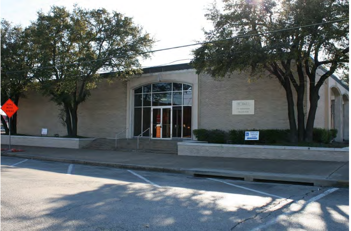
Photo 4: Resource #86, Citizens National Bank Building (Bank of America), east elevation, 301 W. Knox St. Camera facing SW.
