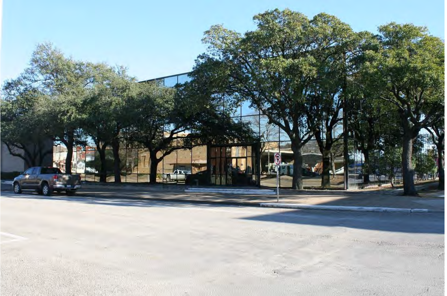
Photo 5: Resource #86, Citizens National Bank Building (Bank of America) addition, 303 W. Knox St. Camera facing SE.
