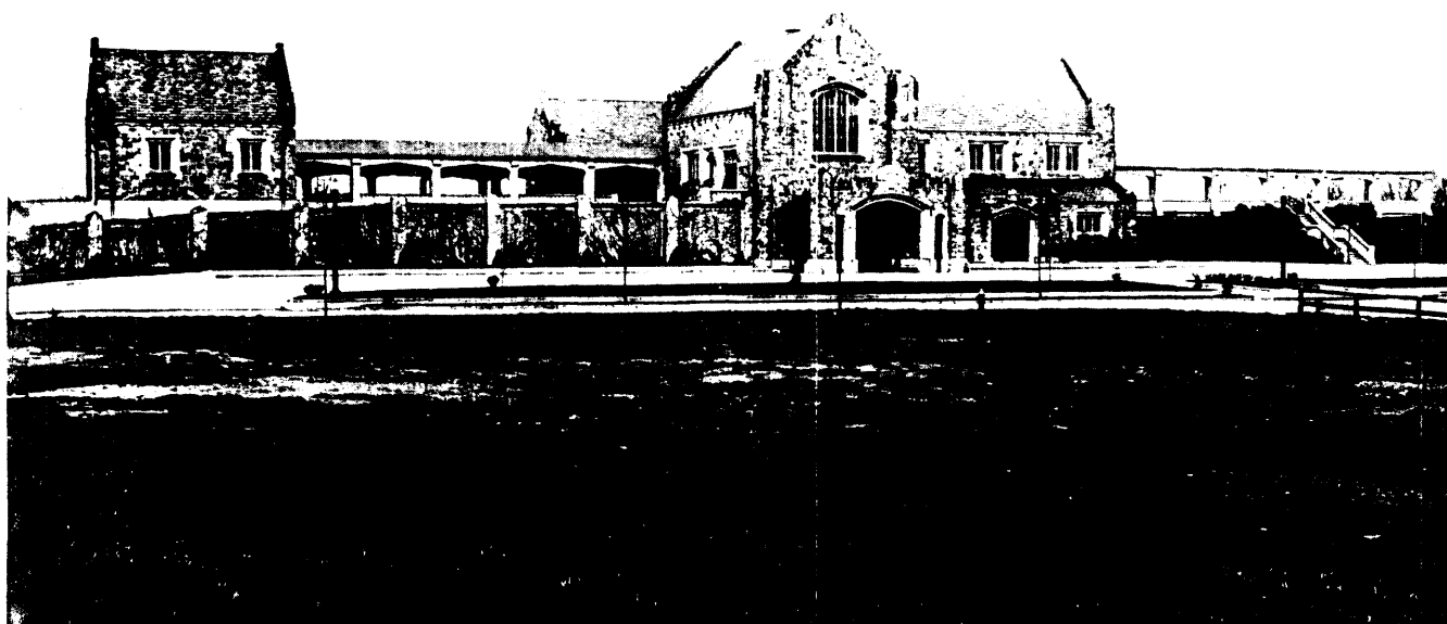
The new Madison station was opened April 17, 1916. The building at the left housed the Railway Express office. Prior to the elevation, the area in the foreground was thickly covered with homes, all of which were removed for the station. In 1976 the station was declared a historic site.
