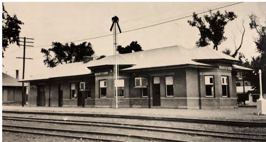
Figure 10: The AT&SF passenger depots in Garden City, Kansas, (top) Las Animas, Colorado, (5BN.415) (middle) and Rocky Ford, Colorado, (5OT.190) (bottom), followed the same standardized design as the Lamar depot with some minor variations. (Source: Pounds, Santa Fe Depots, the Western Lines /Finney County Historical Society/John McCall Collection/Frank O. Kelley Collection)
