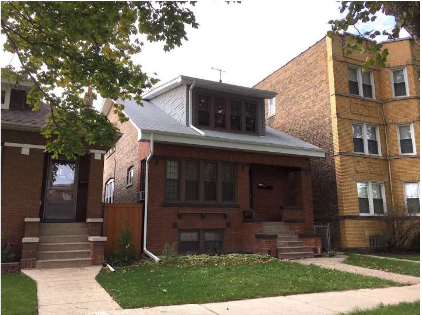
IMAGE 18: An example of a bungalow with a less common side-gable roof at 3052 N. Kenneth.
