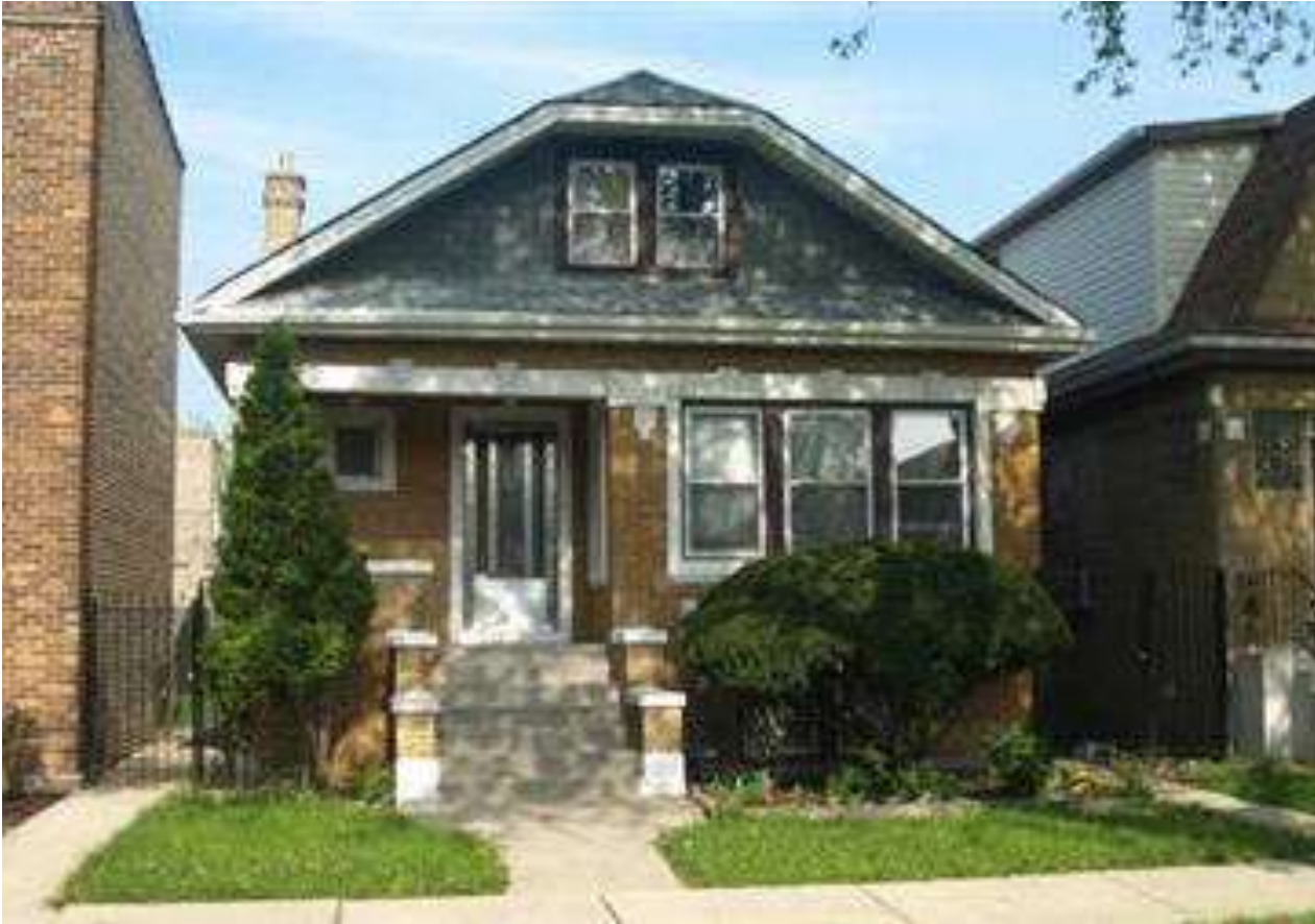
IMAGE 5: An example of a frame gabled roof with a clipped peak at 2851 N. Kostner.
