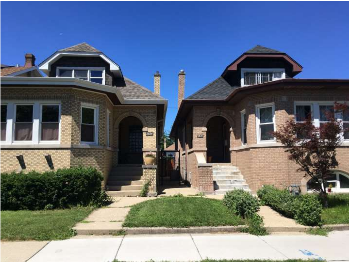
IMAGE 7: Five-sided polygonal bays on the 2800 block of N. Kostner.
