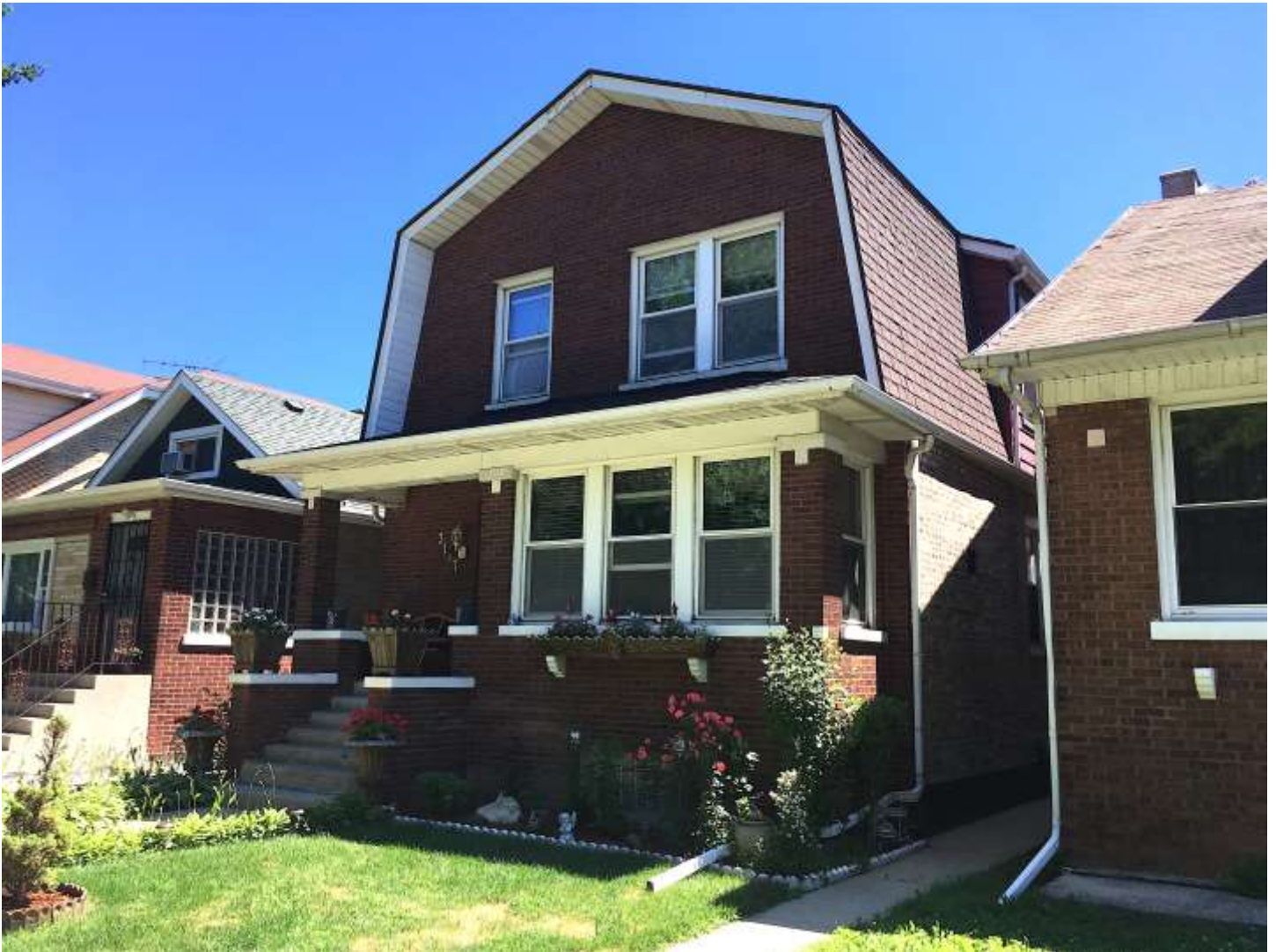
IMAGE 16: Example of a contributing true gable front, which is an extension of the brick façade, at 3117 N. Kolmar.
