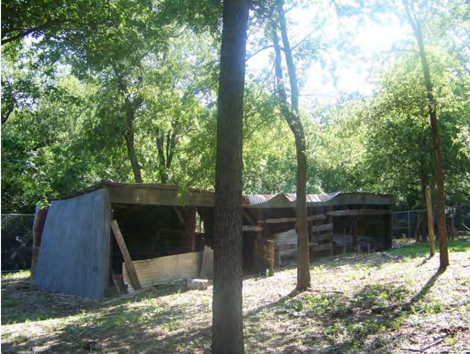
TX_Dallas County_ Everard Sharrock Jr. Farmstead_0010.tif Chicken Coop (noncontributing) Southwest Oblique. Camera facing: Northeast
