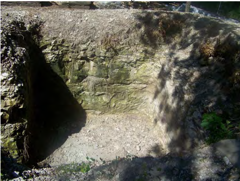
TX_Dallas County_Everard Sharrock Jr. Farmstead_0007.tif Root Cellar Interior View. Camera facing: Northwest
