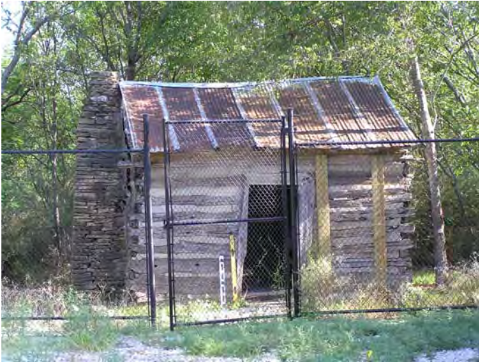
Figure 3 - Log cabin with reinforcement, August 2007
