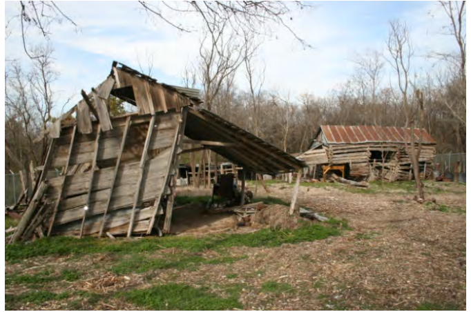
Figure 15 - Plank barn, February 2008
