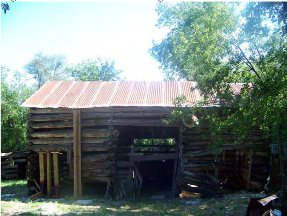
TX_Dallas County_ Everard Sharrock Jr. Farmstead_0003.tif Log Barn South Elevation. Camera facing: North
