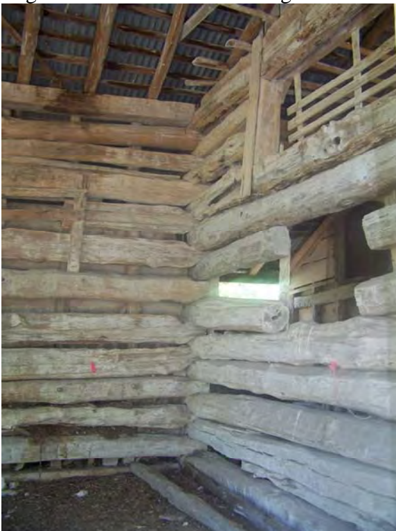
TX_Dallas County_ Everard Sharrock Jr. Farmstead_0005.tif Log Barn Interior View showing 'crib door'. Camera facing: Northeast
