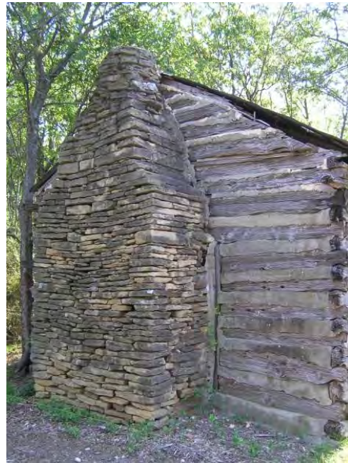
Figure 4 - Log cabin stone chimney, August 2007
