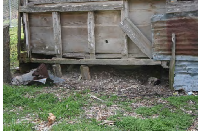
Figure 9 - Log barn – details of crib with bois d’Arc piers, February 2008
