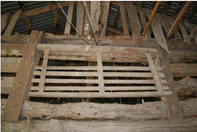
Figure 10 - Crib door in upper wall of log barn, May
