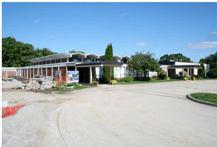
View of the primary elevation.
