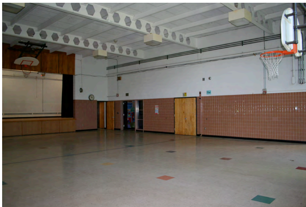
Figure 16. (Image 0023) Monroe Elementary, Section A, Multi-Purpose Space – 2014
