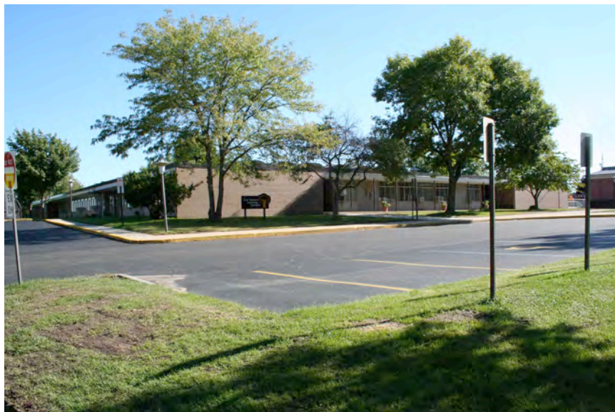
View of the primary elevation.
