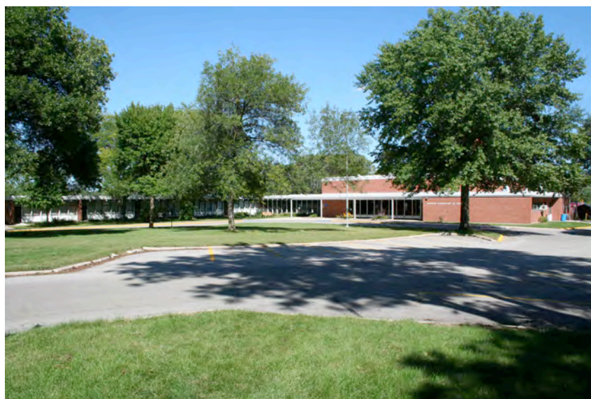
View of the primary elevation.
