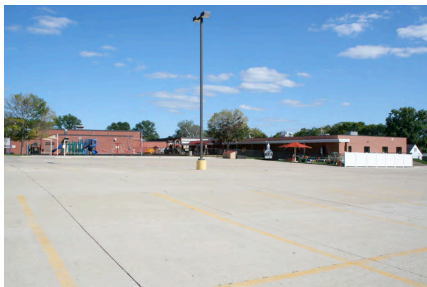
View of the rear elevations.
