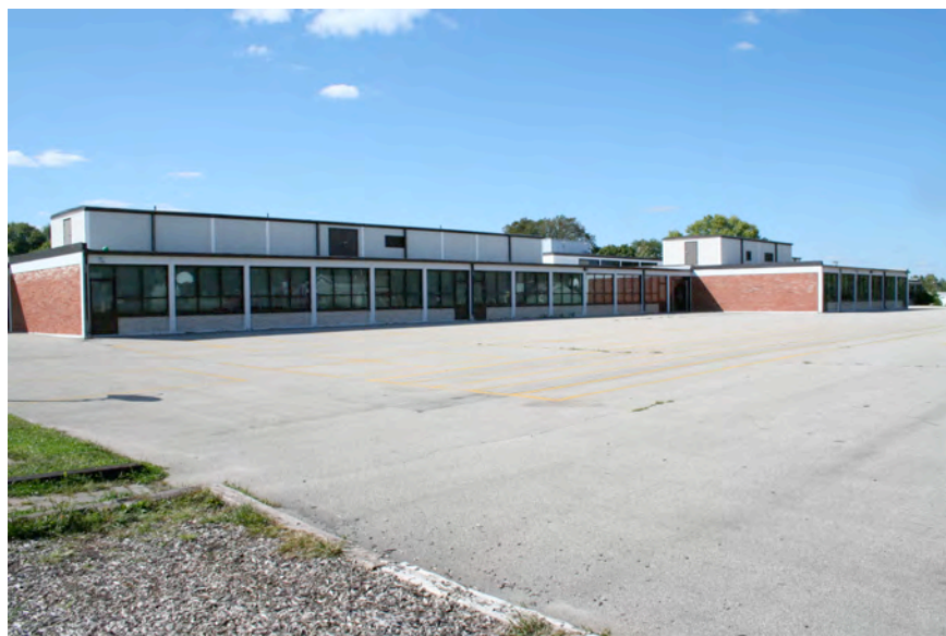
View of the rear elevation with classrooms.
