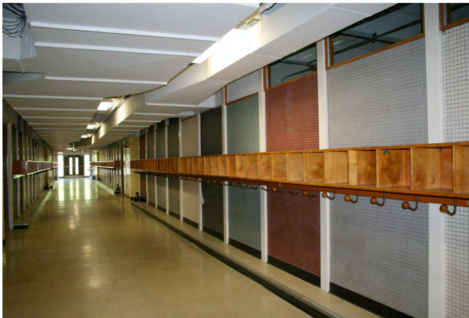
Figure 22. (Image 0019) Monroe Elementary, Typical Hallway – 2014
