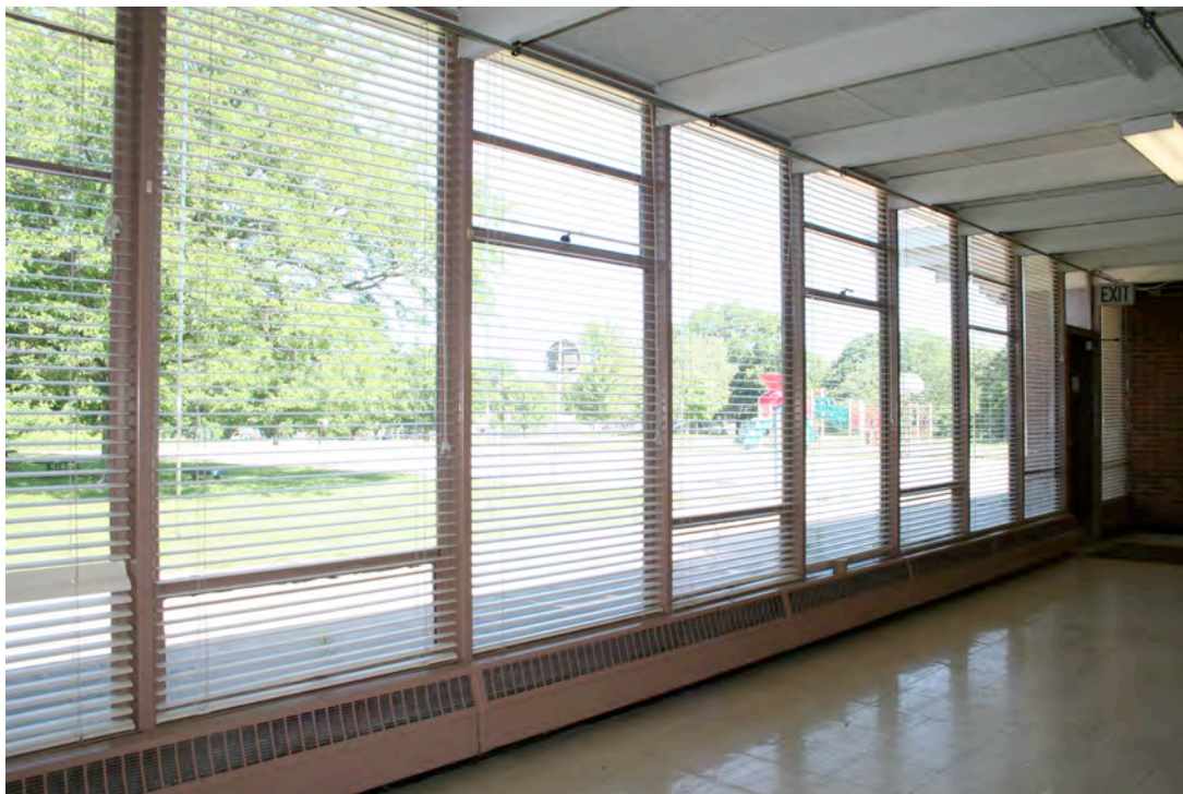
Figure 13. (Image 0018) Monroe Elementary, Typical Windows – 2014
