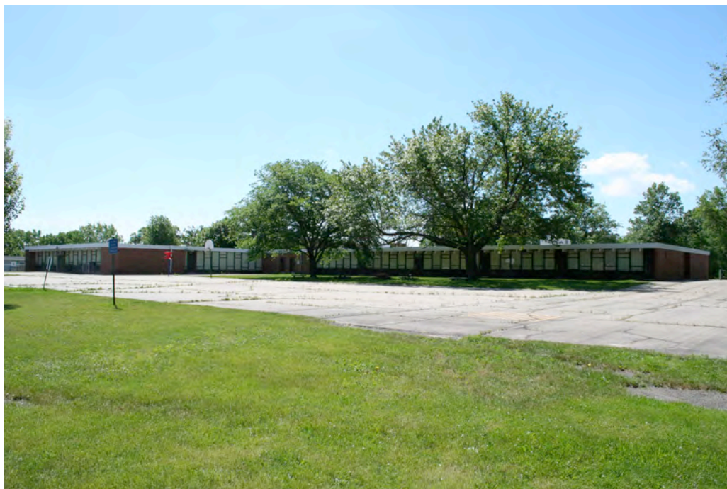
Figure 9. (Image 0010) Monroe Elementary, Rear (North) Elevation – 2014
