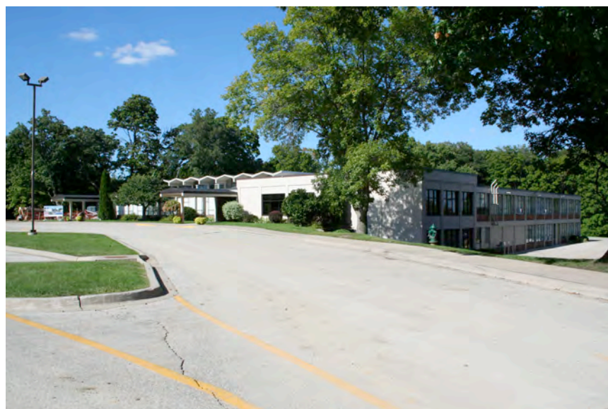
View of the primary elevation and secondary elevations.
