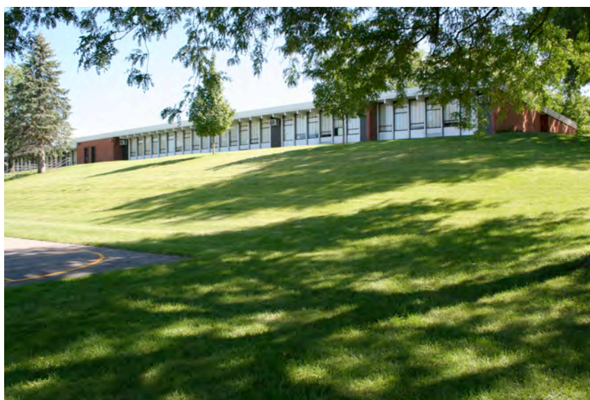
View of the classroom wing showing fenestration that is the same as used for Monroe Elementary.
