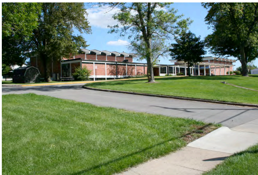
View of the primary elevation.
