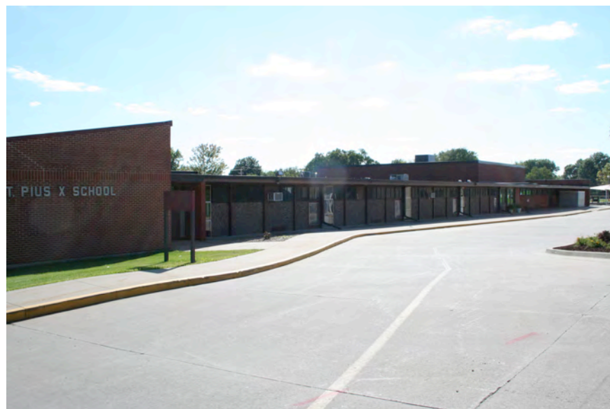
View of the primary elevation.
