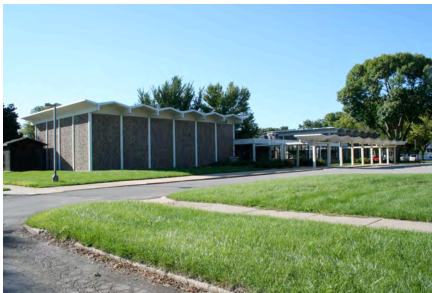
View of the primary elevation.
