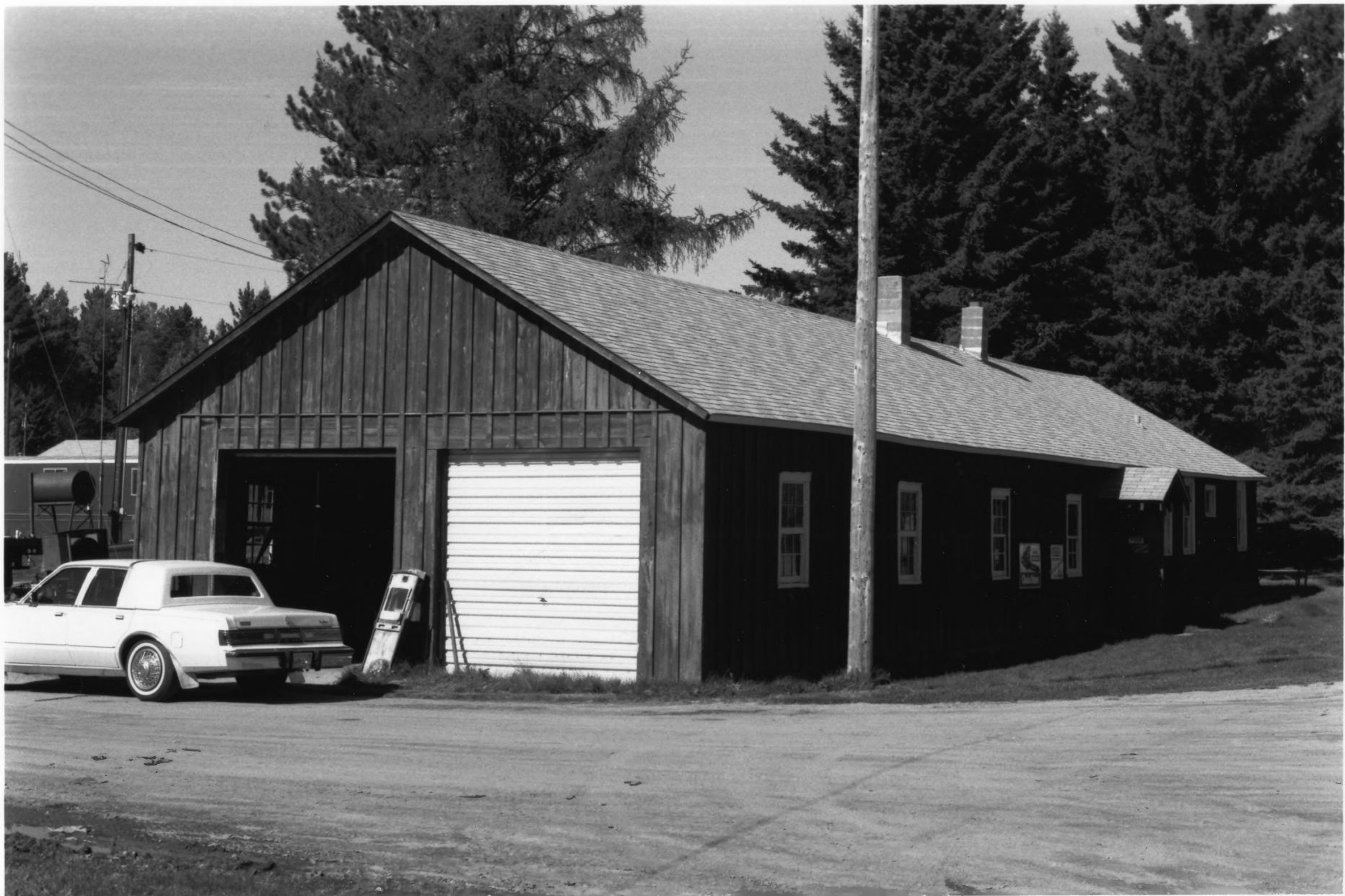
Civilian Conservation Corps Camp 5-52 St. Louis Co., MN 09338/17
