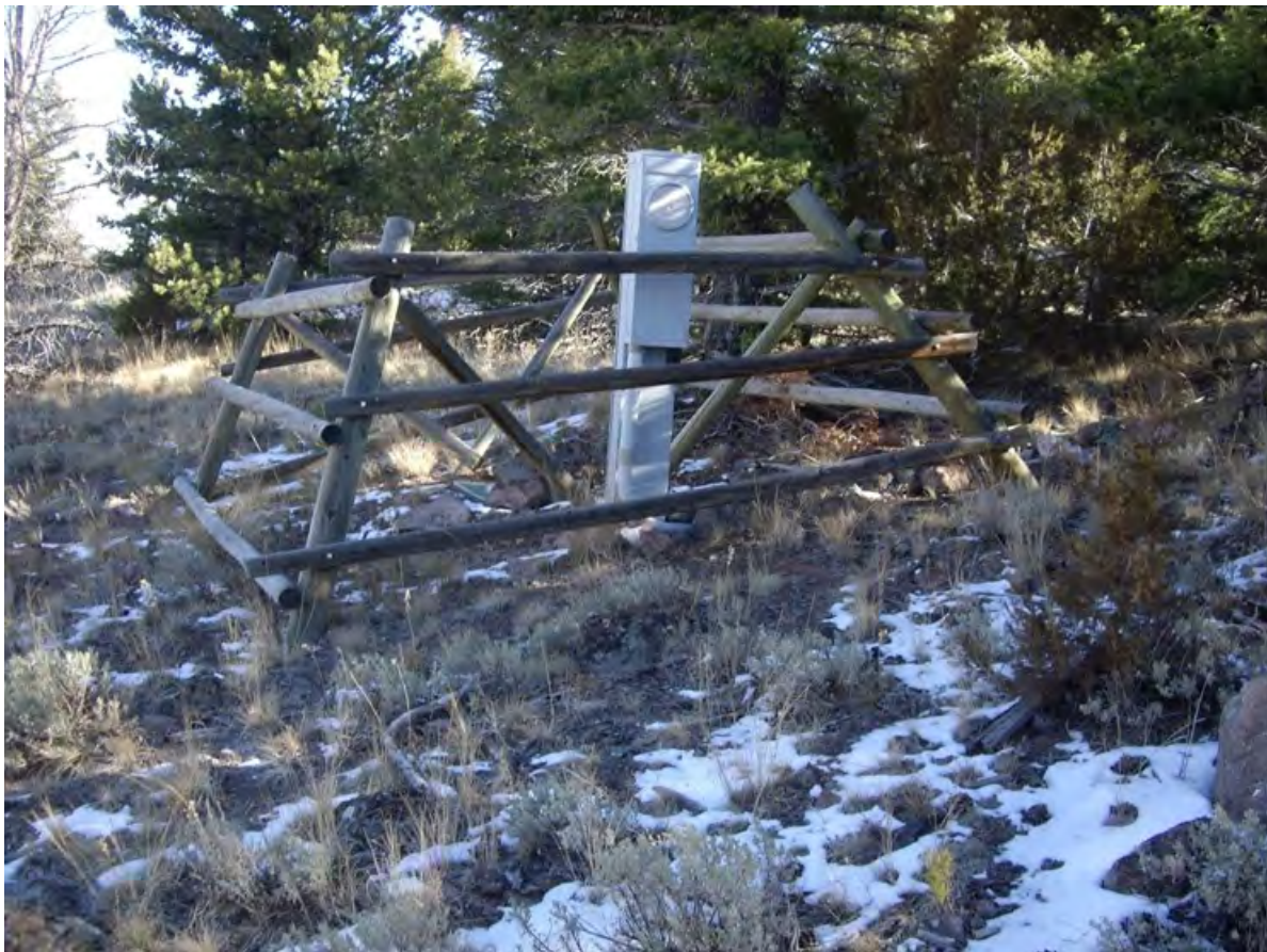
MT_BeaverheadCounty_CanyonResortAirwayBeacon_0010: Electric Vault Box. View to the northeast.
