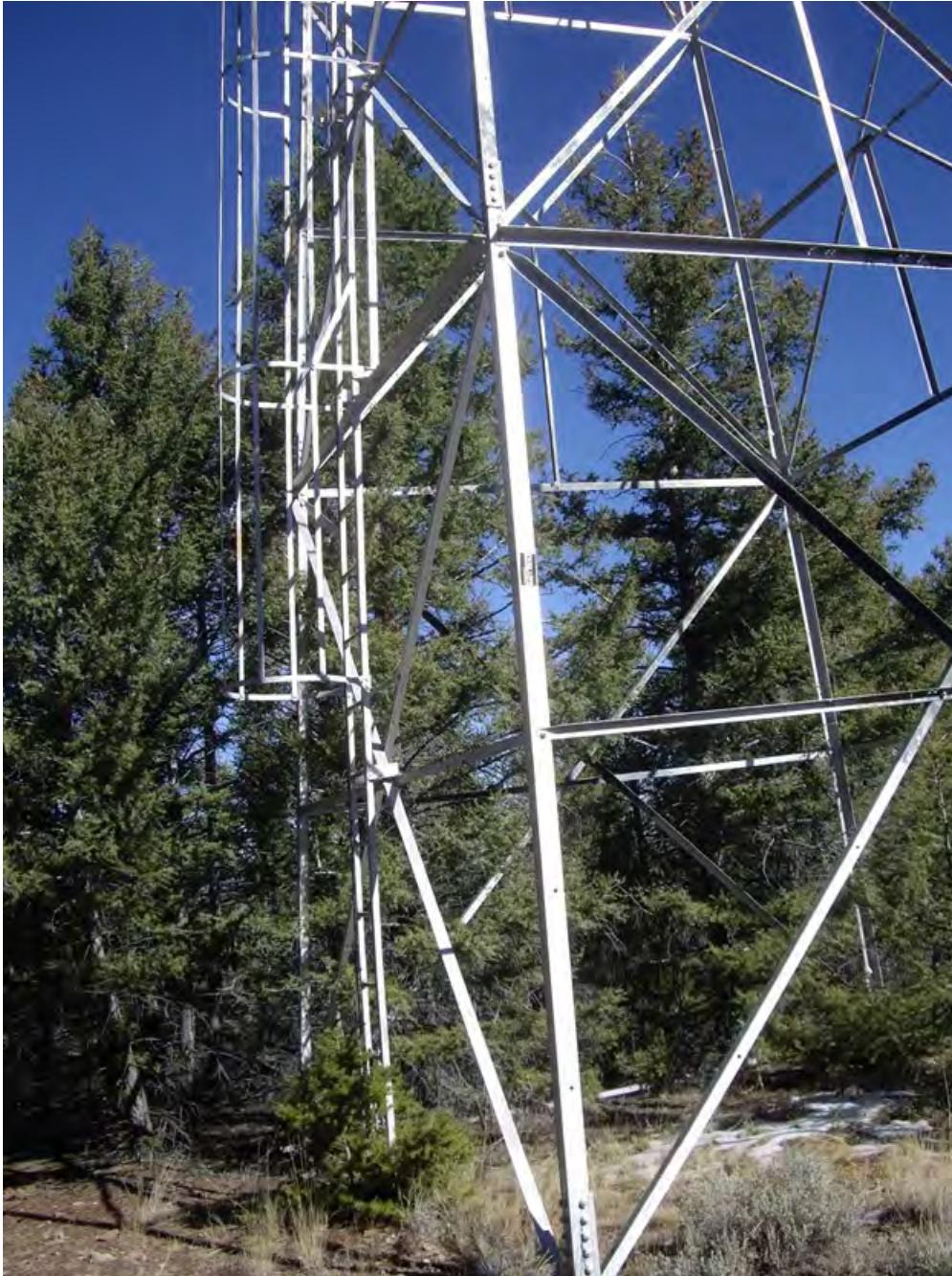
MT_BeaverheadCounty_CanyonResortAirwayBeacon_0007: Tower base. View to the North.
