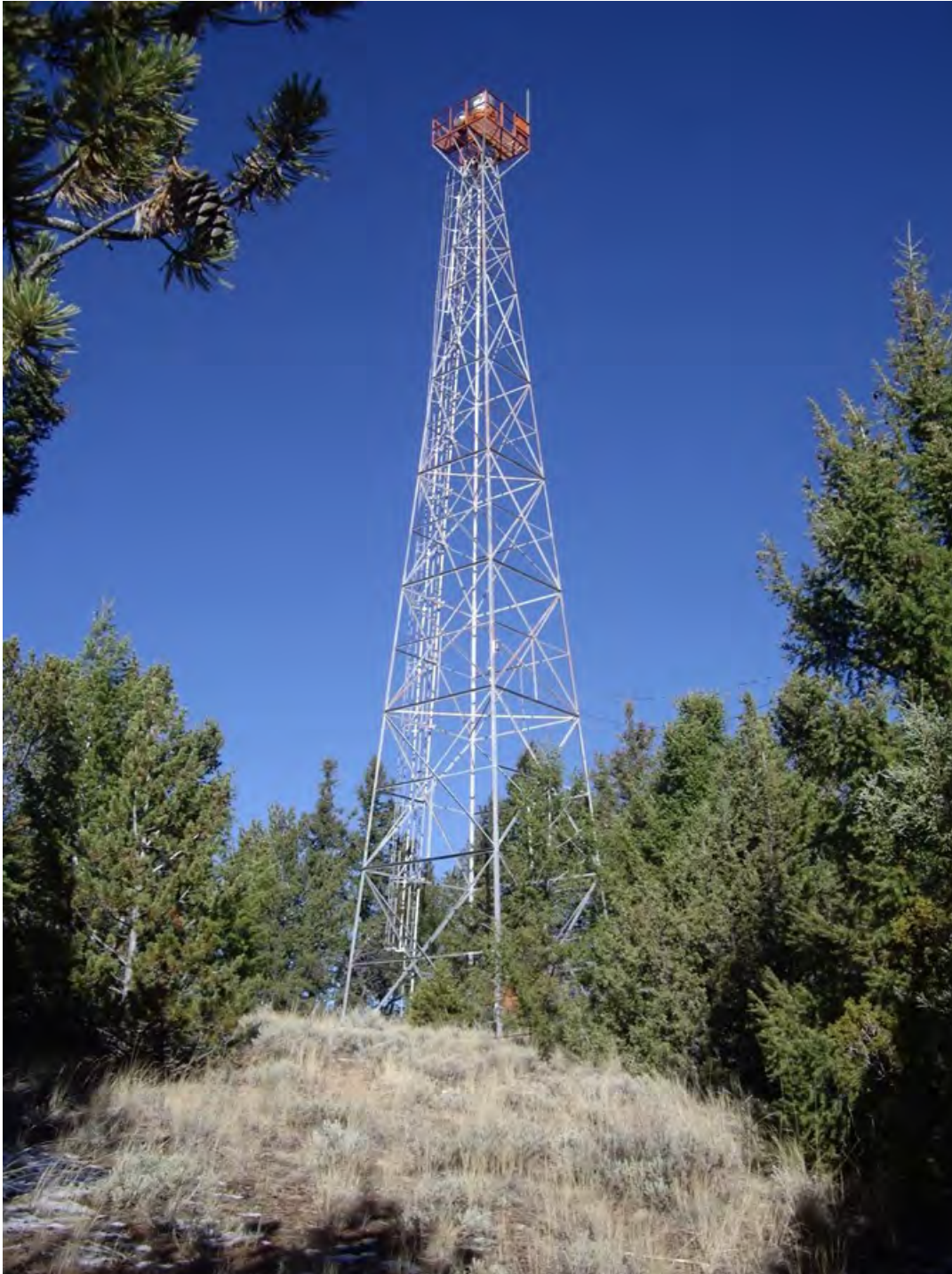
MT_BeaverheadCounty_CanyonResortAirwayBeacon_0005: View to North-northwest.
