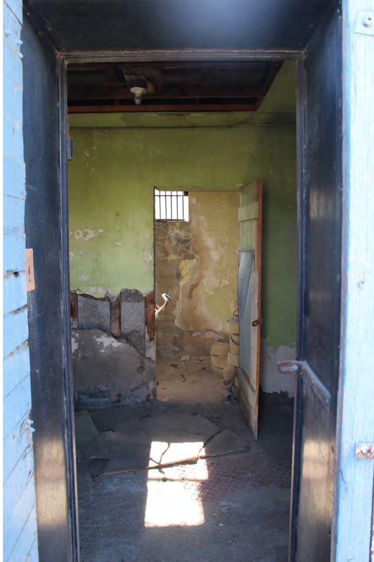
Cimarron City Jail view from the entrance into the rooms taken 2018
