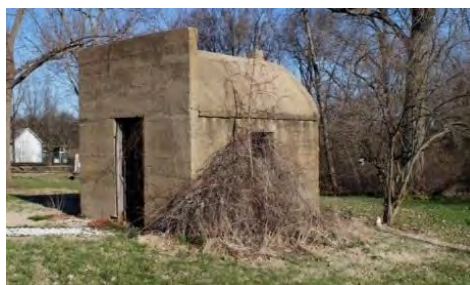
Figure 4: Hoyt City Jail. 31 March 2019
