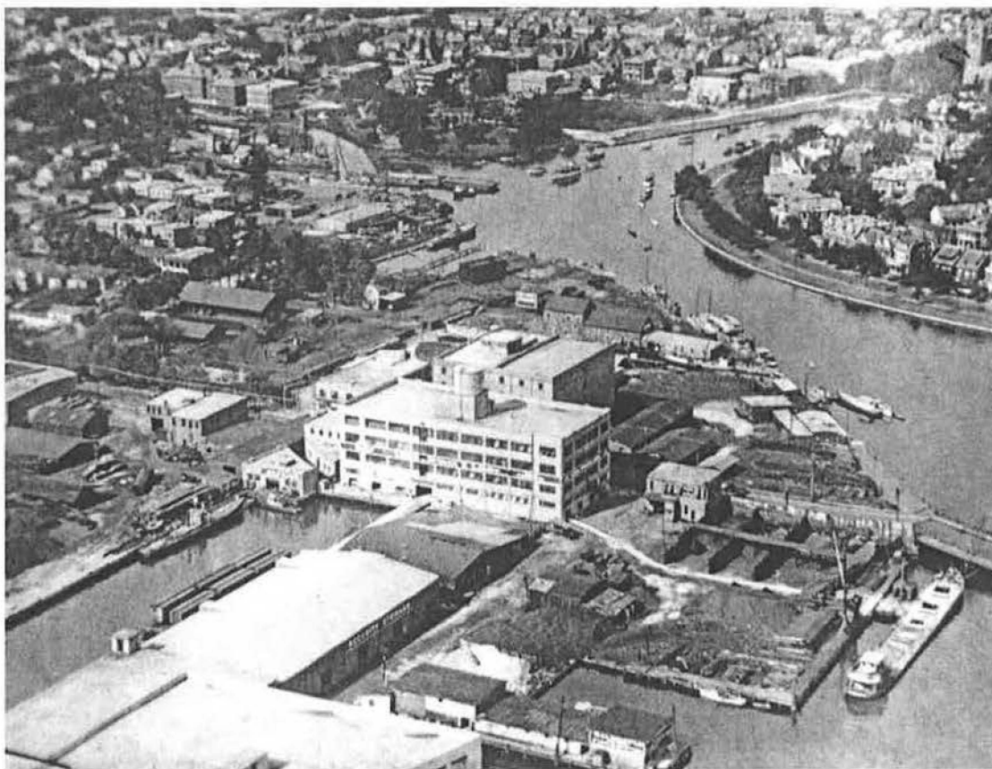
Figure 1. Security Storage & Safe Deposit Company Warehouse (center of picture), ca. 1923.
