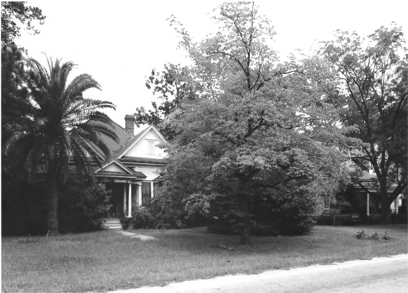
Brookwood North Historic District Valdosta, Lowndes Co., GA 16 of 47
