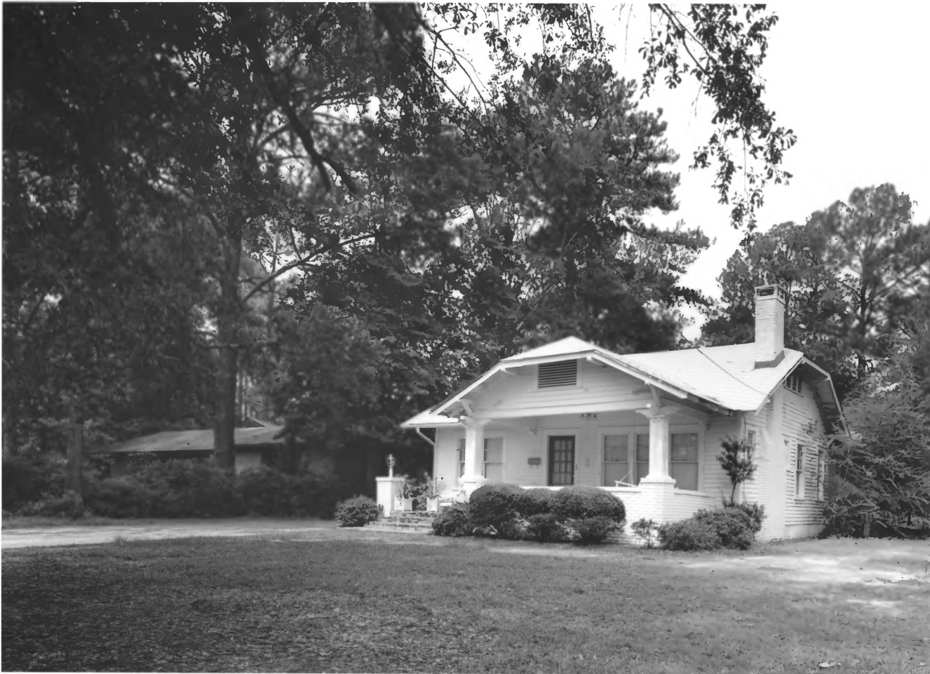
Brookwood North Historic District Valdosta, LOWNDES CO., GA 20 of 47
