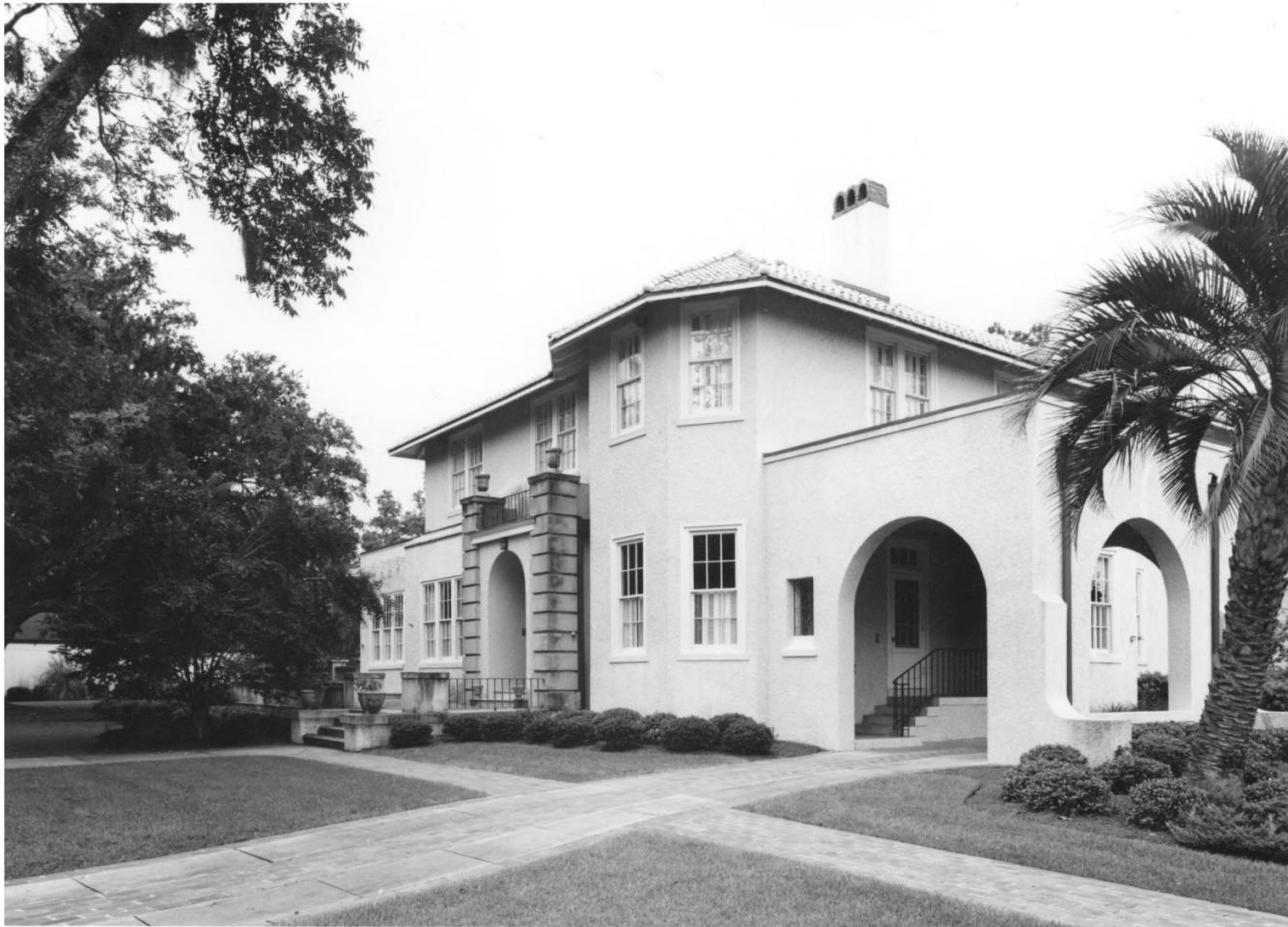
BROOKWOOD NORTH HISTORIC DISTRICT VALDOSTA, LOWNDES CO., GA 35 of 47
