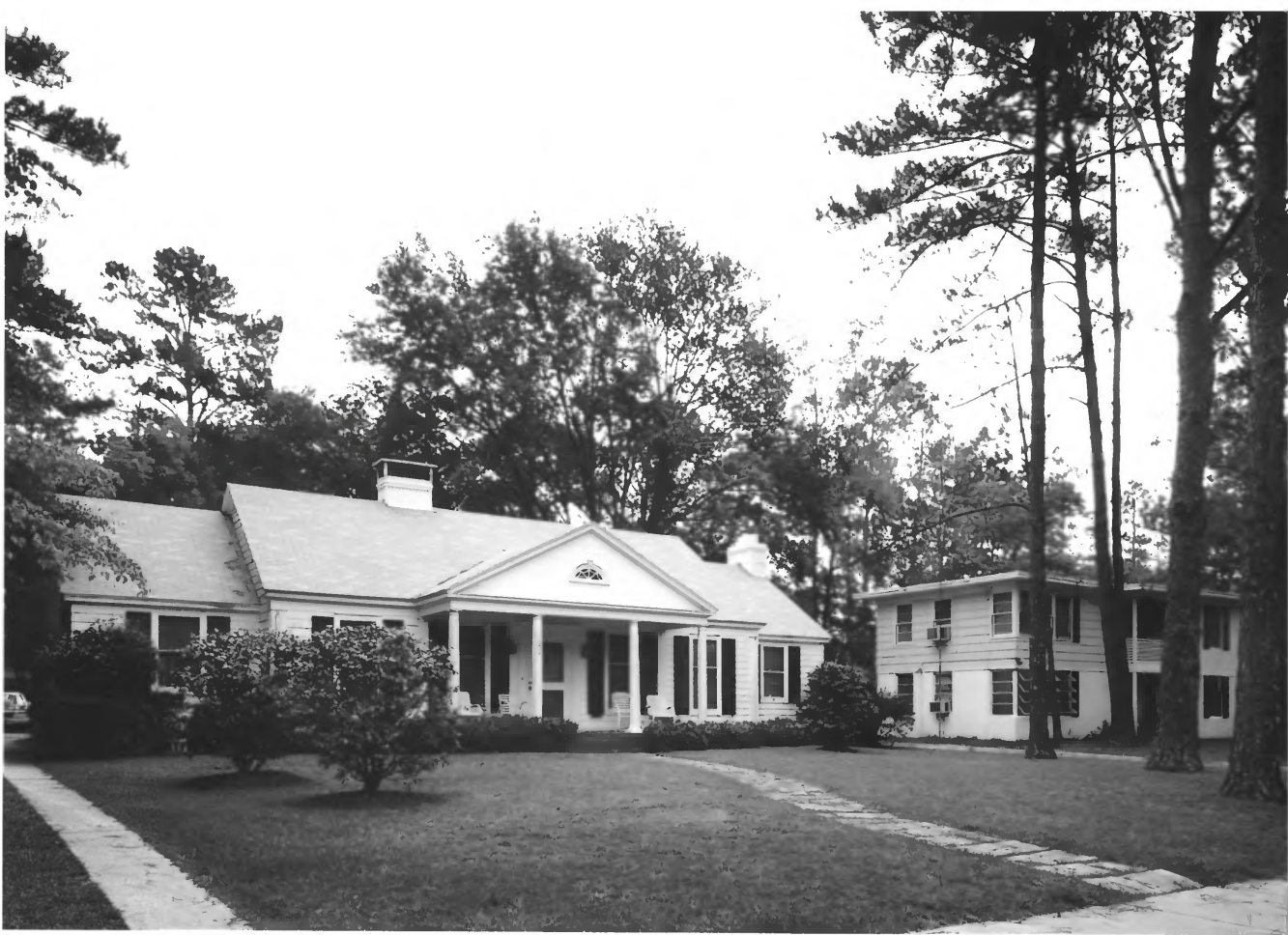
BROOKWOOD NORTH HISTORIC DISTRICT VALDOSTA, LOWNDES CO., GA 31 of 47
