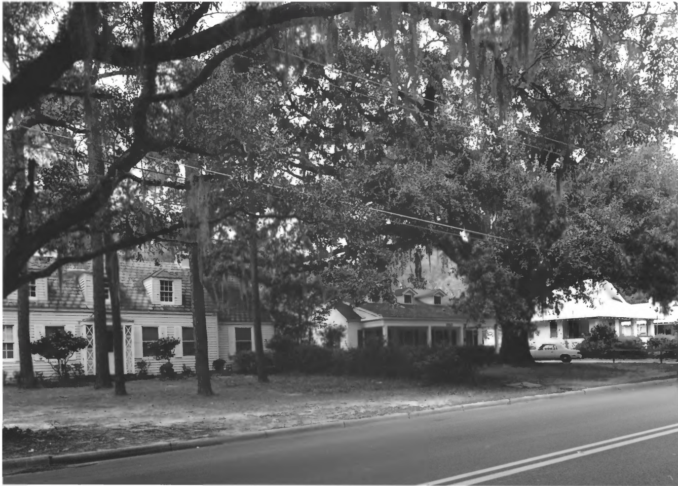
Brookwood North Historic District Valdosta, Lowndes Co., GA 9 of 47
