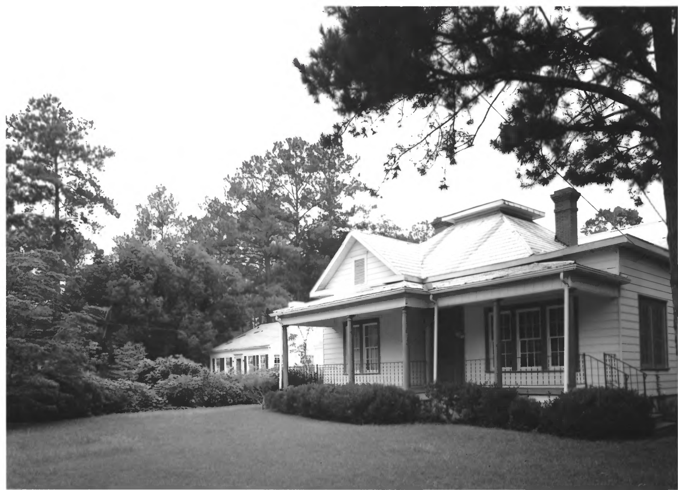
Brookwood North Historic District Valdosta, LOWNDES CO., GA 25 of 47
