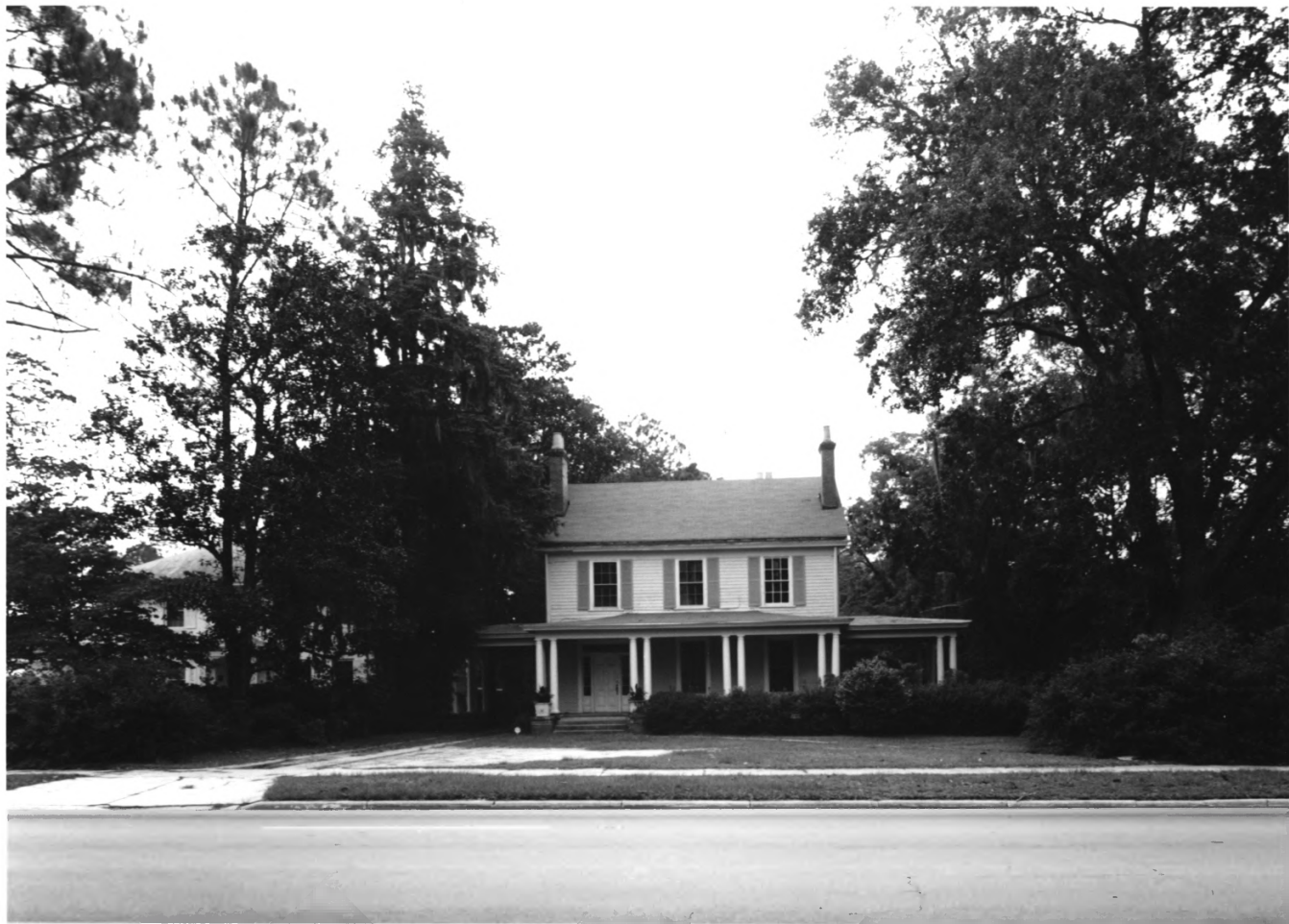
BROOKWOOD NORTH HISTORIC DISTRICT VALDOSTA, LOWNDES CO., GA 40 of 47
