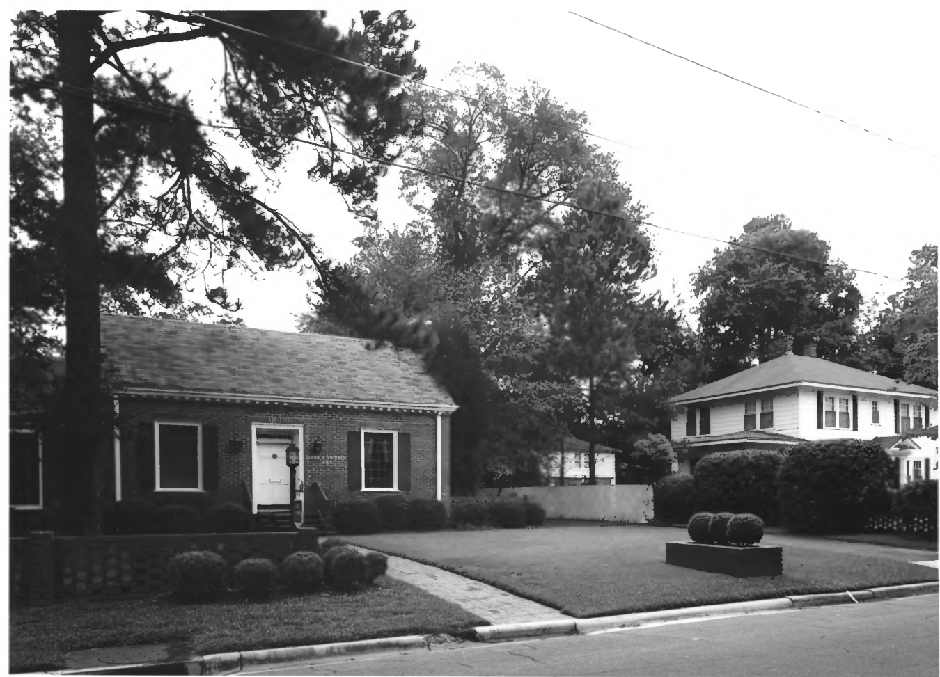
Brookwood North Historic District Valdosta, Lowndes Co., GA 22 of 47
