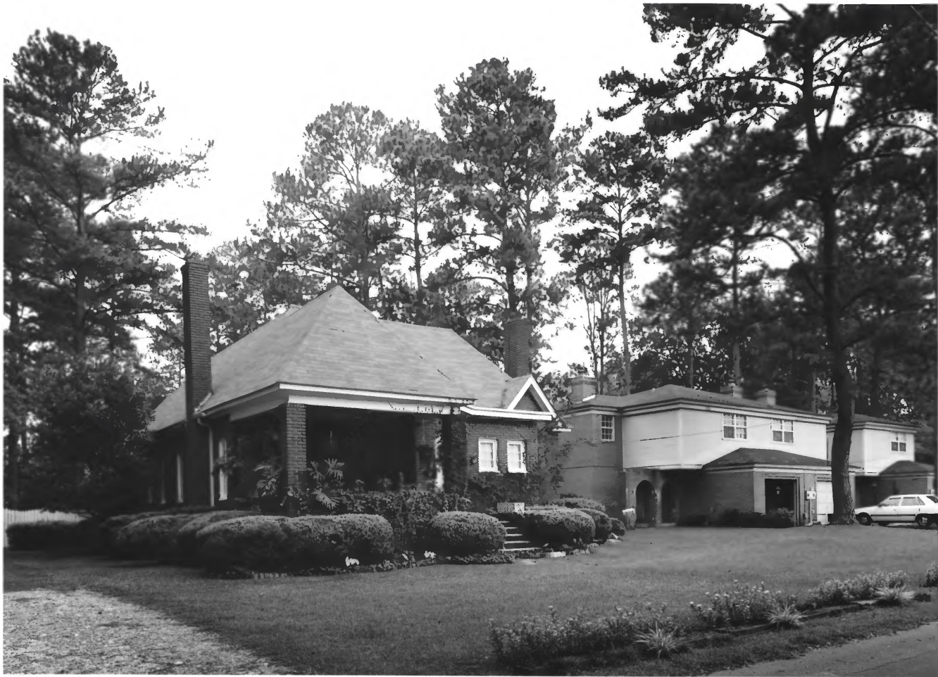
Brookwood North Historic District Valdosta, LOWNDES Co., GA 30 of 47
