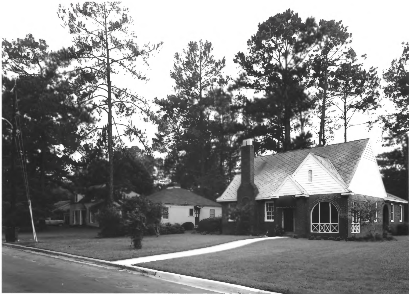
BROOKWOOD NORTH HISTORIC DISTRICT VALDOSTA, LOWNDES CO., GA 38 of 47
