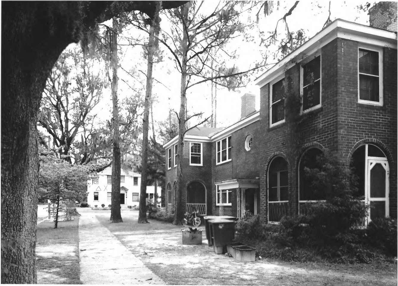
BROOKWOOD NORTH HISTORIC DISTRICT VALDOSTA, LOWNDES CO., GA 33 of 47
