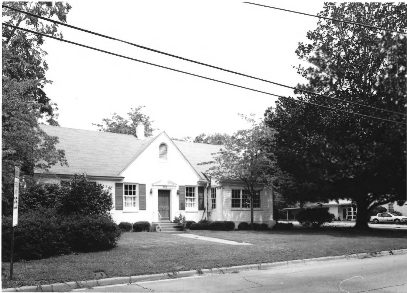
Brookwood North Historic District Valdosta, Lowndes Co., GA 4 of 47
