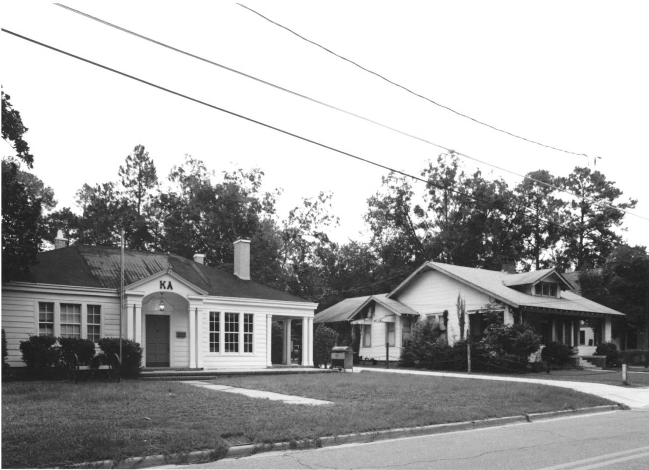
BROOKWOOD NORTH HISTORIC DISTRICT VALDOSTA, LOWNDES CO., GA 43 of 47
