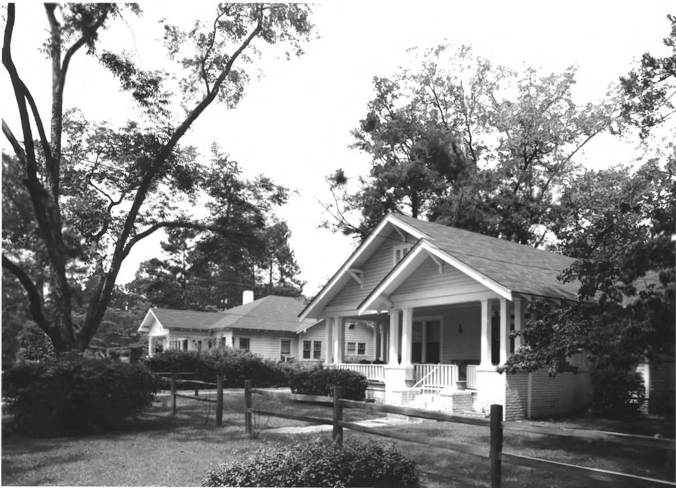
Brookwood North Historic District Valdosta, Lowndes Co., GA 15 of 47
