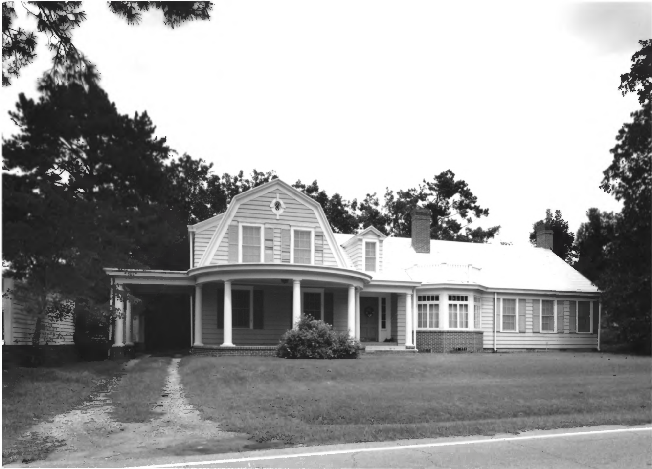
Brookwood North Historic District Valdosta, LOWNDES CO, GA 18 of 47
