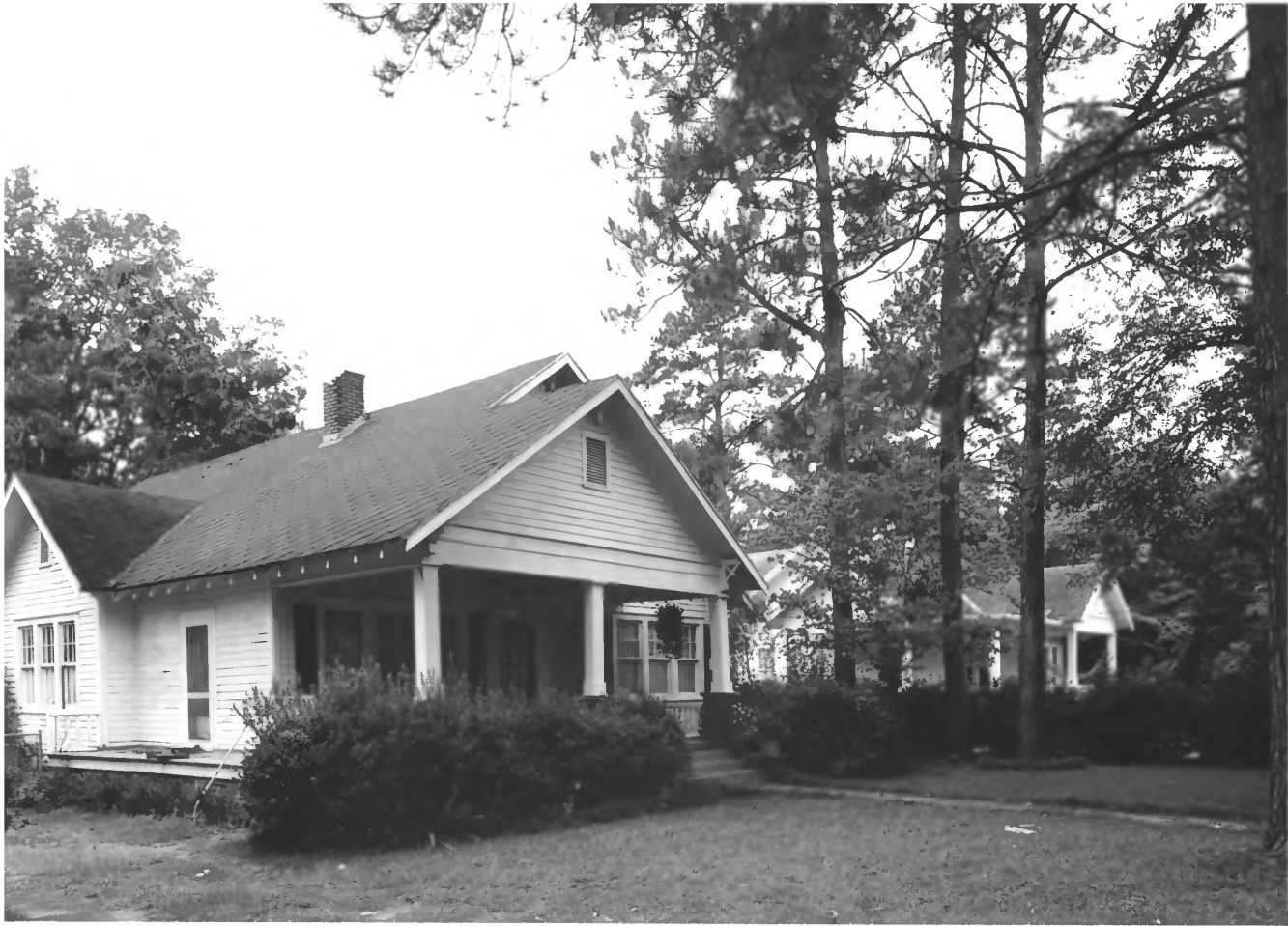
Brookwood North Historic District Valdosta, LOWNDES CO., GA 23 of 47
