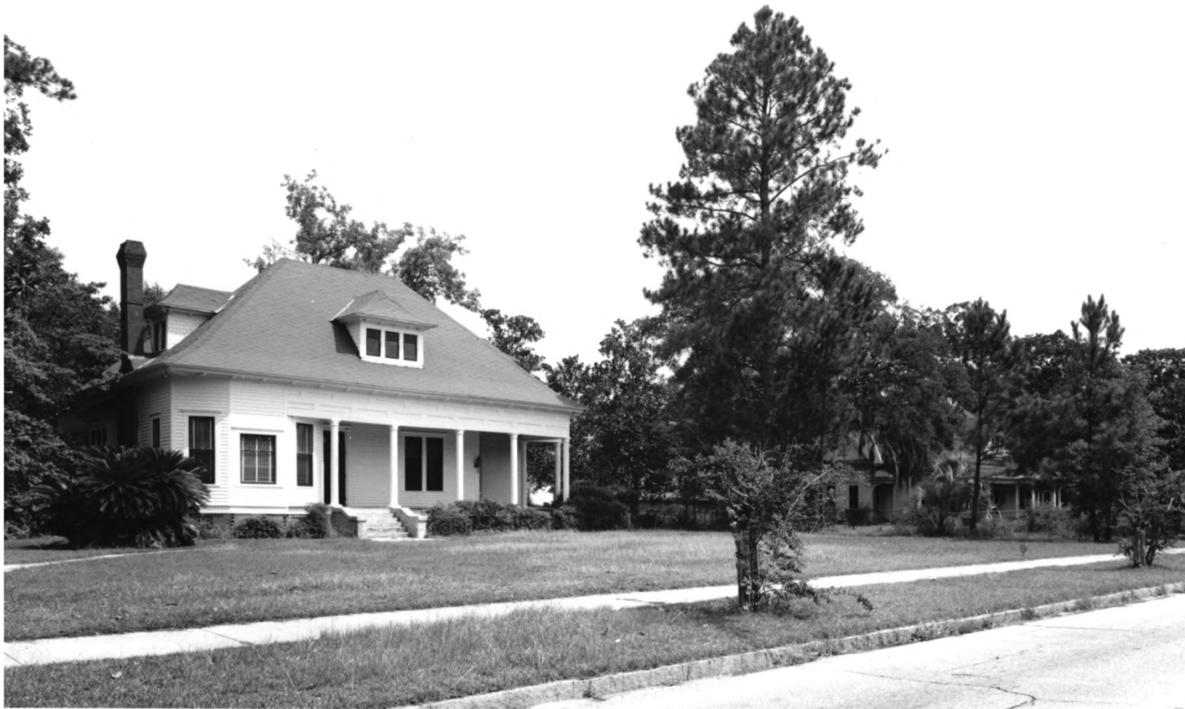
Brookwood North Historic District Valdosta, Lowndes Co., GA 2 of 47
