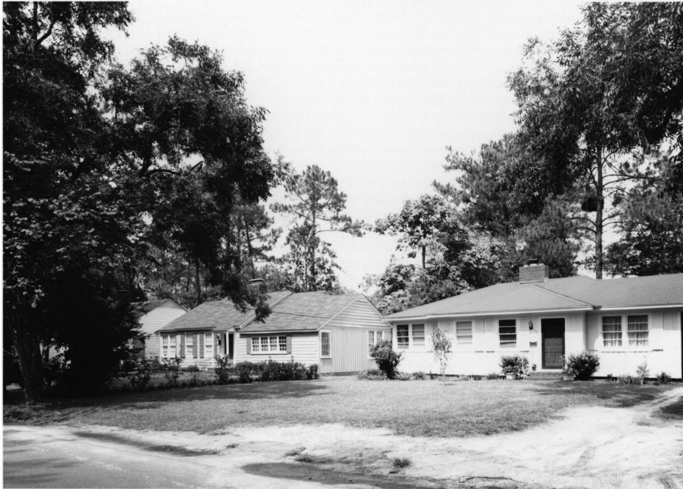
Brookwood North Historic District Valdosta, Lowndes Co., GA 14 of 47
