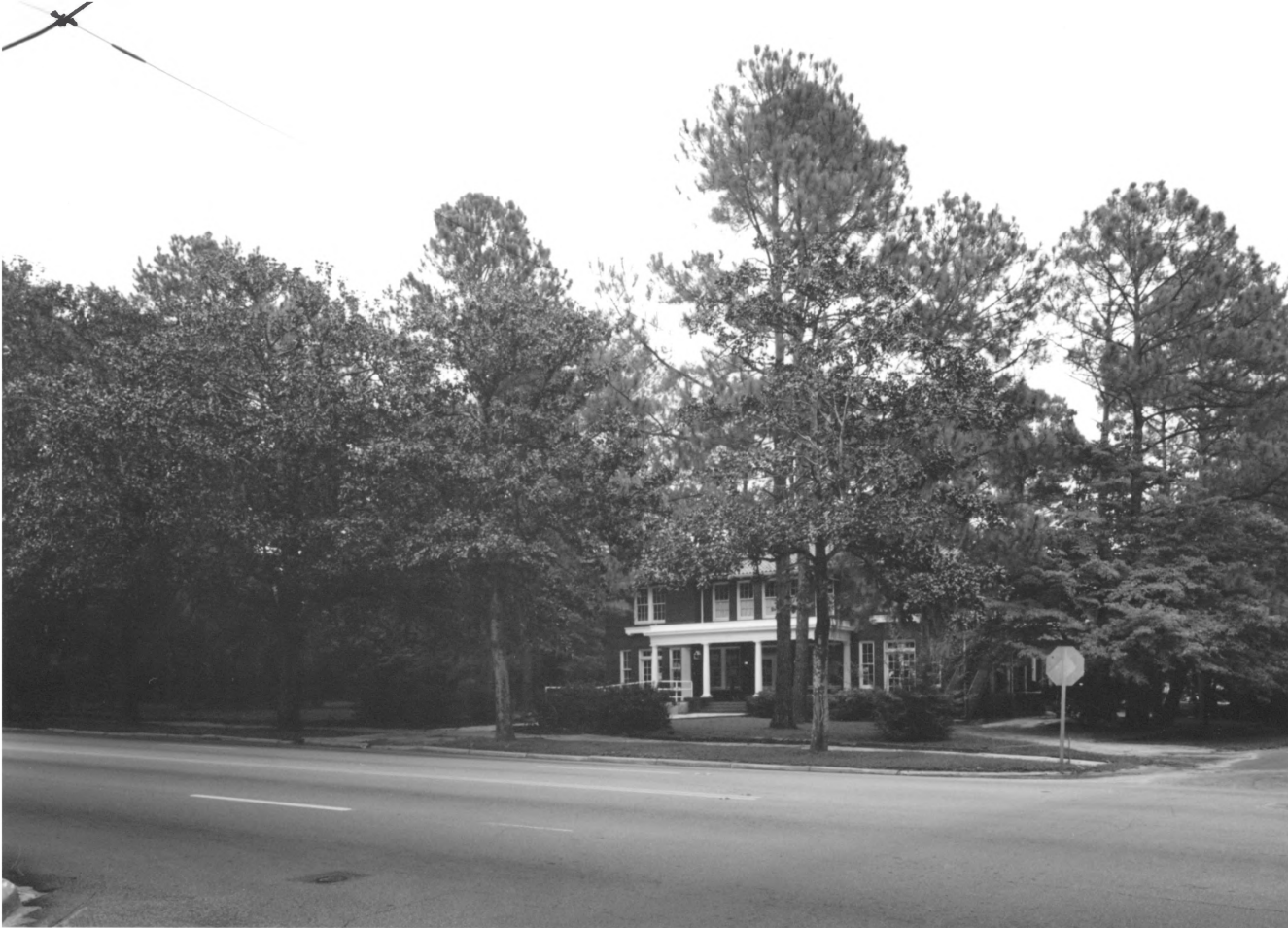
Brookwood North Historic District Valdosta, LOWNDES CO., GA 24 of 47
