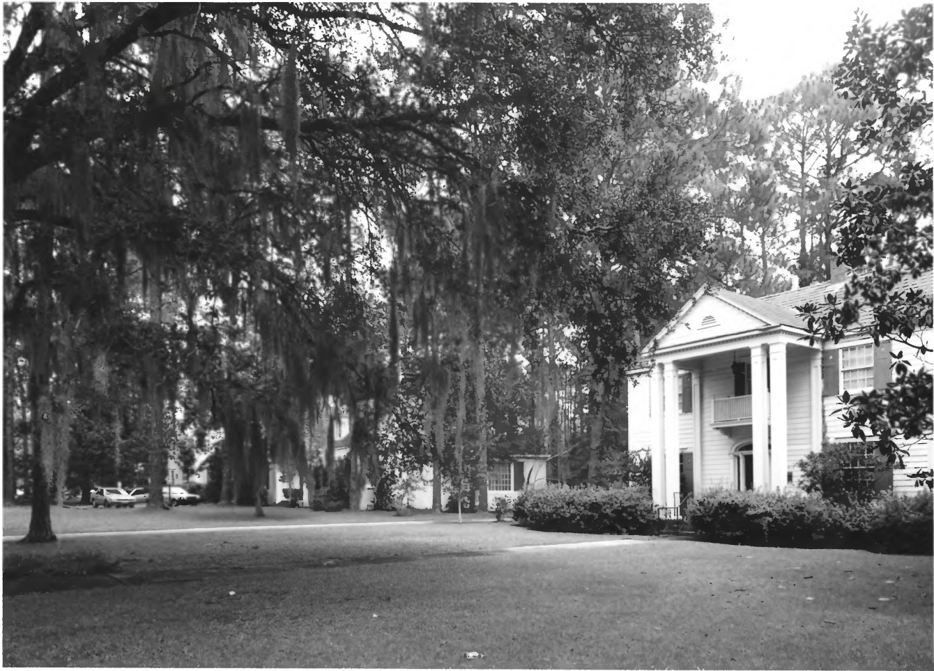
Brookwood North Historic District Valdosta, Lowndes Co., GA 8 of 47
