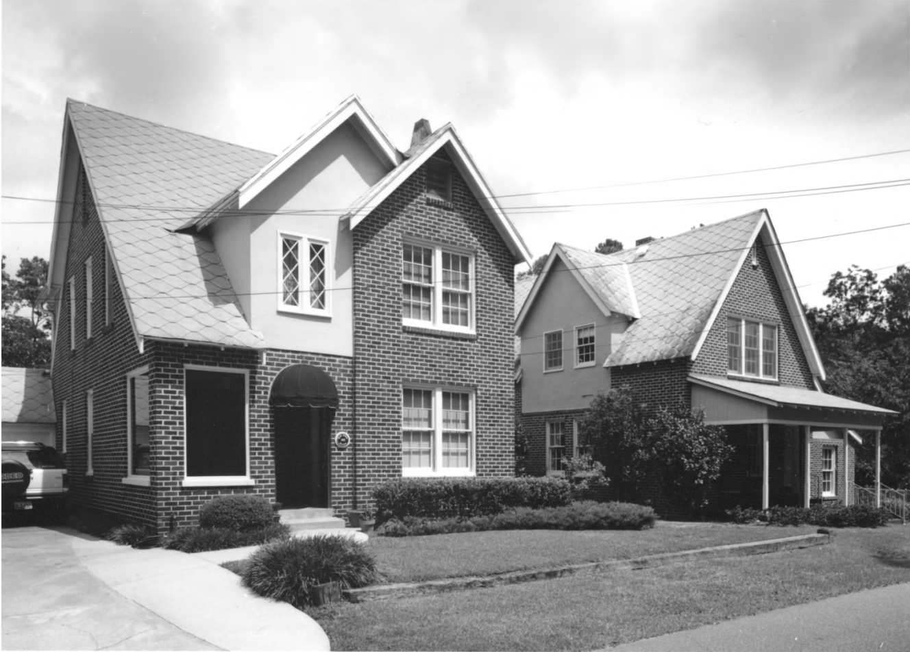
Brookwood North Historic District Valdosta, Lowndes Co., GA 12 of 47
