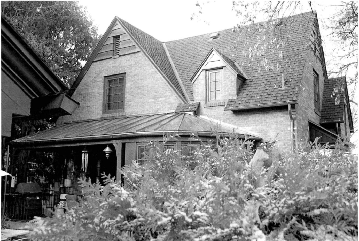
South elevation, photo by Barbara Behan, October 2005
