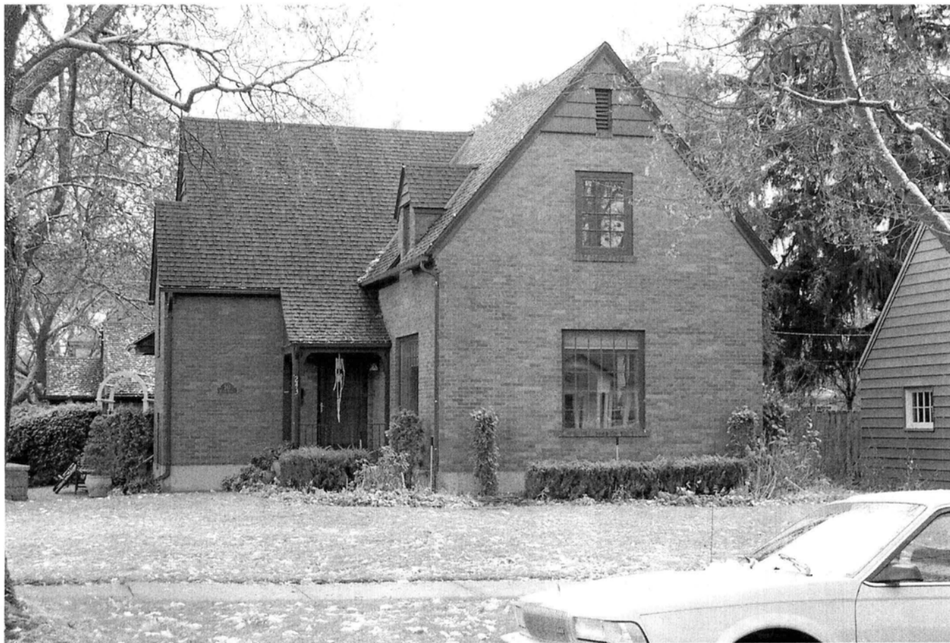
North elevation, photo by Barbara Behan, October 2005
