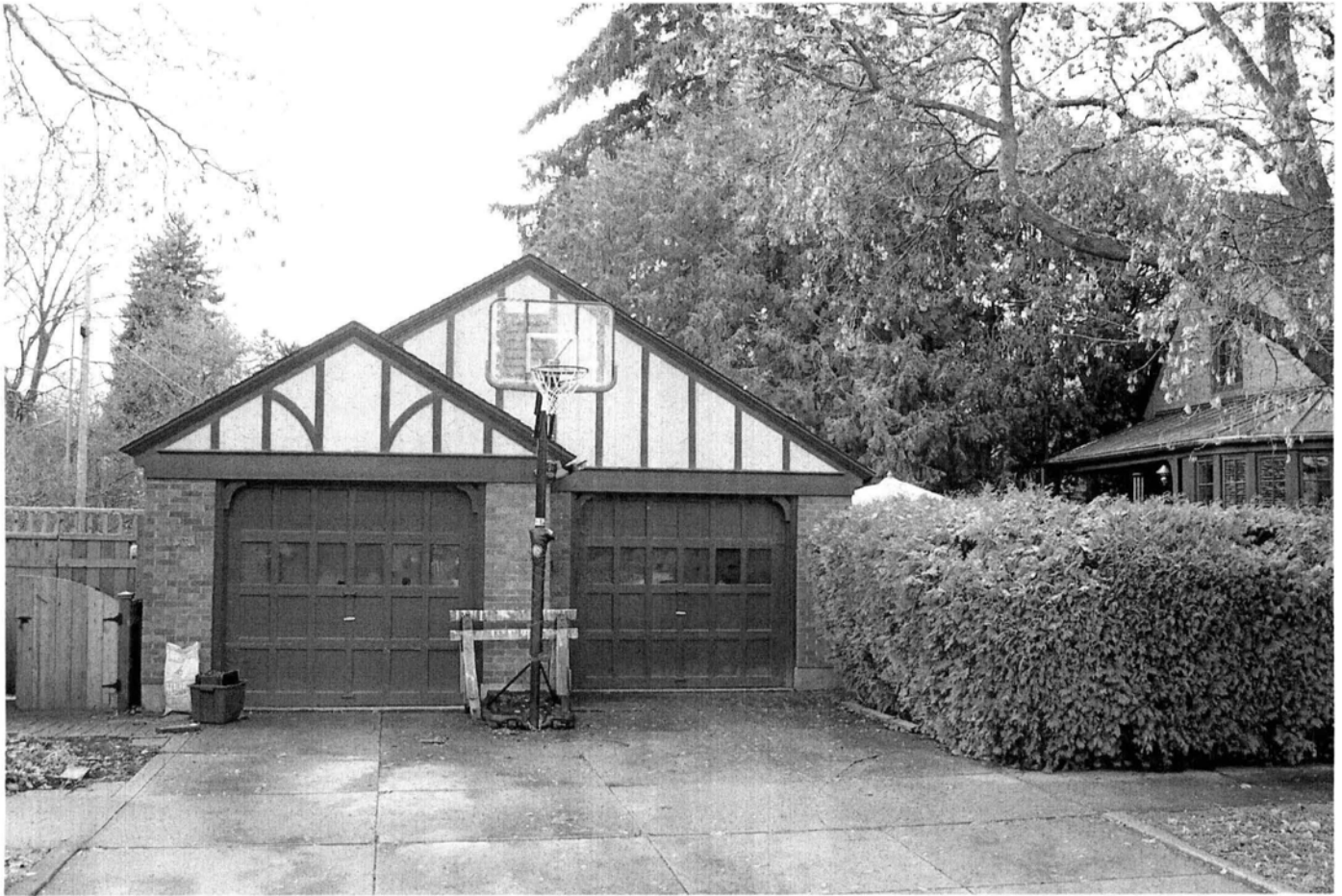
Garage – east elevation, photo by Barbara Behan, October 2005
