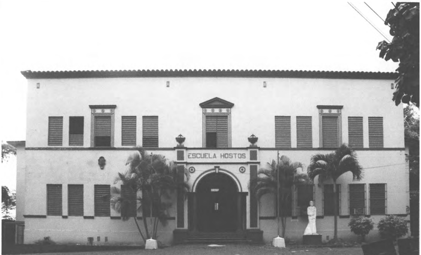
FIG. 2: Eugenio María de Hostos School northeast elevation, looking southwest. Main facade existing conditions in the town of Las Marías, Puerto Rico. Original reversed hipped roof and wood louvers windows has been substituted but the fenestrations retain their original proportions. The frontispiece on center is a predominant feature in otherwise bare façade. Windows in group of five, featuring interrupted cornice on ground floor, highlighted center window on second floor level and cartouche underneath central window. A cornice on ground floor level breaks with each window's opening at window sill height. Portions of the openings have been filled adroitly in cement, corresponding with the top of the cornice, to accommodate smaller window units. At roof level height one of four lantern shape, low-relief, coarse finish inlay, concrete motif are distributed along the front façade below a cornice. Photo: Mariana Morales, May 28, 2012.
