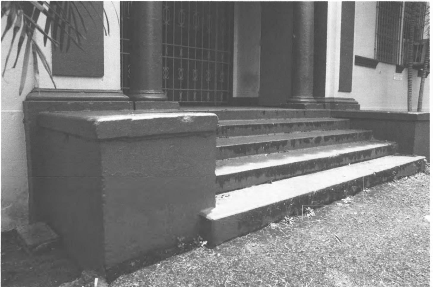
FIG. 3: Eugenio María de Hostos School northeast elevation, looking southwest. A five stepped stoop with no handrails flanked by a low pier at each side; acts like a pedestal for the pilasters. Photo: Mariana Morales, May 28, 2012.
