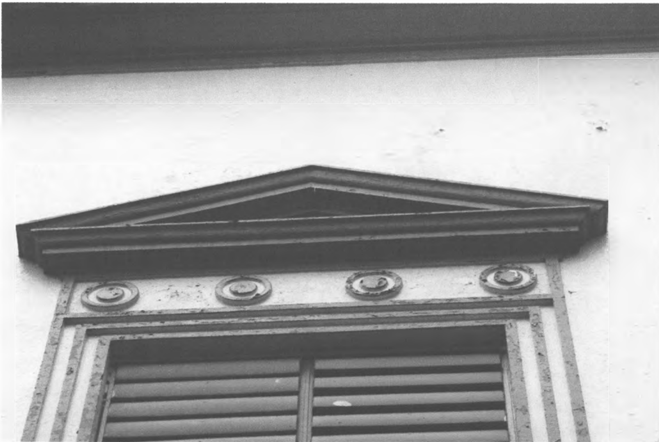
FIG.5: Eugenio María de Hostos School exterior detail, looking southwest. Highlighting the window at center, where the principal's office used to be located. Three flat (fillet) moldings surrounds the 4'-3" wide opening. Above, a small entablature framed by a single fillet molding encases four "bull's-eye" round medallions laid-out horizontally. On top a pediment crowns on axis the second floor window. Photo: Mariana Morales, May 28, 2012.
