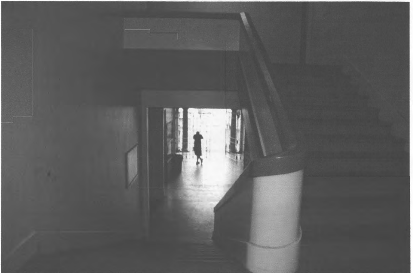
FIG.7: Eugenio María de Hostos School interior view, looking northeast. The stairway is built in concrete and is located on axis with the main entrance prominently featured with a double height space. The dog-leg stair is plain and wide, they feature a round post where the center balustrade ends at the curtail step. Steps are finished in polished concrete and include stair nosings. Photo: Mariana Morales, May 28, 2012.
