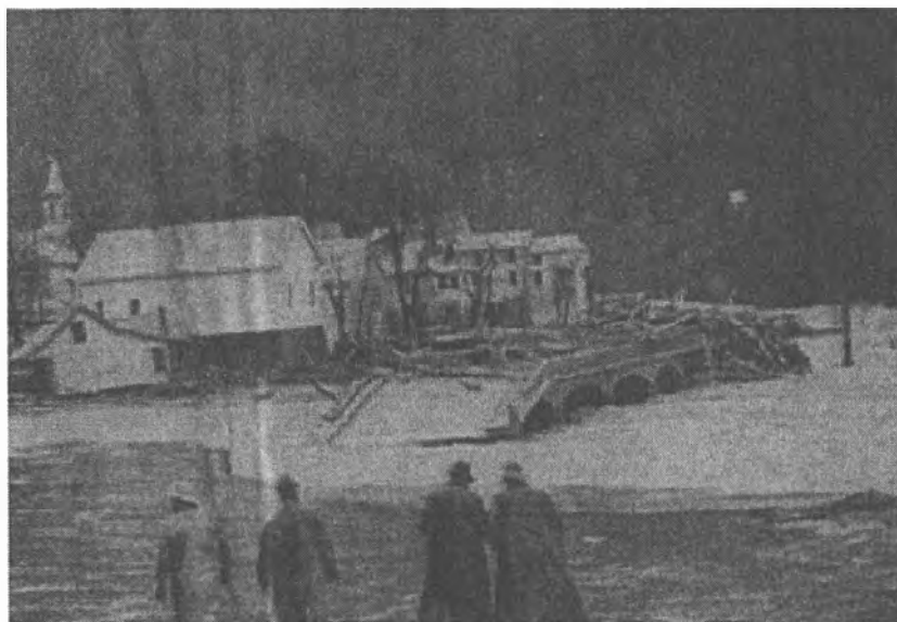
Figure 3. Historic photo of damaged highway bridge, 1937
