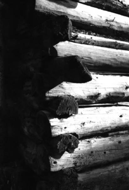
Orin Mallette Cabin, northeast (dogtrot) corner of west pen, with saddle-notching and half-notching
