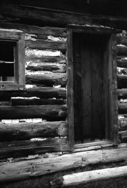
Orin Mallette Cabin, center of south facade of west pen, showing gun-notch in log to left of top of door
