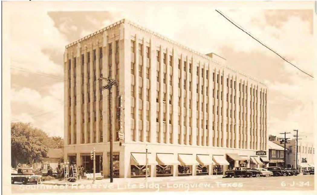
Figure 7. McWilliams (Southwest Reserve Life Insurance) Building c. 1940. Courtesy of the Texas Historical Commission.
