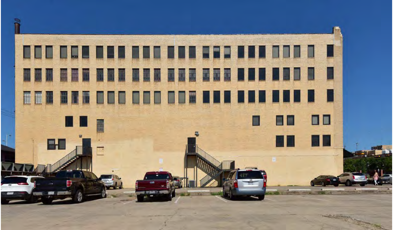
Photo 3. East Elevation, view W.
