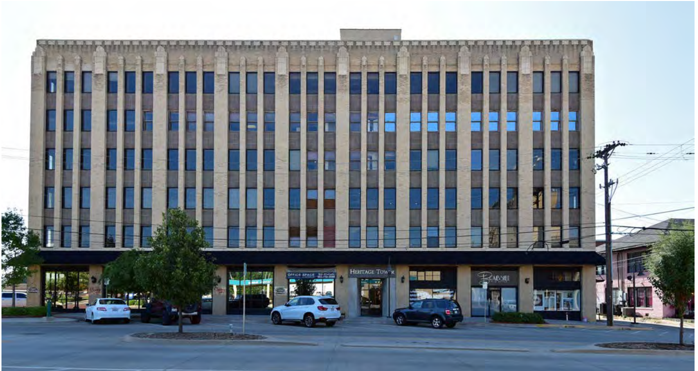
Photo 1. West elevation, view E.
