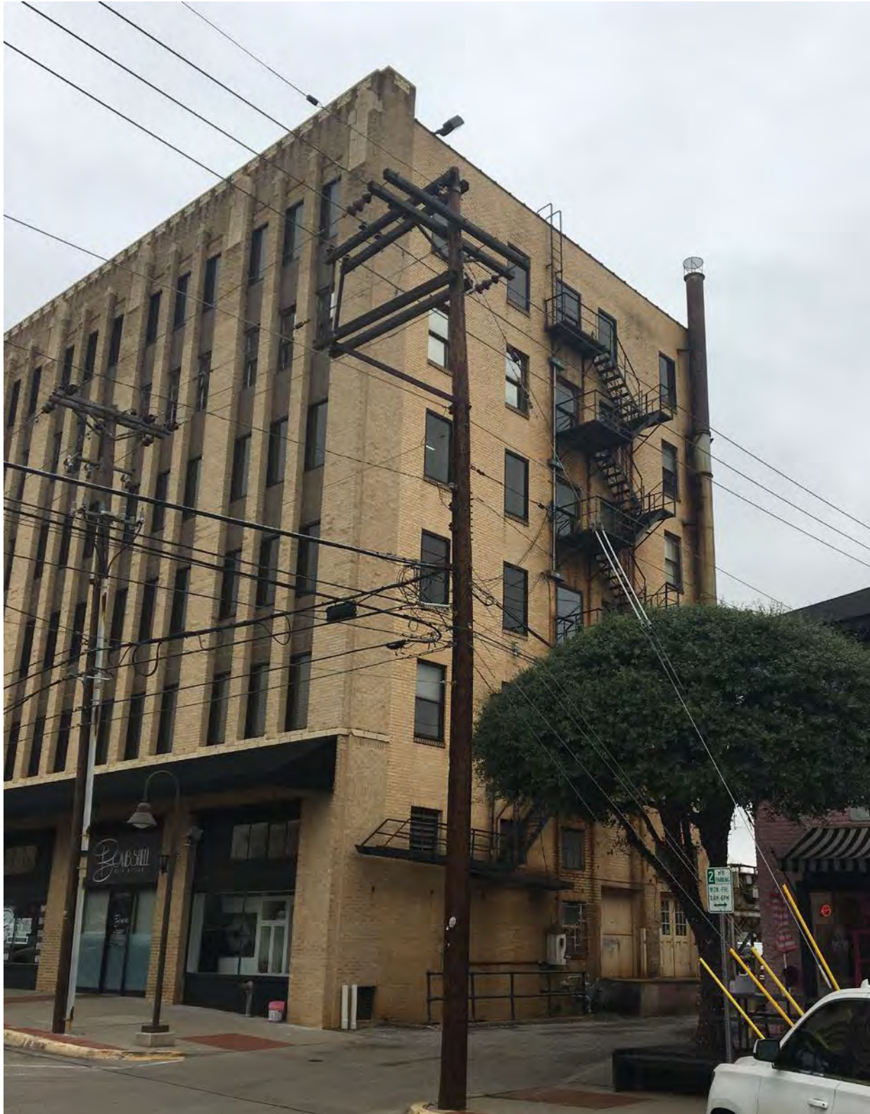
Photo 4. South elevation, view NE.
