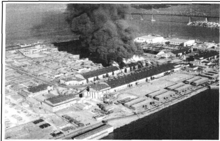
Figure 12. Former pavilions on fire at Treasure Island, April 10, 1947 with the Hall of Transportation and Palace of Fine and Decorative Arts shown in upper right. [Record Group 80-G, Negative 397192, NARA]
