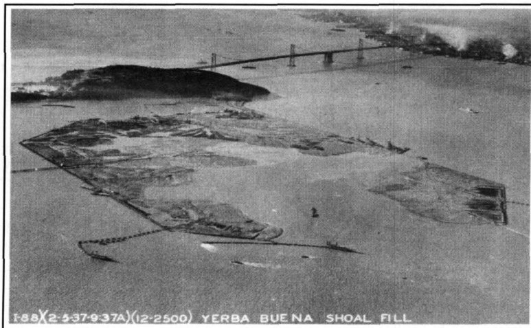
Figure 2. Filling of Yerba Buena Shoals, showing construction of the administration and hangar buildings, February 5, 1937. [Treasure Island Museum Collection]
