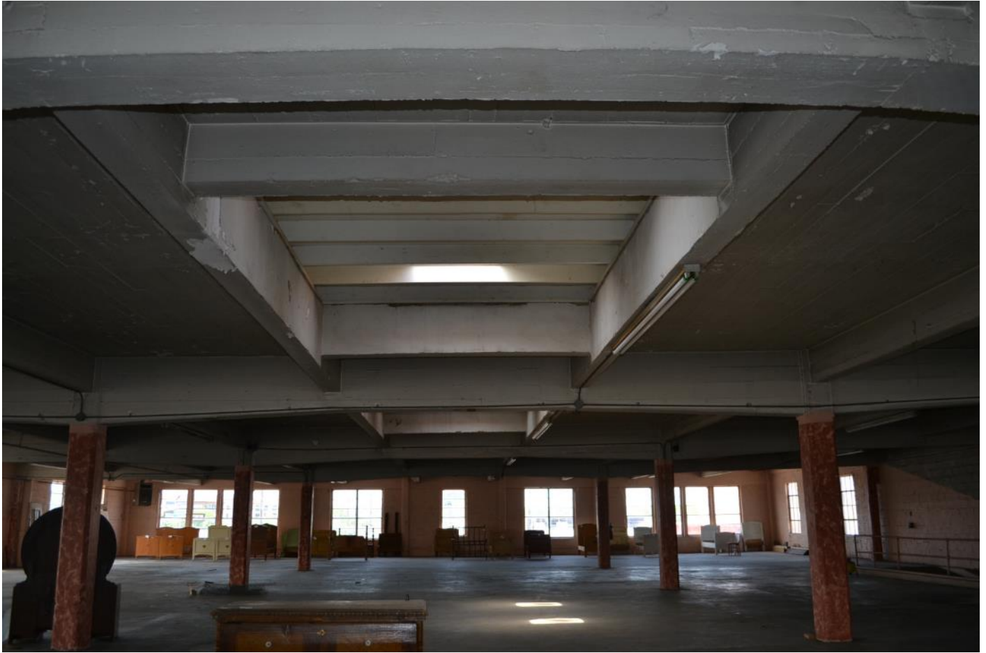
Photo 9: Poe Motor Company, interior, second floor, skylight detail
