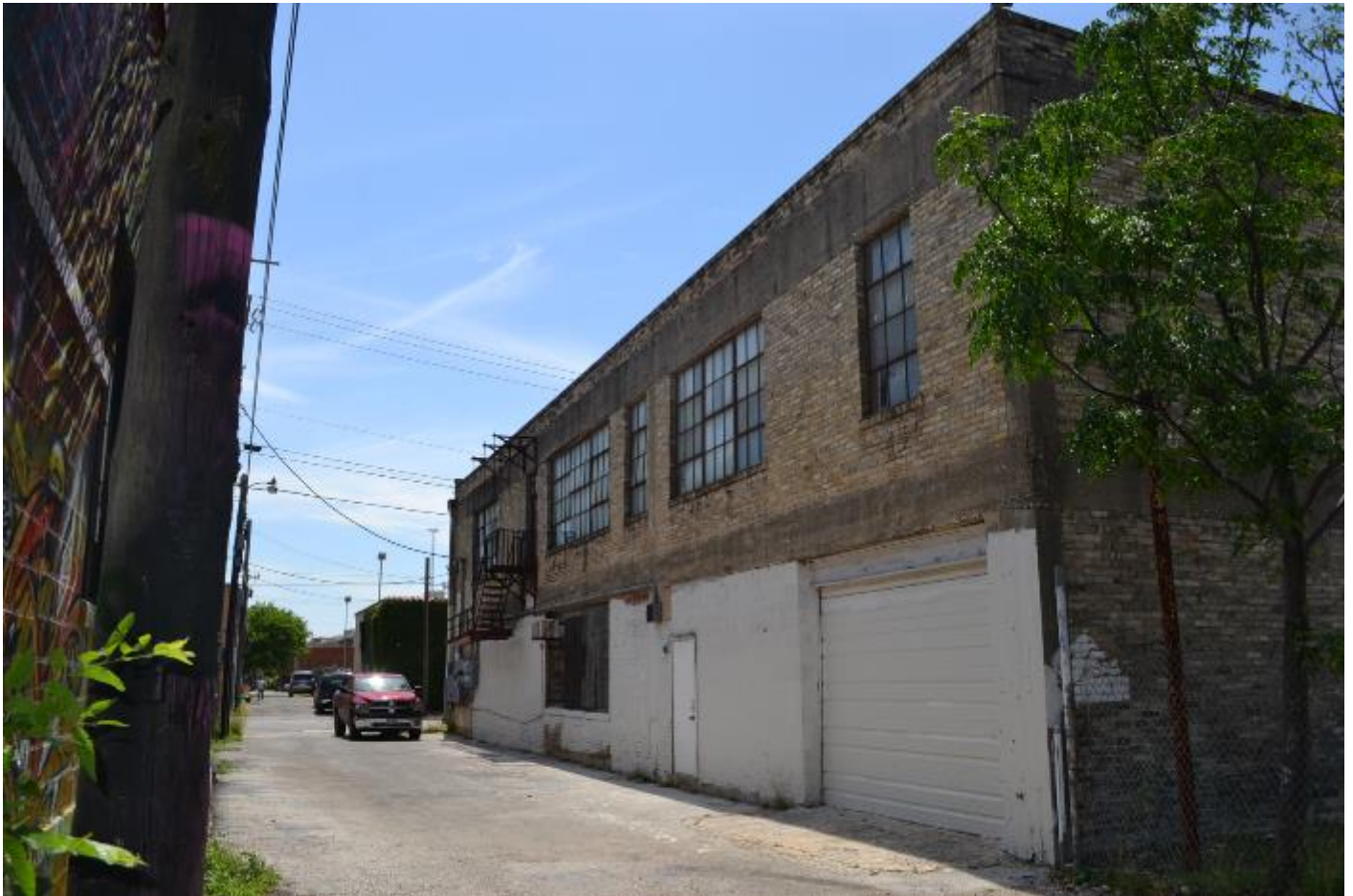
Photo 5: Poe Motor Company, southeast elevation, view west
