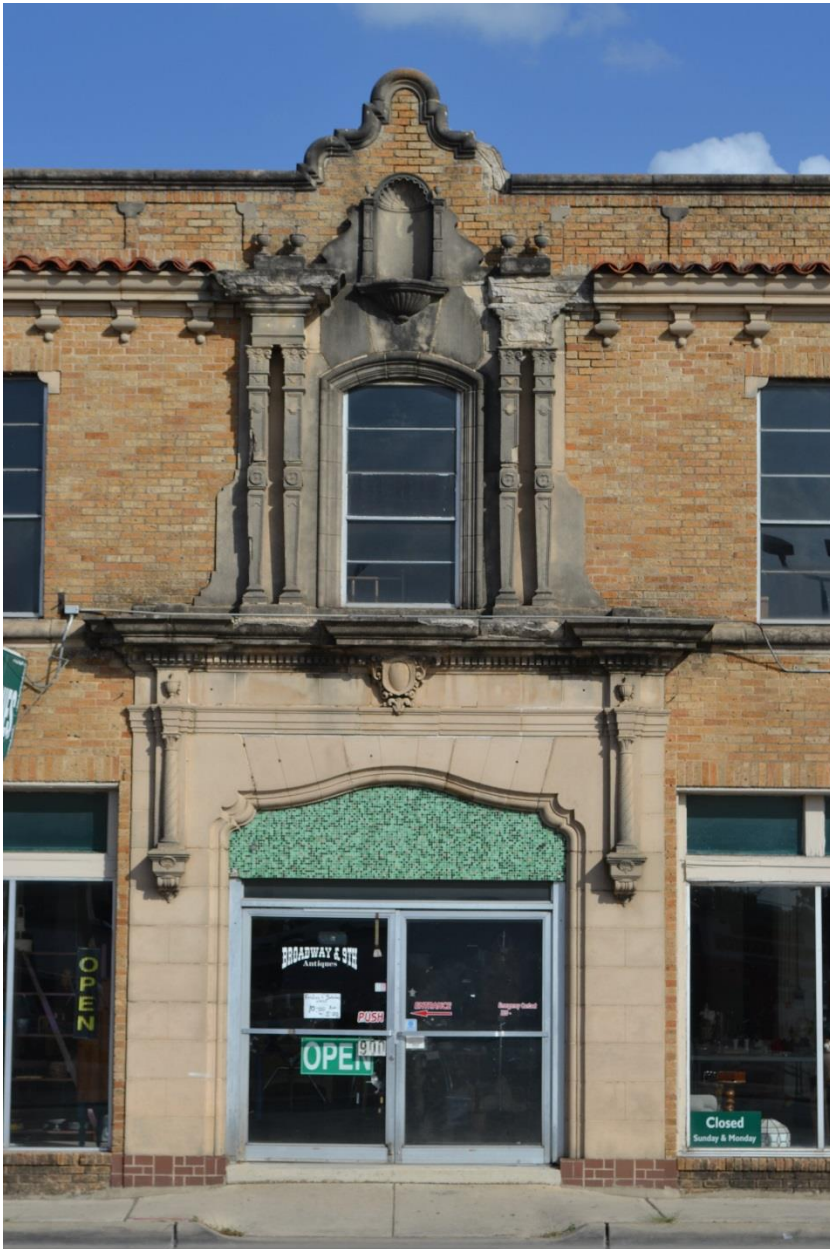
Photo 11: Poe Motor Company, northwest elevation entry detail, view southeast
