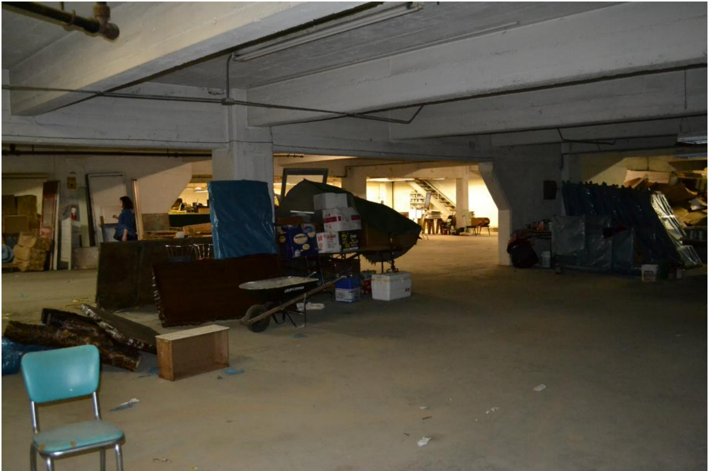
Photo 10: Poe Motor Company, interior, basement
