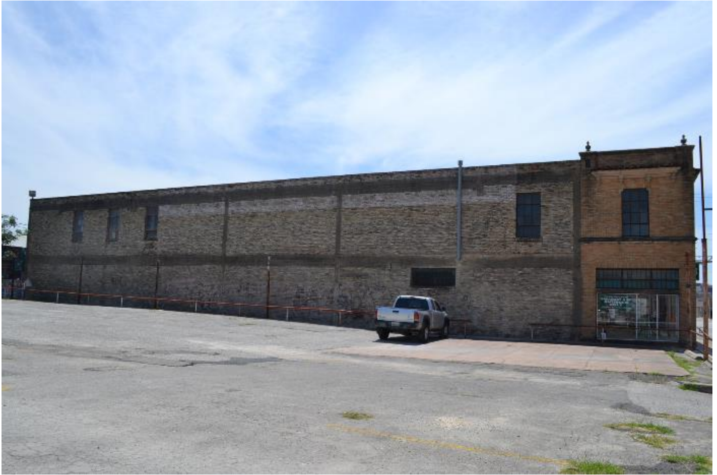
Photo 4: Poe Motor Company, northeast elevation, view southwest
