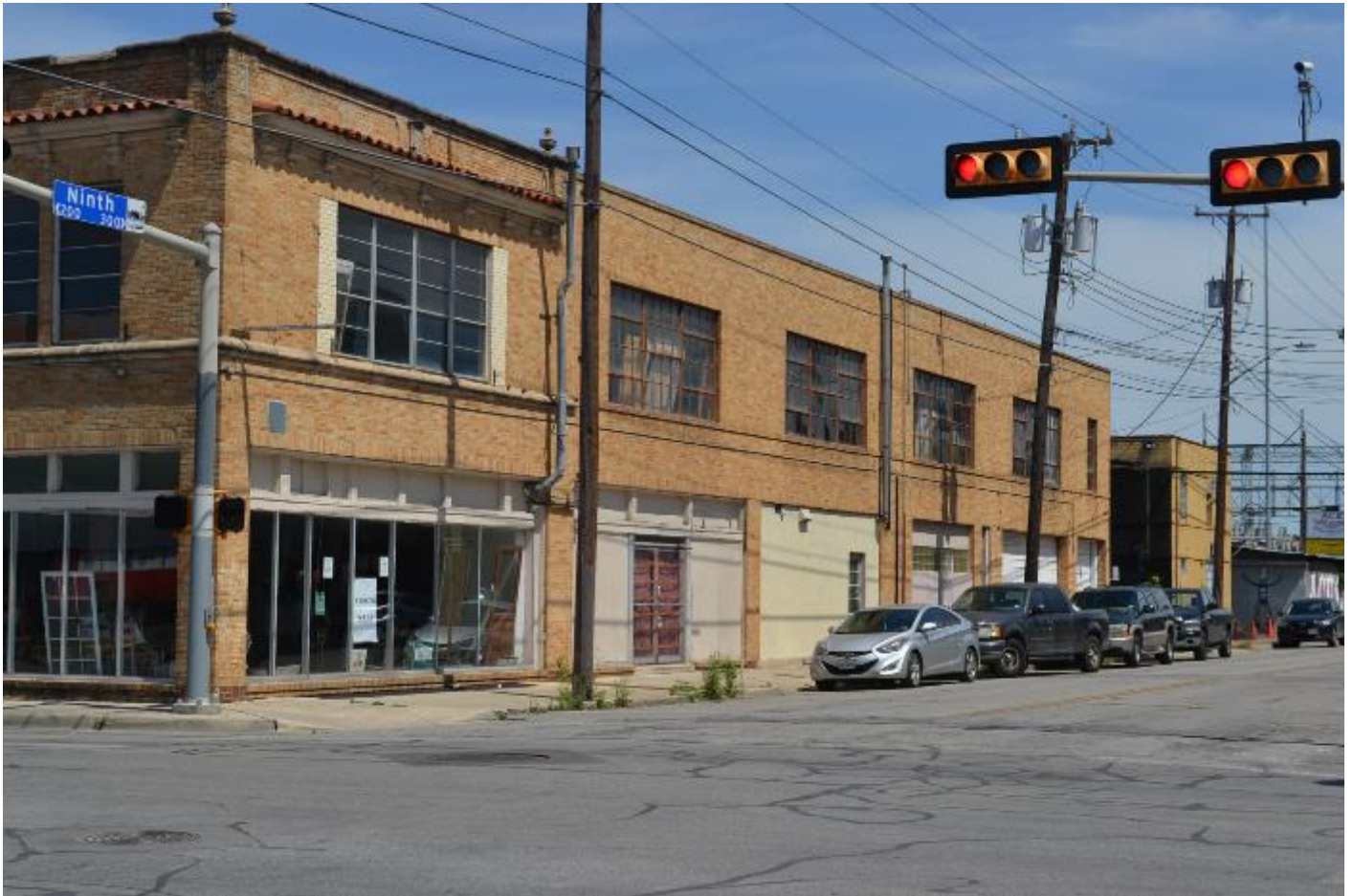
Photo 3: Poe Motor Company, southwest elevation, view east
