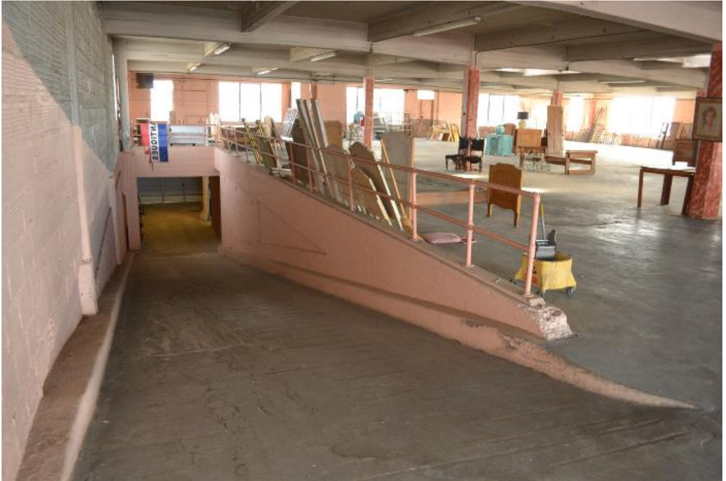
Photo 7: Poe Motor Company, interior, vehicular ramp, view from second floor
