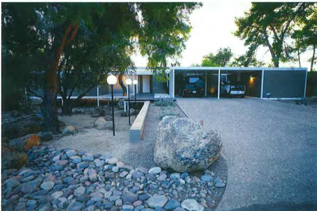
Photograph 2 of 19. Front façade, facing southwest.
