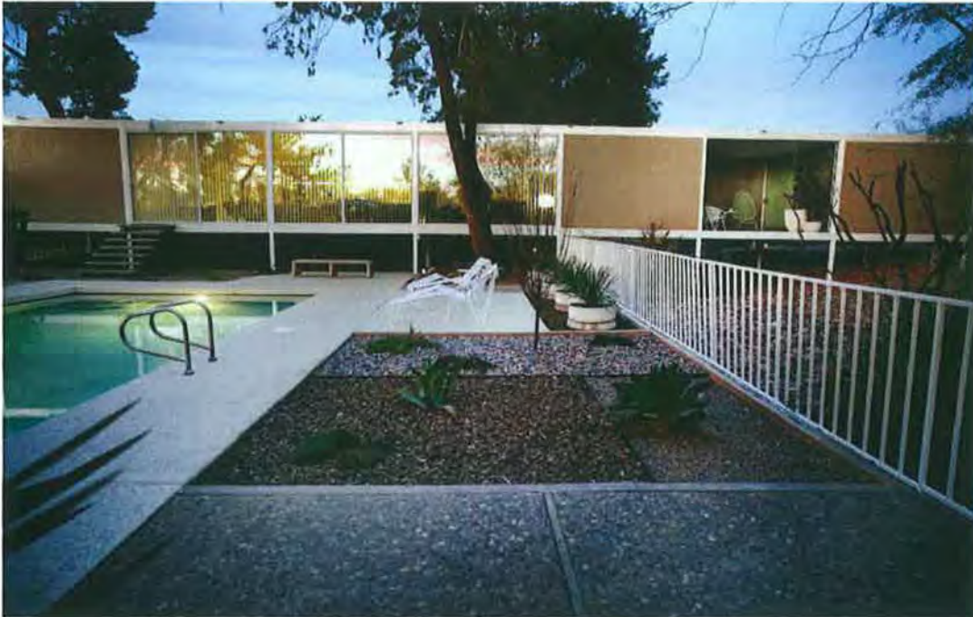
Photograph 10 of 19. Rear façade and planting areas, facing north.
