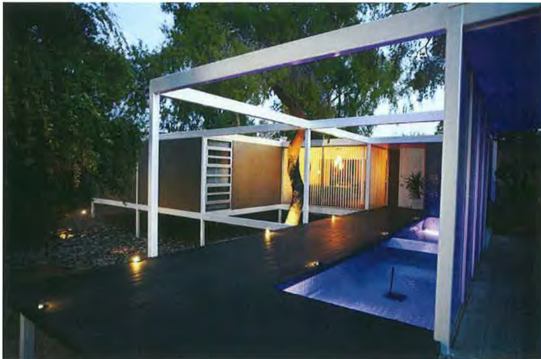
Photograph 5 of 19. Boardwalk, facing south.
