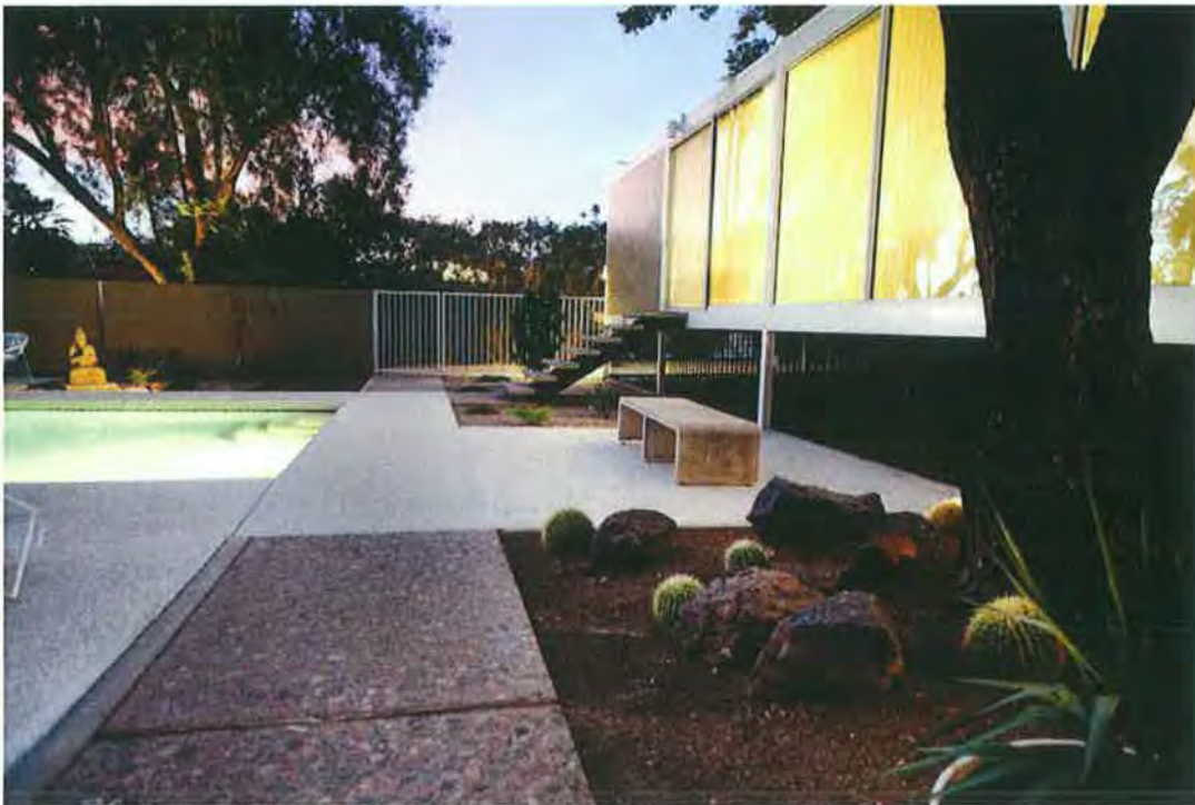
Photograph 9 of 19. Rear façade, facing west.
