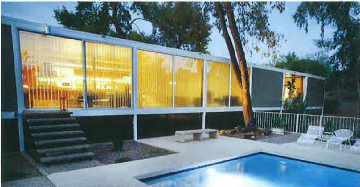
Figure 4. The rear of the house. Sara Abbott, 2016.
