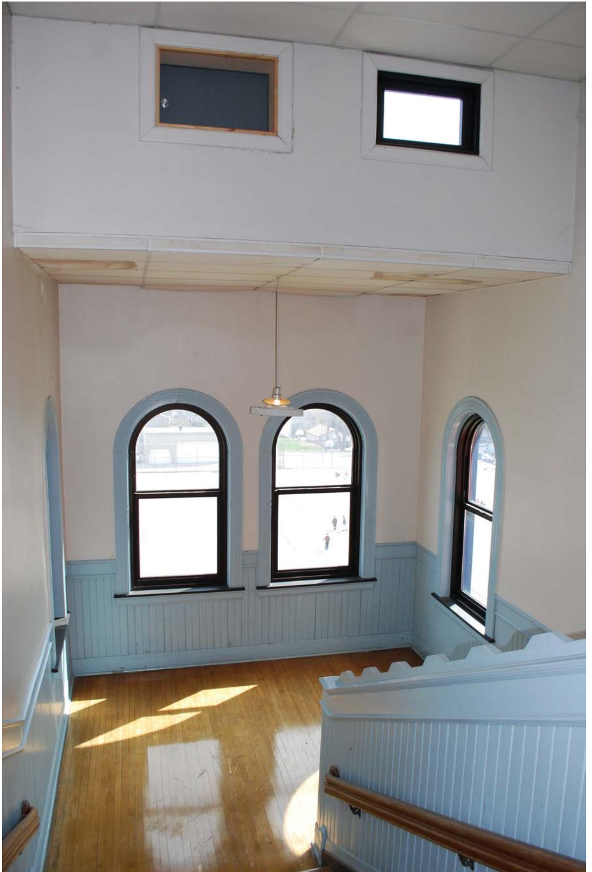
Dover Street School and Social Center, City of Milwaukee, Milwaukee County, 12 of 14
