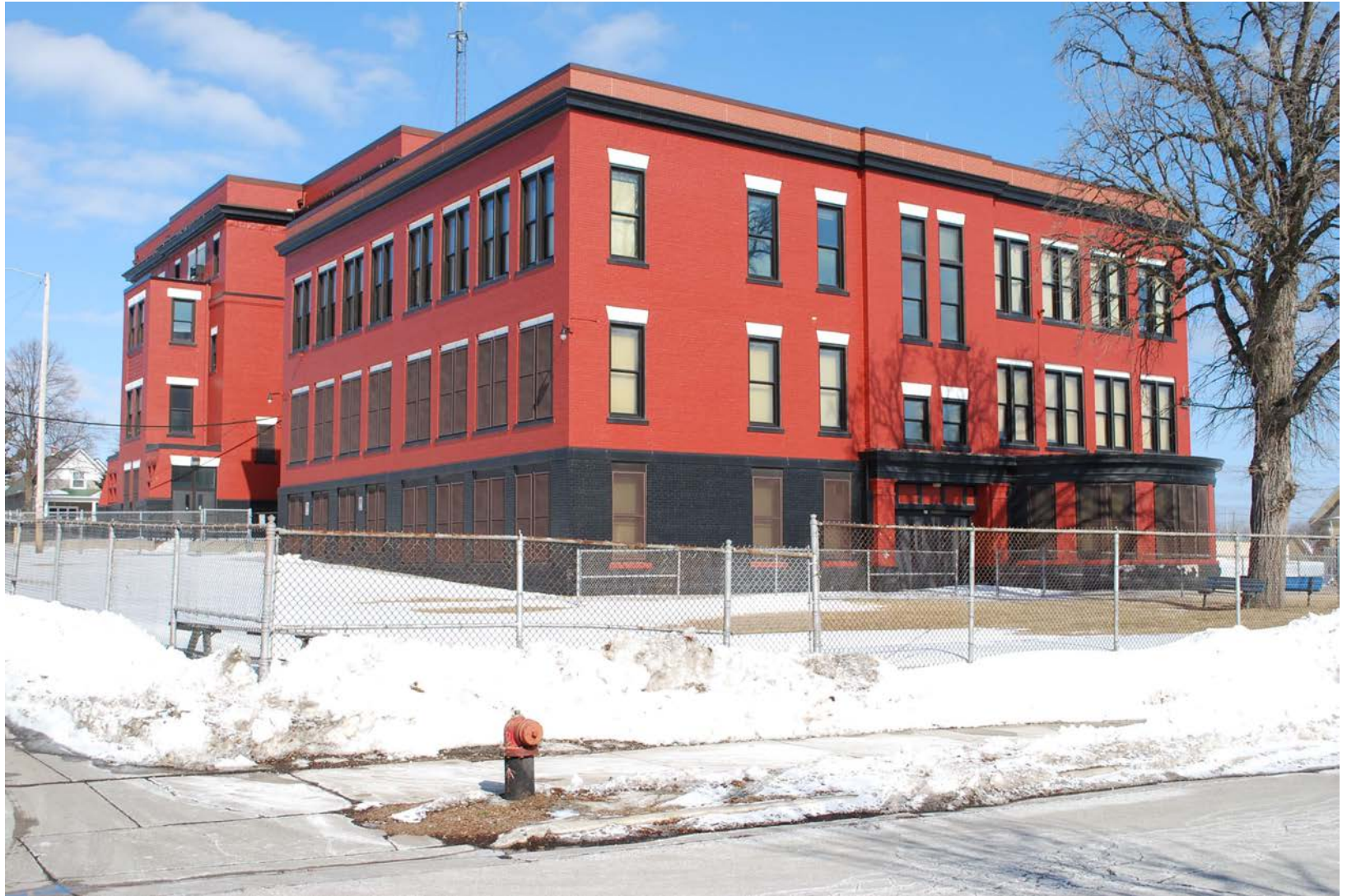
Dover Street School and Social Center, City of Milwaukee, Milwaukee County, 3 of 14
