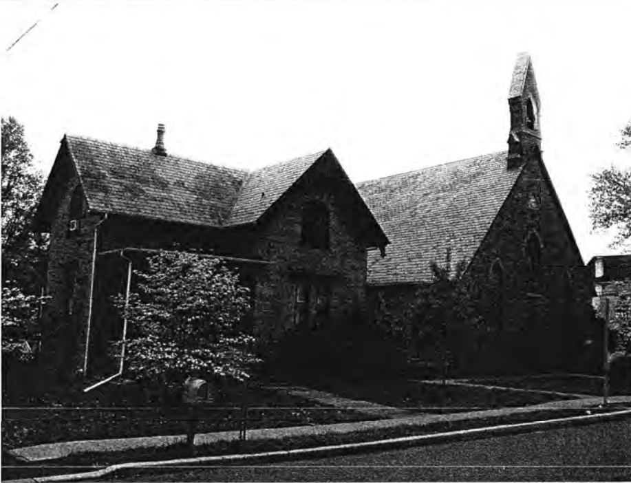
James Bird, Architect, First Presbyterian Church of Stockton, Stockton, NJ, 1867.
