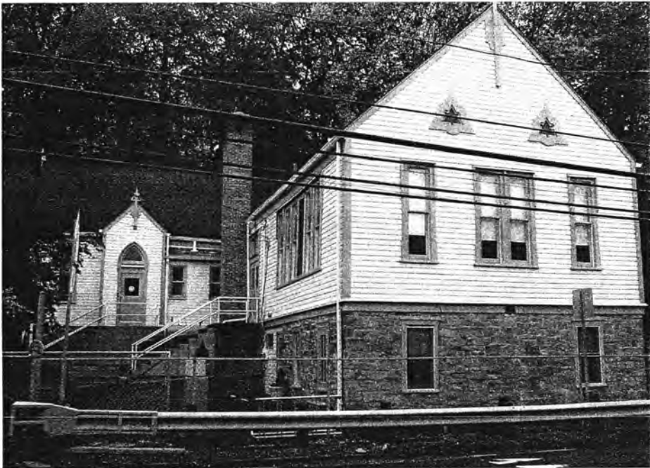
James Bird, Architect, District No. 98 Schoolhouse, Stockton, NJ, 1872-1884.
