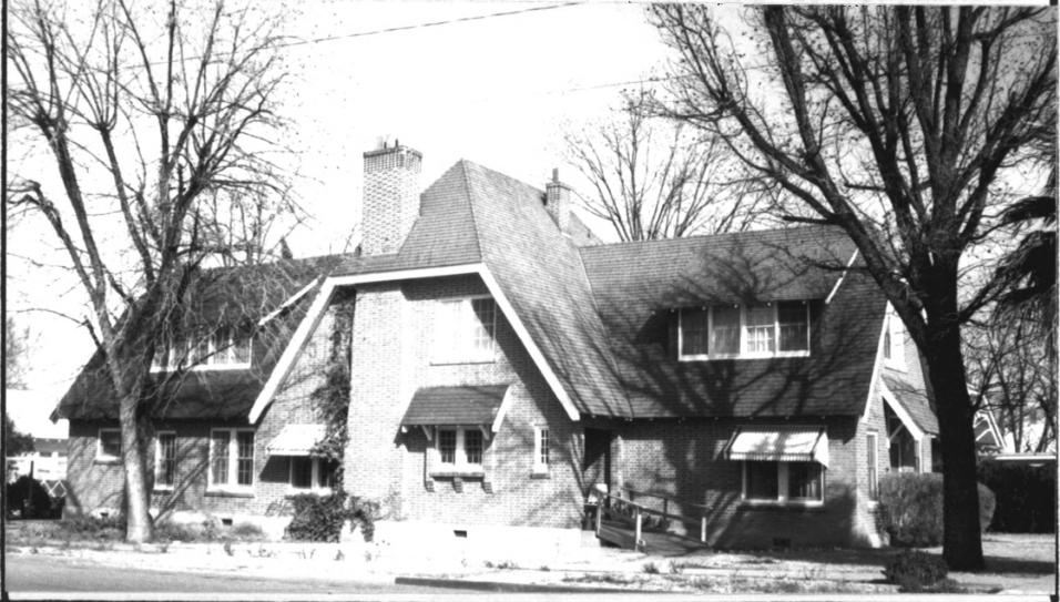
ADDITIONAL DESCRIPTION/ANALYSIS (annotated form): Roof type contd: hipped gable, shed roof dormers, brick chimneys. Porches contd: on 11th Street. Alteration contd: conversion to duplex, wheel chair ramp on top of original stairs.
