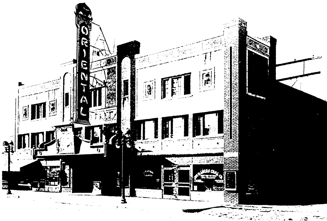
Figure 3. This circa September 1929 photograph of the Oriental Theater shows the south elevation, the original marquee, and part of the east elevation. SOURCE: Rocky Mountain Photo Company image in the files of the Denver Public Library, Western History and Genealogy Department; photo dated based on businesses in building and film being shown.
