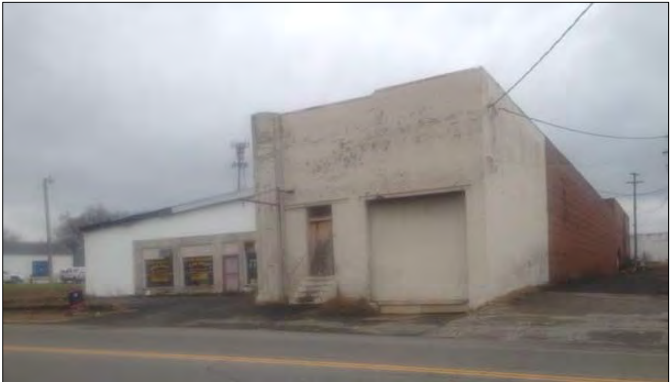
Figure 11: William M. McMurry Loose Floor Tobacco warehouse, 2016.
