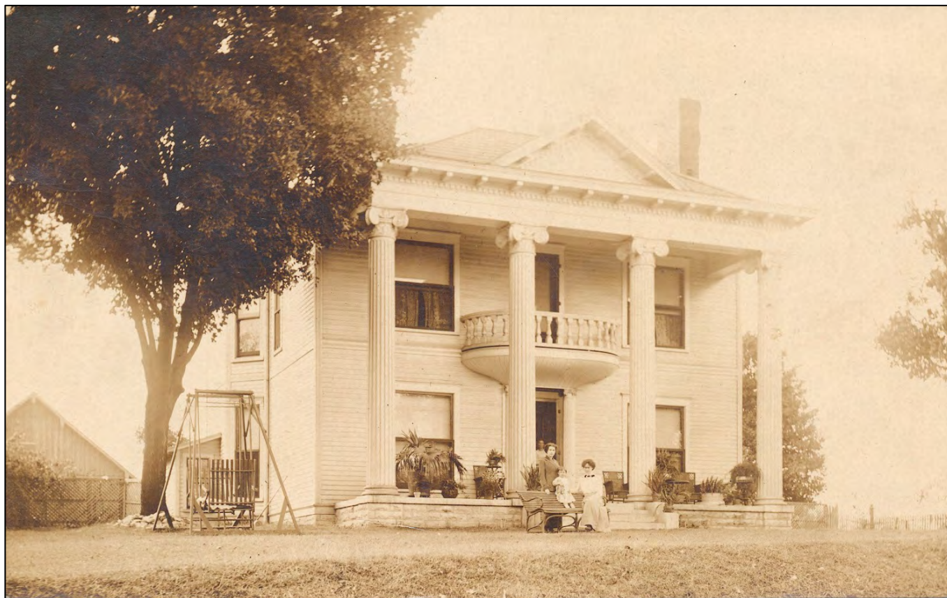
Figure 9: William M. Murry House, circa 1911. Source: Postcard of Sandra Helm Workman, descendant of Lizzie McMurry.
