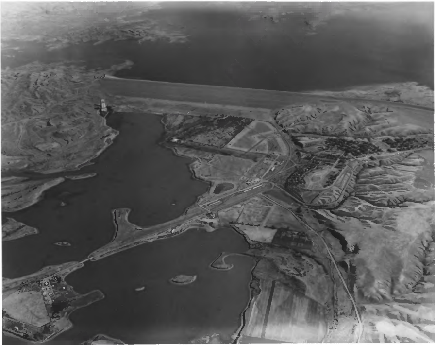
Fort Peck Dam, Fort Peck area, MT
