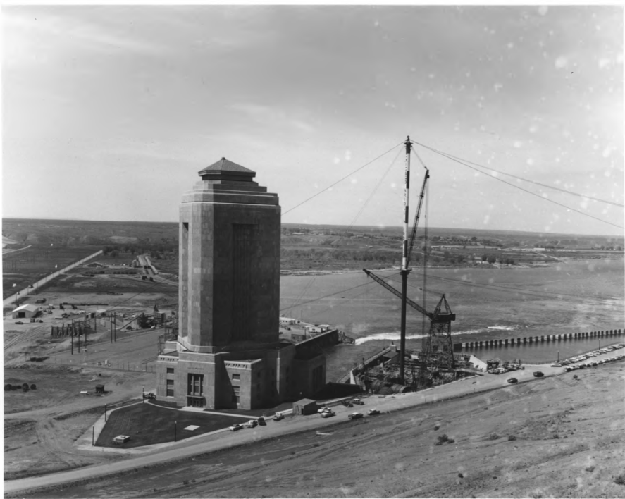
Fort Peck Dam, Fort Peck M.H.A., MT
