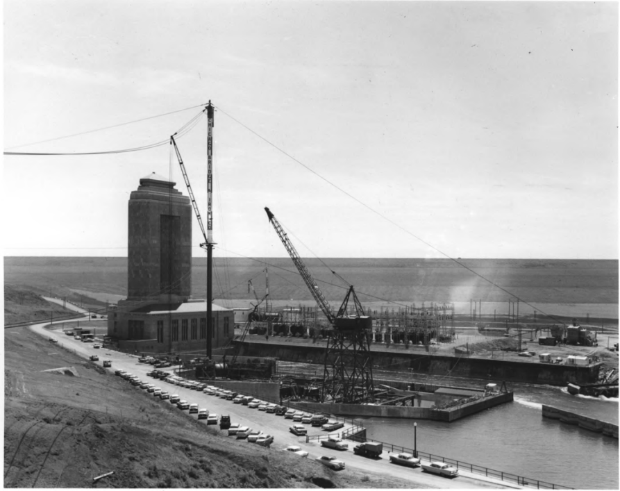
Fort Peck Dam, Fort Peck, M.D., MT
