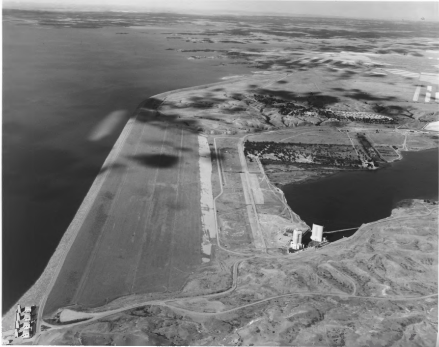
Fort Park Dam, Fort Park MRA, MT
