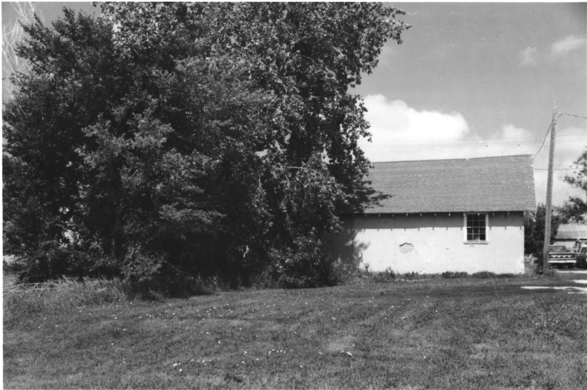
Experimental Rammed Earth Machine Shed, Brookings Co., S.D., No. 5
