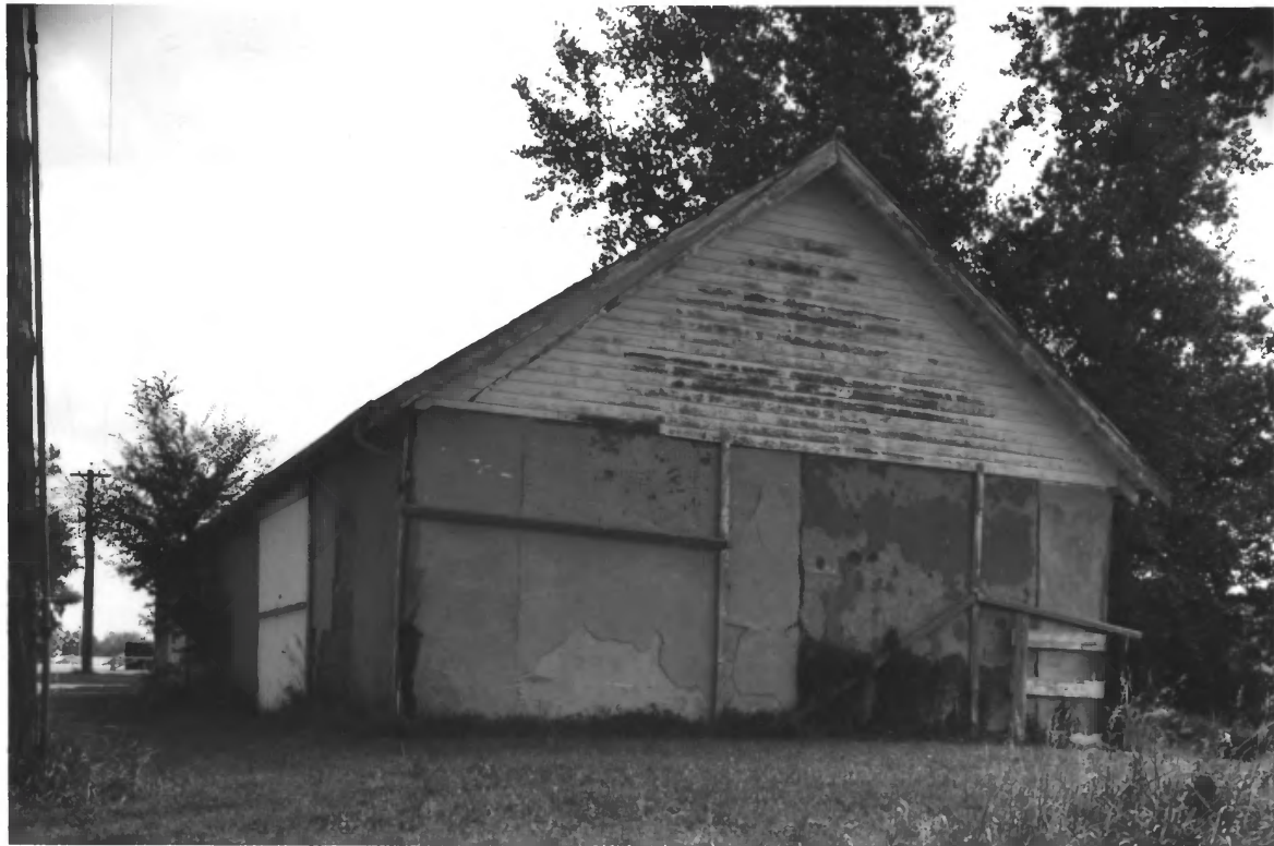
Experimental Rammed Earth Machine Shed, Brookings Co., S.D. , No. 3
