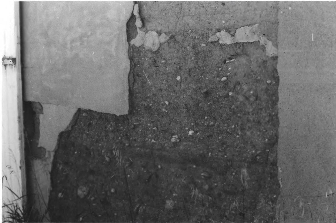
Experimental Rammed Earth Machine Shed, Brookings Co., S. D., No. 2
