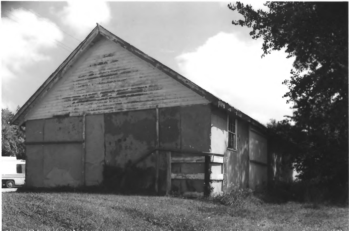
Experimental Rammed Earth Machine Shed, Brookings Co., S.-D., No. 4
