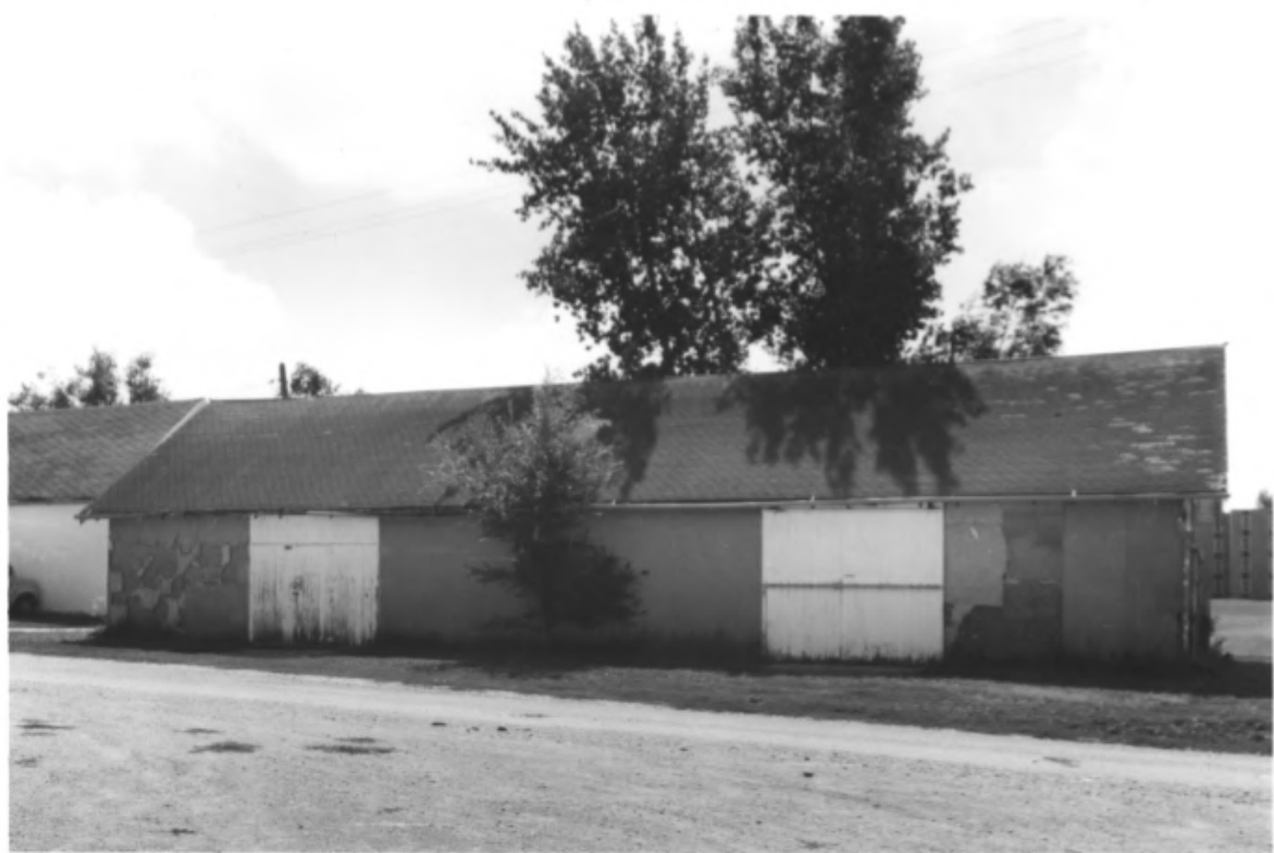
Experimental Rammed Earth Machine Shed, Brookings Co., S.D., No. 1
