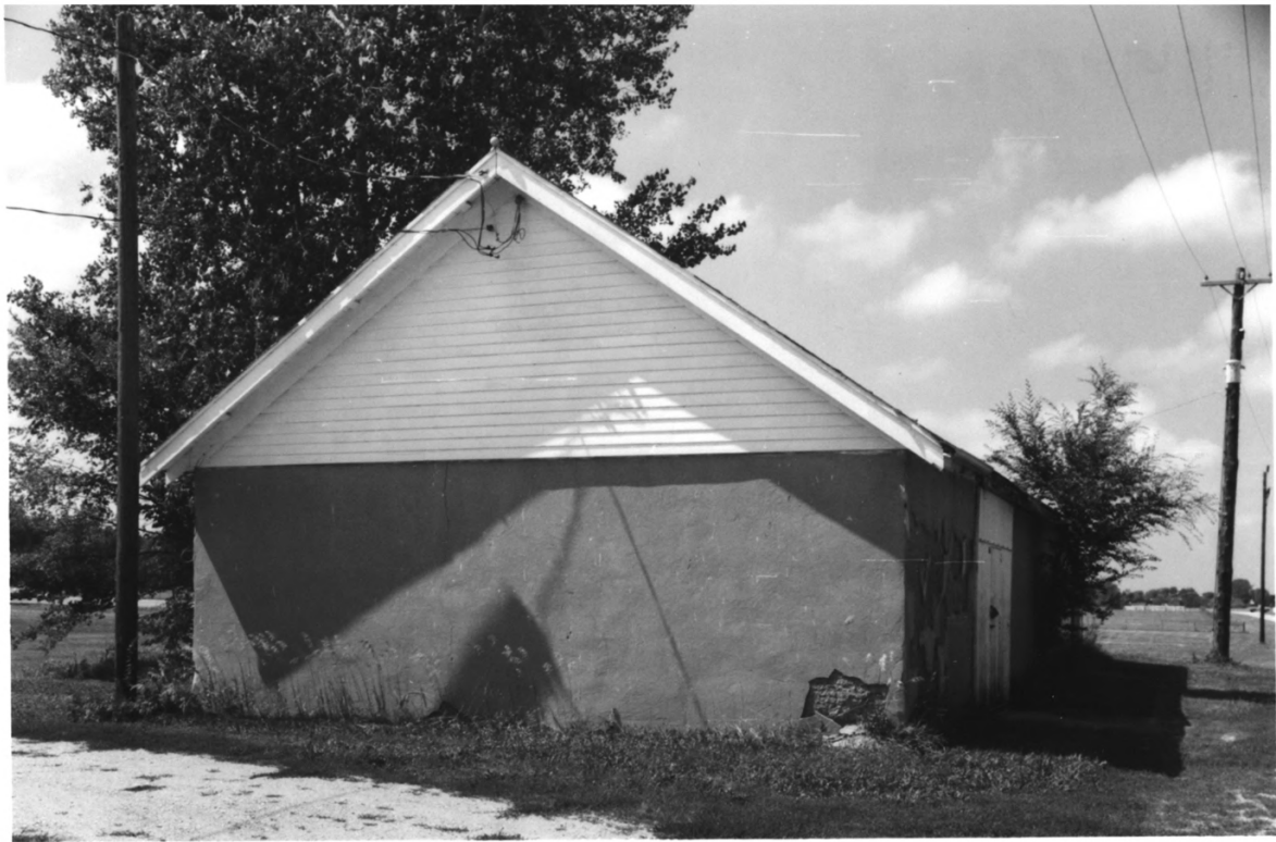
Experimental Rammed Earth Machine Shed, Brookings Co., S-D., No. 6
